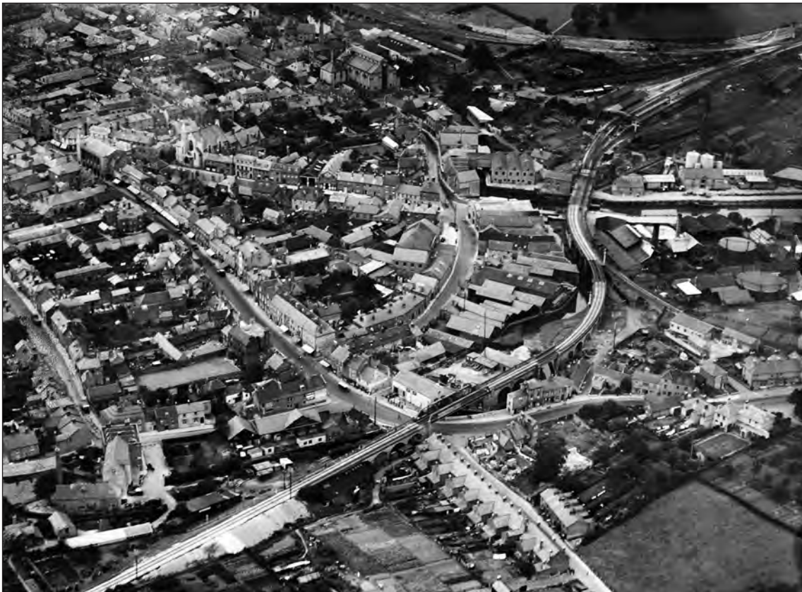
Figure 18 – The area of plan-unit I, seen from the south-east in 1928 (EPW023022, © Historic England Archive - Aerofilms collection).
