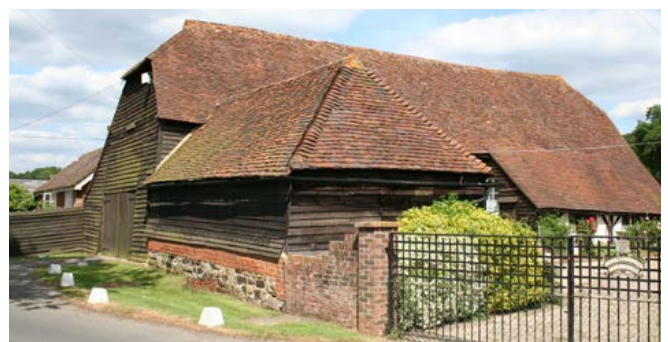
Barns in the Low Weald rarely exceeded five bays in length. This example has a former shelter shed attached to its side and possibly stabling in the single-storey range. Photo © Bob Edwards
