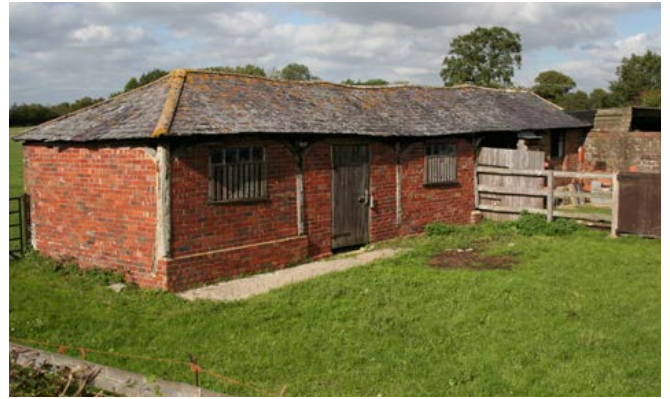
Most cattle housing in the area dates from the 19th century and took the form of open-fronted shelter sheds. This range has been subsequently infilled with brick to provide stabling. Photo © Bob Edwards
