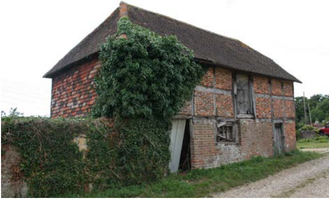
A rare example of a timber-framed stable, probably 17th century in date. The lower wall has been re-built in brick. Photo © Bob Edwards
