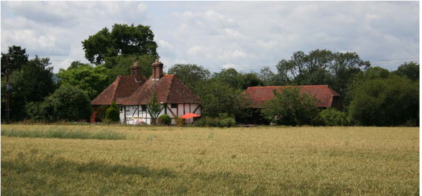
A characteristic small Wealden farmstead with its medieval, timber-framed house with a hipped roof and a barn clad in weatherboard, set within a landscape of medium-sized fields with well-wooded boundaries. Photo © Bob Edwards
