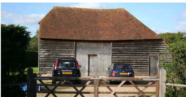
A three-bay barn with an outshot against the gable end. The small door suggests that this was a multifunctional barn, possibly providing stabling or housing for cattle in this end of the building. Photo © Bob Edwards
