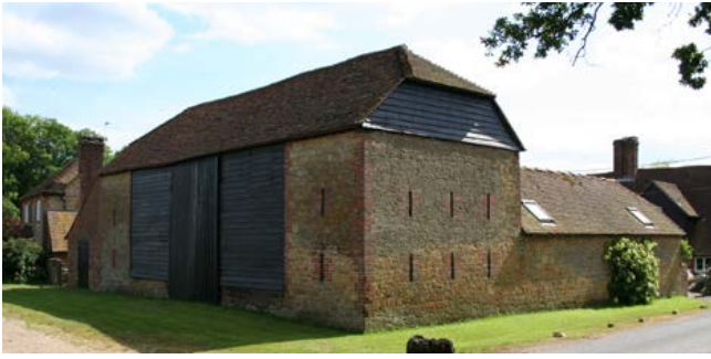
A regular L-plan yard with a five-bay barn and attached single-storey range that provided stabling or housing for cattle. Photo © Bob Edwards
