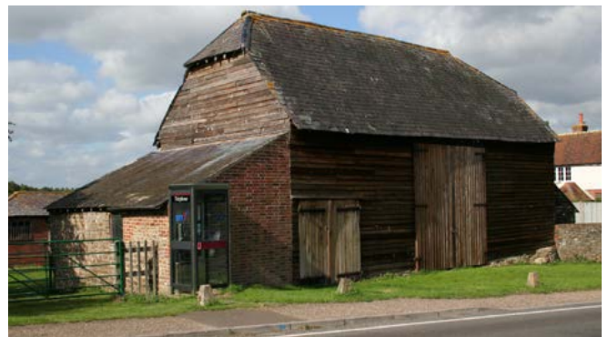
Timber-framed barns of three bays are common on the smaller farms of the area. Photo © Bob Edwards
