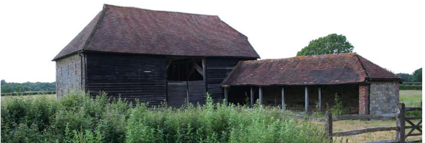
Outfarms and field barns were once a common feature of the Low Weald landscape but few survive intact. This outfarm has a three-bay barn and attached shelter shed facing into a yard. Photo © Bob Edwards
