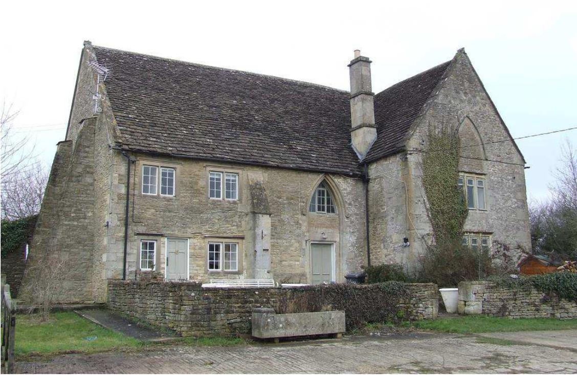
*Figure 3: General view of the south elevation of Manor Farmhouse. Hall range to the left and cross-wing to the right (photo Matt Hurford)*
