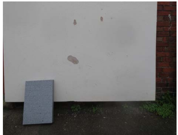
Figures 34 – 37 Several areas of failing render finish; reasons for this are unclear, possibly impact or unsuitable application
