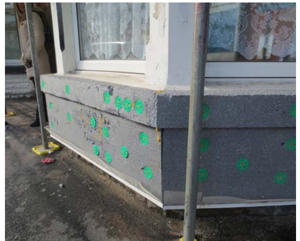
Figures 68 - 71 Different insulation treatments below bay windows: (clockwise from top left) (i) Conventional flashing; (ii) No flashing, graded insulation, sill uninsulated; (iii) No flashing, insulated to top of sill; (iv) No insulation, render only
