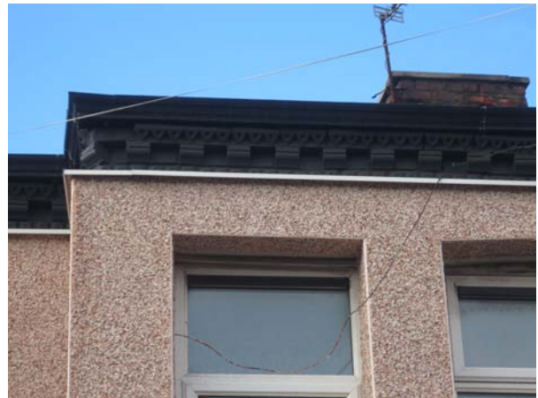
Figures 54 – 55 The ornate brickwork at eaves has been left exposed
