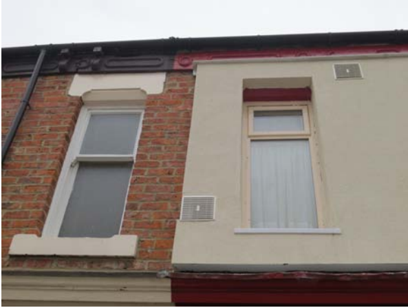
Figure 16 Untreated vs treated window, Note new sill
