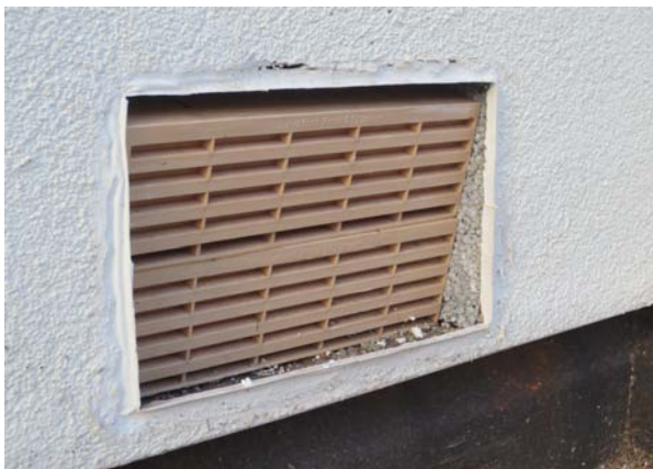
Figures 90 - 91 Possible routes for rainwater ingress behind insulation
