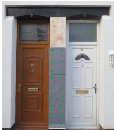
Figures 88 & 89 Uninsulated vs insulated party wall frontage; the difference in thermal impact is unclear
