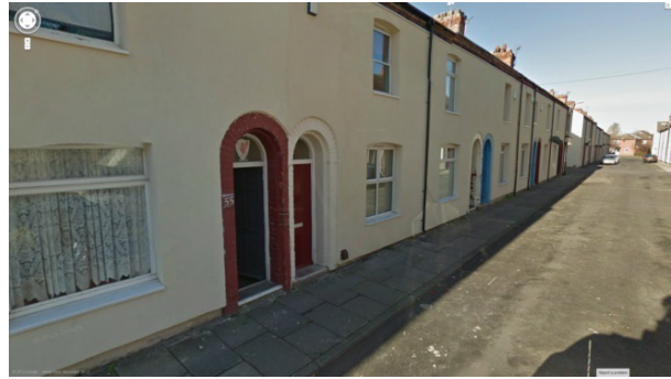
Figures 38 & 39 Untreated door surrounds; note different detailing on opposite sides of street 54
