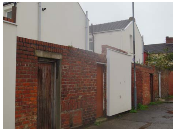
Figure 31 Insulation to end wall
