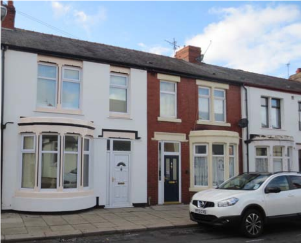
Figures 74 & 75 Note different approaches to lintels, i.e. leaving exposed or covering: leaving them exposed retains the feature but increases the thermal bridge, covering them creates a cleaner look and increases insulation coverage
