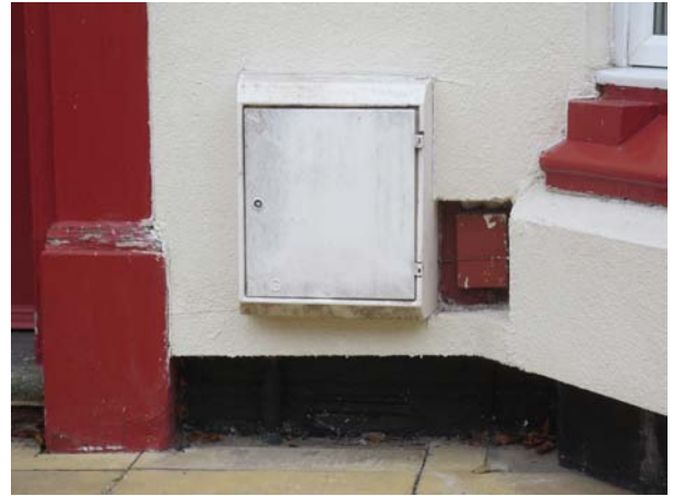
Figures 10 & 11 Thermal bridges at eaves, lintel, flue, gas box and floor level
