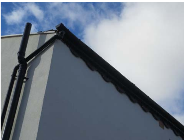
Figures 72 & 73 Insulated to top of eaves (left) and stopping short due to lack of space (right)
