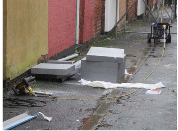
Figure 27 Wet EPS boards awaiting installation
