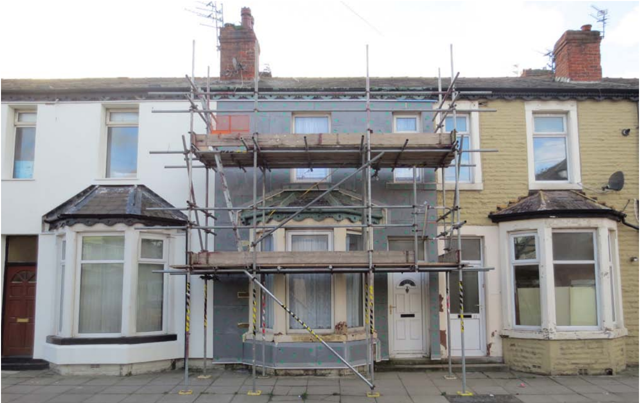
Figure 65 Three identical properties at different stages: completed, underway and untreated
