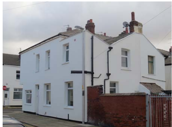
Figure 85 Lamppost obstructing pipework removal
