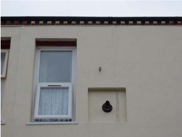
Figures 10 & 11 Thermal bridges at eaves, lintel, flue, gas box and floor level
