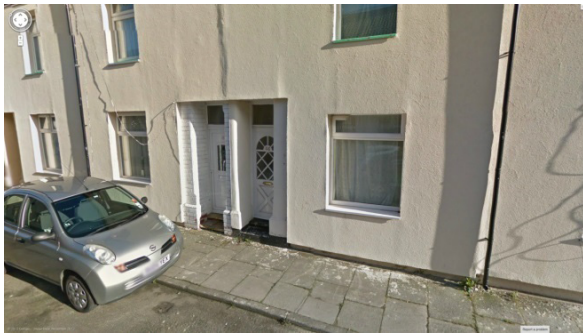
Figures 38 & 39 Untreated door surrounds; note different detailing on opposite sides of street 54
