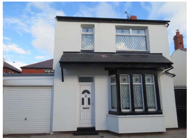
Figures 80 – 83 Note large uninsulated areas: vannels, gas pipes, porch roofs, window & door surrounds
