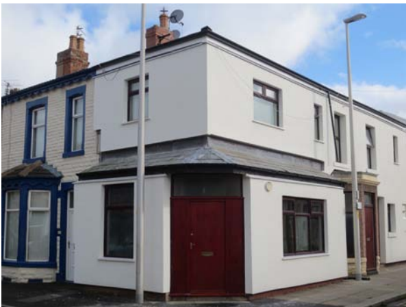
Figures 80 – 83 Note large uninsulated areas: vannels, gas pipes, porch roofs, window & door surrounds
