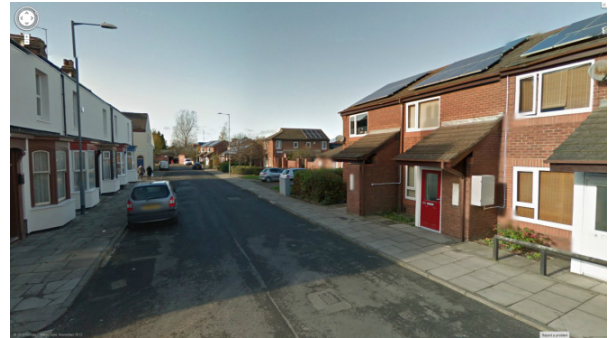
Figures 40 & 41 Alternative CO 2 - saving measures adopted on adjacent (more modern) properties (EWI vs PV) 55
