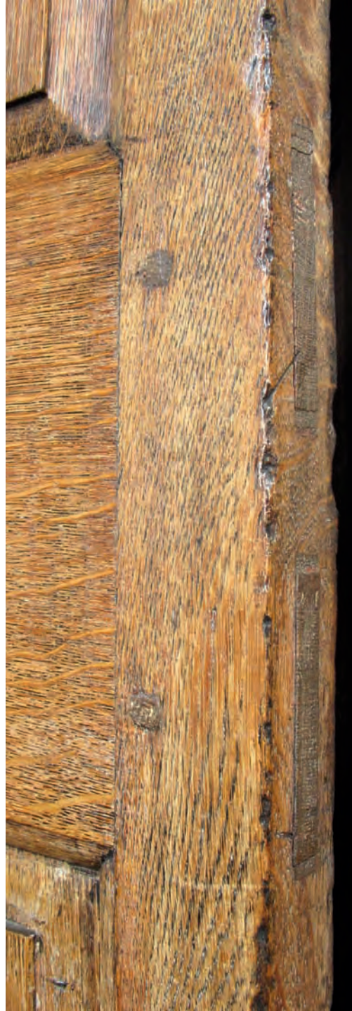
Pinned mortice-and-tenon joint in a late 17th-century door leaf. This method for securing joints in architectural joinery remained in use up to the early 19th century.
