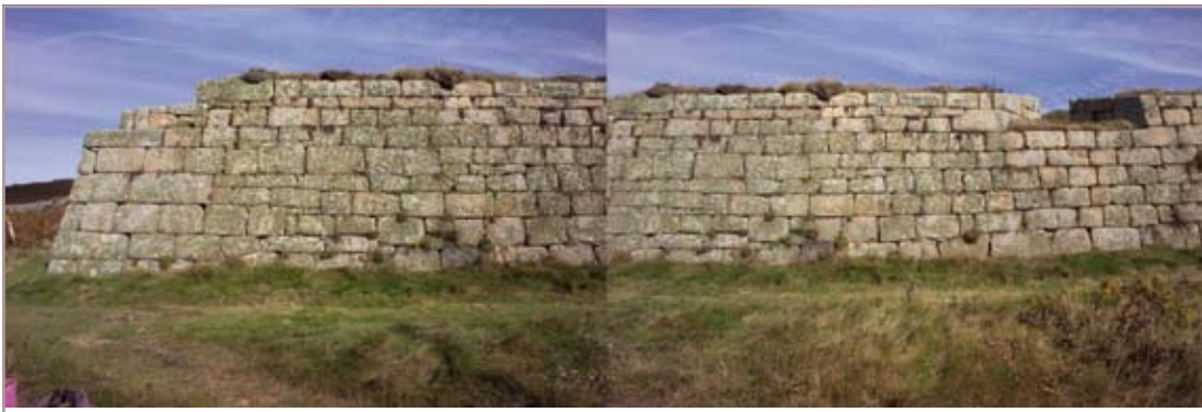
An outer face of a Redan, a part of the Garrison Wall. Above is, one pair of, a number of overlapping photographs taken by Mick Clowes and used by Steve Tovey, both of the Metric Survey Team, to produce the precise drawing of this face shown below
