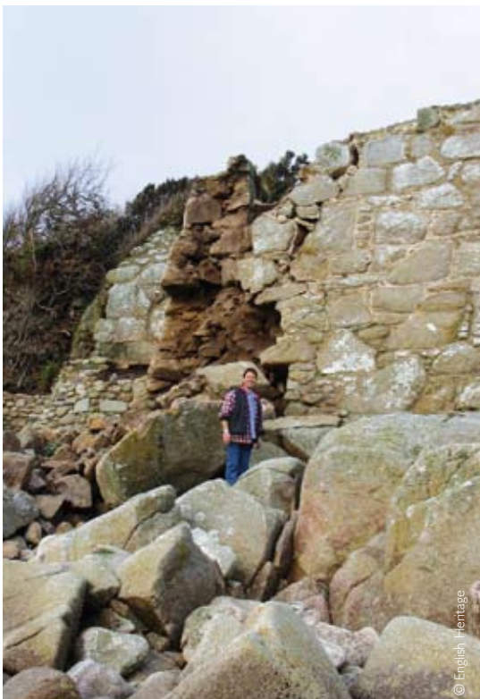
In 2004 part of a mid 18th-century gun battery that collapsed after a winter storm
