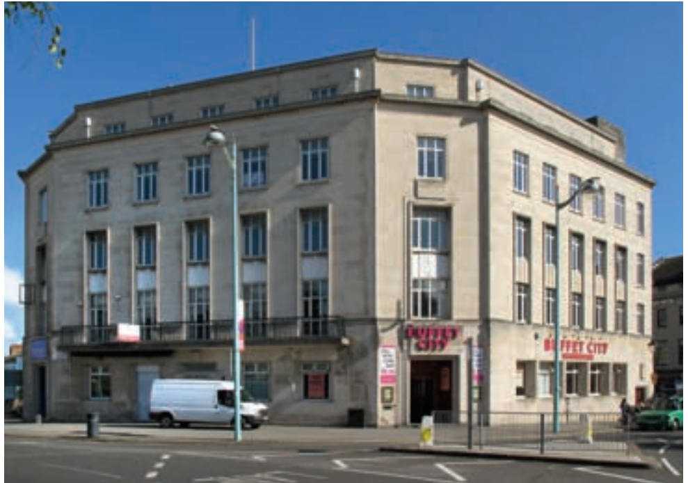
Figure 14 Royal Insurance (now Royal Building), St Andrew's Cross. Alec F French & Partners in association with Sir John Burnet Tait & Partners, 1949–53. [DP086667]
