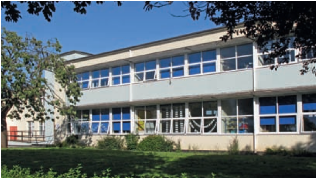
Figure 61 Plymview Primary School, Blandford Road, Efford. Edgar Catchpole, city architect, 1949. [DP088599]
