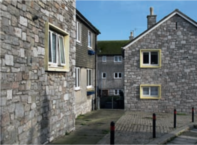
Figure 54 Housing at Paton Watson Quadrate, Barbican. H J W Stirling, city architect, 1958. [DP086735_1]
