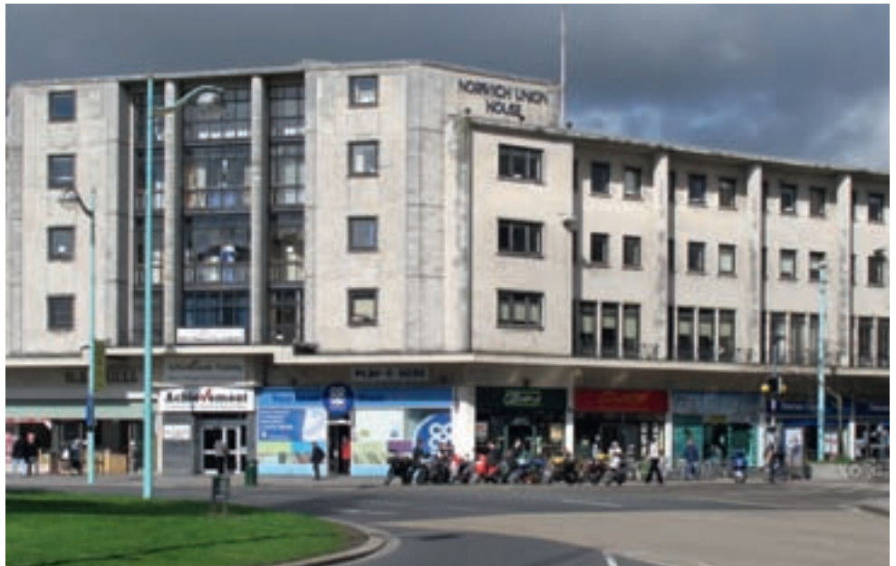
Figure 15 Norwich Union House, St Andrew's Cross/ Old Town Street. Donald Hamilton Wakeford & Partners, 1950–2. [DP086552]
