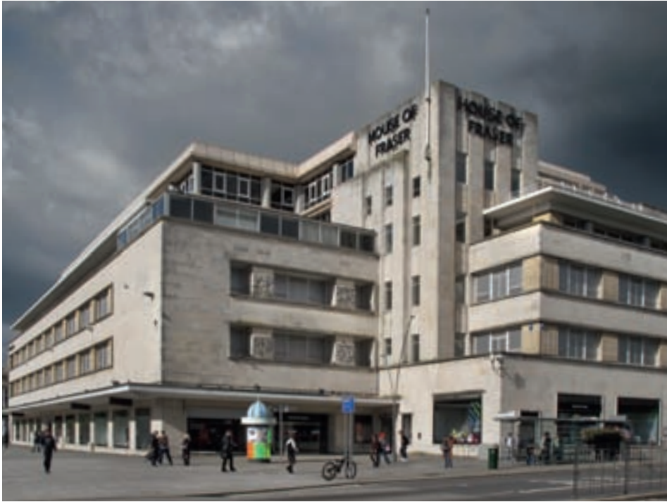
Figure 12 Dingles department store (now House of Fraser), Royal Parade. Thomas Tait of Sir John Burnet Tait & Partners, 1949–51. [DP086630]
