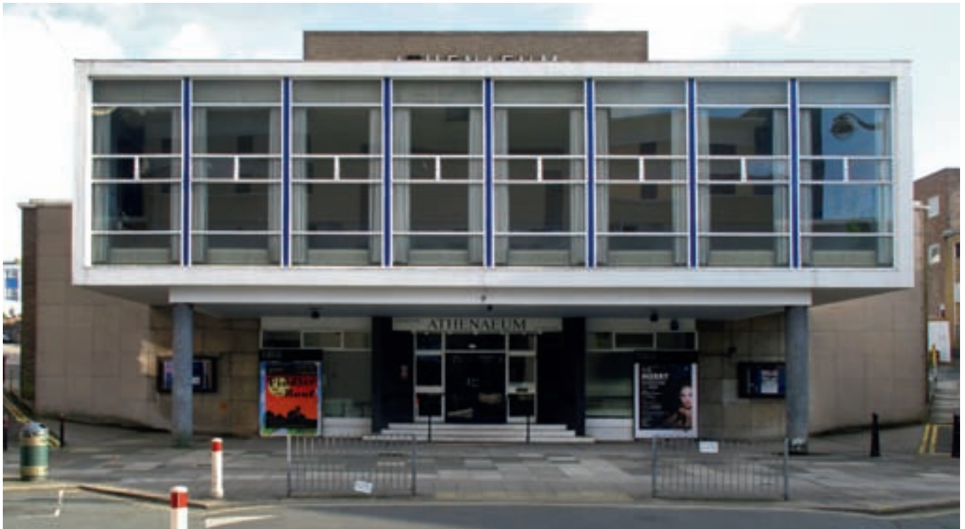
Figure 37 Athenaeum, Derry’s Cross. The symmetrical north elevation facing Derry’s Cross and axial to Raleigh Street. Walls & Pearn, 1958–61 [DP086703]
