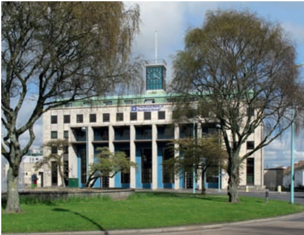
Figure 29 National Provincial Bank (now RBS), St Andrew's Cross. B C Sherren, staff architect to National Provincial Bank, 1955–8. [DP086531]
