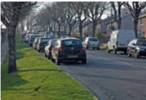
Figure 82 Blandford Road, Efford. BISF Type A houses on right, c 1949.
