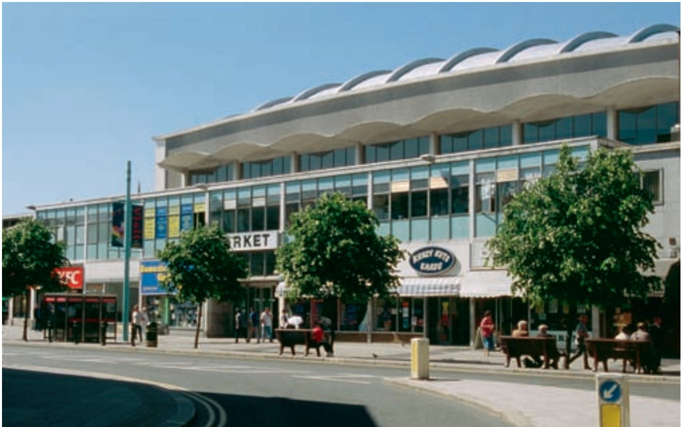
Figure 34 Pannier Market, New George Street/ Frankfort Gate/Cornwall Street (altered c 1999). Walls & Pearn, 1956–9.
