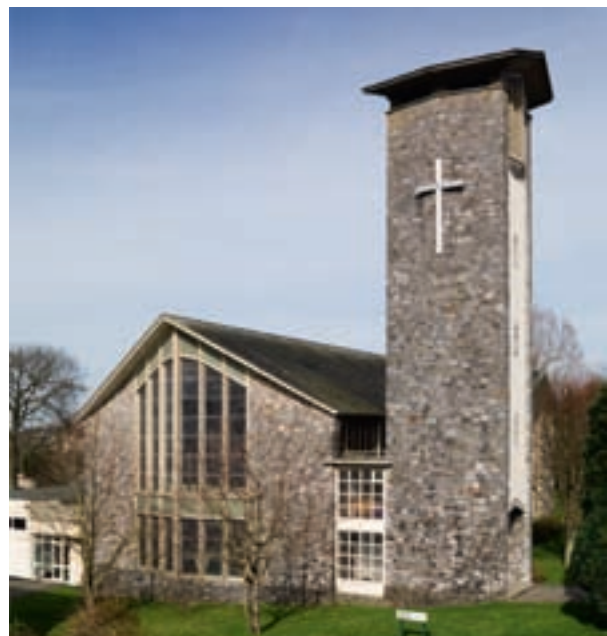
Figure 85 Church of the Ascension, Crownhill. The church from the south-west showing the separate campanile. Listed Grade II in 1998. Potter & Hare, 1956–8. [DP082231]
