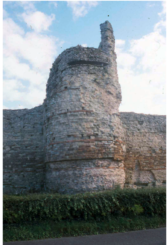
Figure 8 Bastion of the Saxon Shore fort of Pevensey. The upper part of the tower is a concealed Second World War pillbox. Note the slit for a machine gun.
