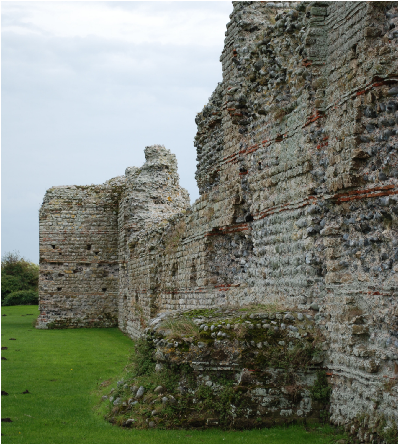
Figure 10 Wall and bastions on the north side of the Saxon Shore fort at Richborough.
