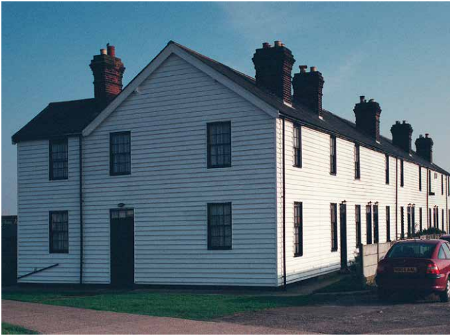
Figure 15 2-8 Haven Road, Canvey Island, Essex is a relatively rare example of a timber framed and weatherboarded row of Coastguard cottages. Dating from the late 19th century, the buildings are listed Grade II. © Joanna Smith
