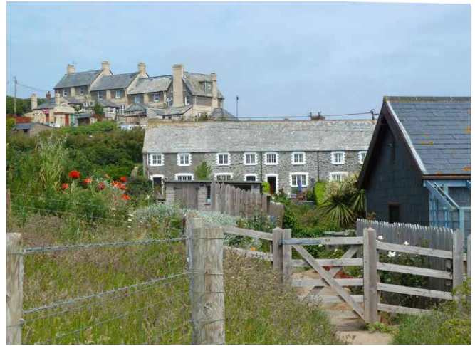
Figure 16 An impressive sequence of associated coastal buildings at Hawker's Cove, Padstow, Cornwall. A lifeboat station and a terrace of Pilots' cottages, dating from the mid-to-late 19th century, were joined by a row of turn-of-the-20th-century Coastguard cottages. The latter is built to the same design as the Isle of Grain station, indicating a more standardised design approach by the Admiralty.
