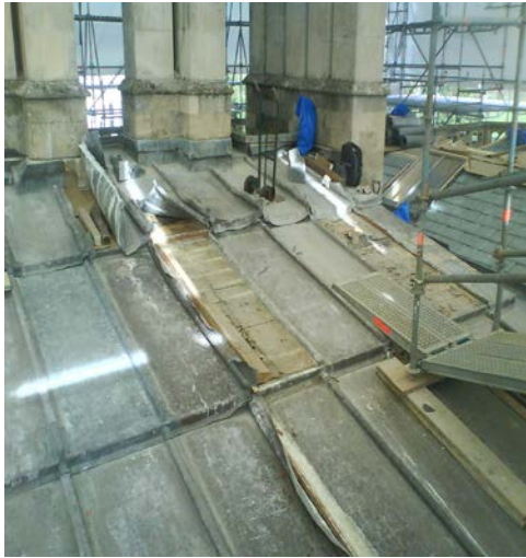
Works in progress to repair the historic leadwork on the South Wing
