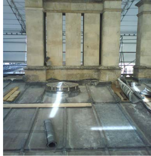
Works in progress to repair the historic leadwork on the South Wing
