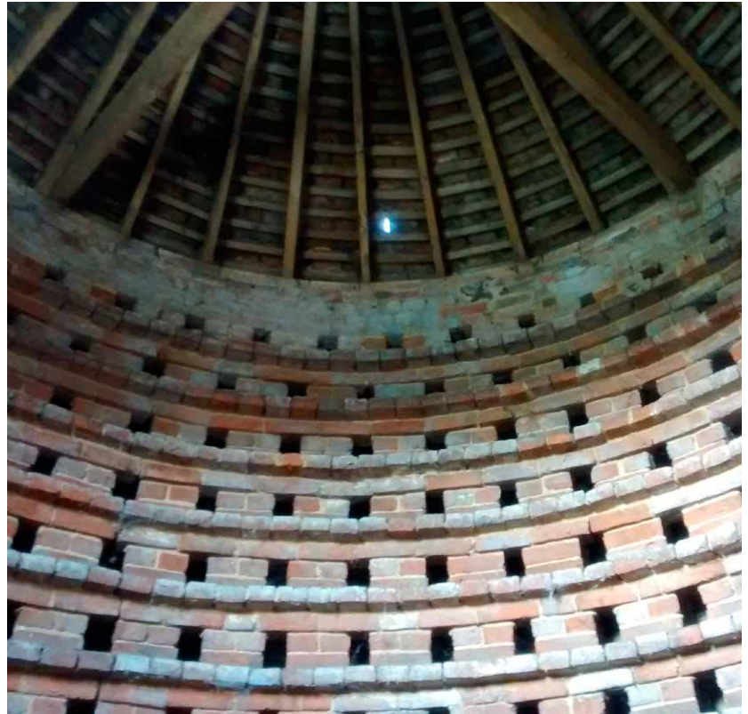
Right: Interior of listed dovecote near Donington showing brick nest-boxes. (The Fens)
