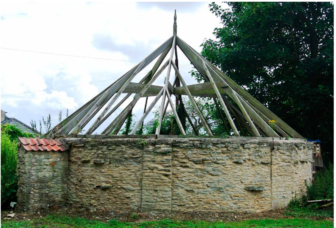
Horse Gin, Brauncewell. The roof was likely thatched rather than tiled. (Southern Lincolnshire Edge)
