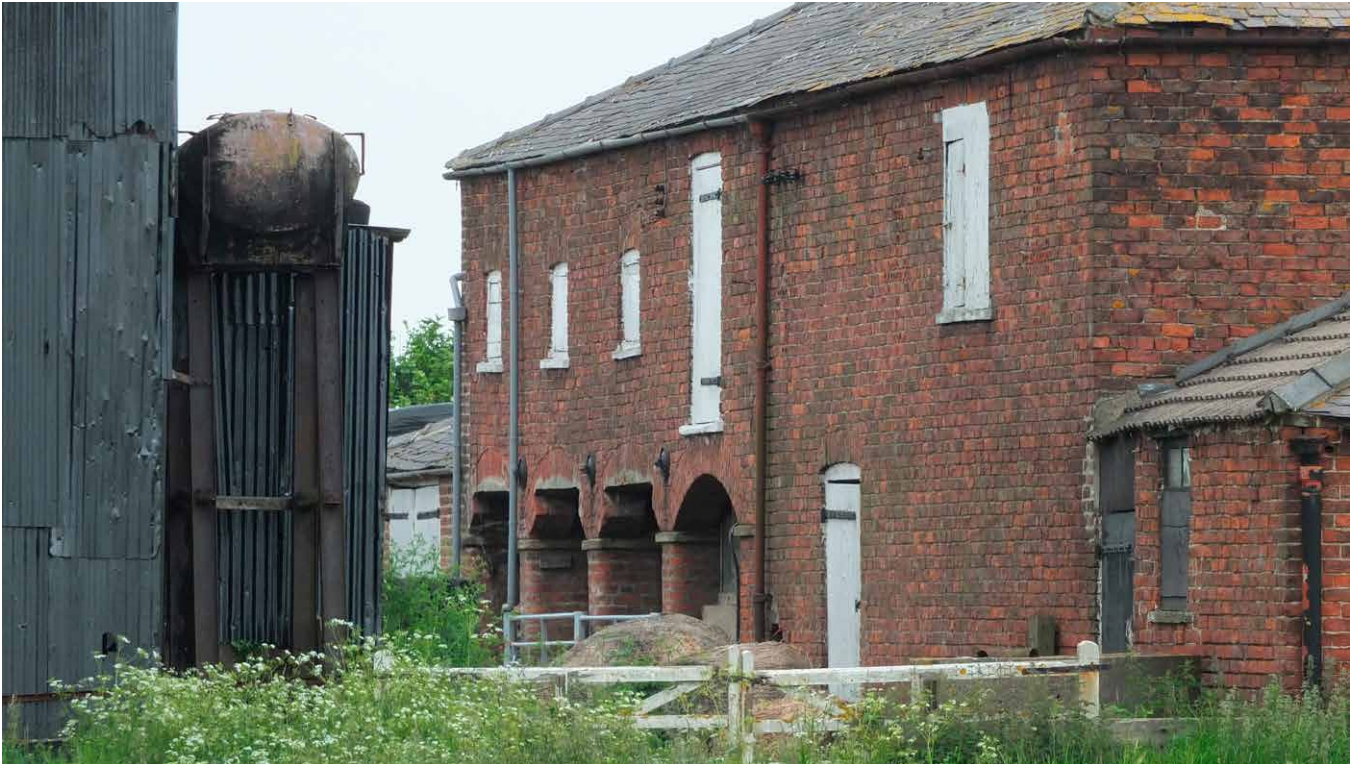
Granary raised over a four-bay cart shed. (Humberhead Levels) © Jen Deadman)
