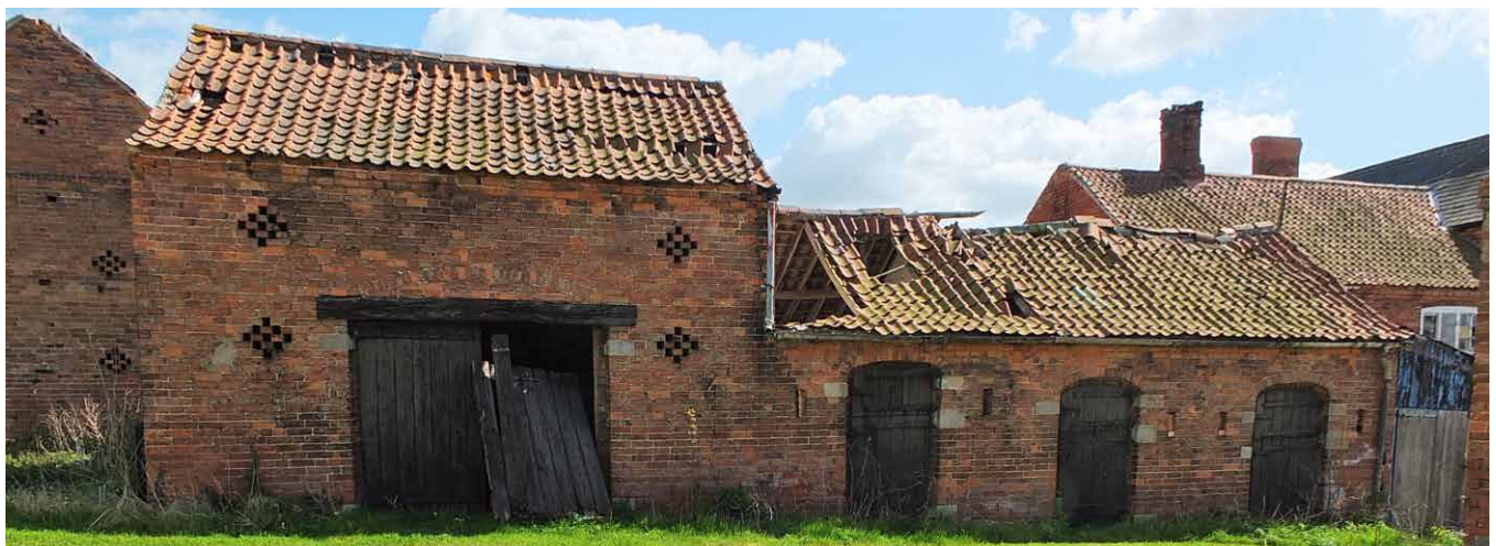
Top Left: Disused iron framed Dutch barn. (Kesteven Uplands)
