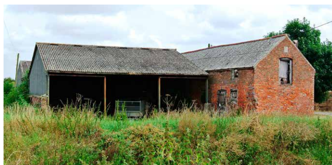
Outfarm with stacking yard and two cart shed extensions off a main brick threshing barn. (The Fens)
