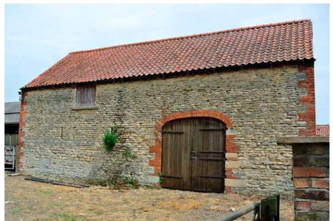
Bottom: Limestone barn with pantile roof and brick quoins and detailing. Saxby. (Northern Lincolnshire Edge)
