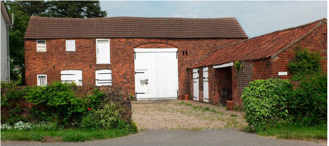
Combination barn, with an adjacent stable and granary in the same range. (Lincolnshire Coast and Marshes)
