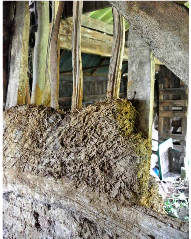
Top: Mud and stud wall construction. (Central Lincolnshire Vale)
