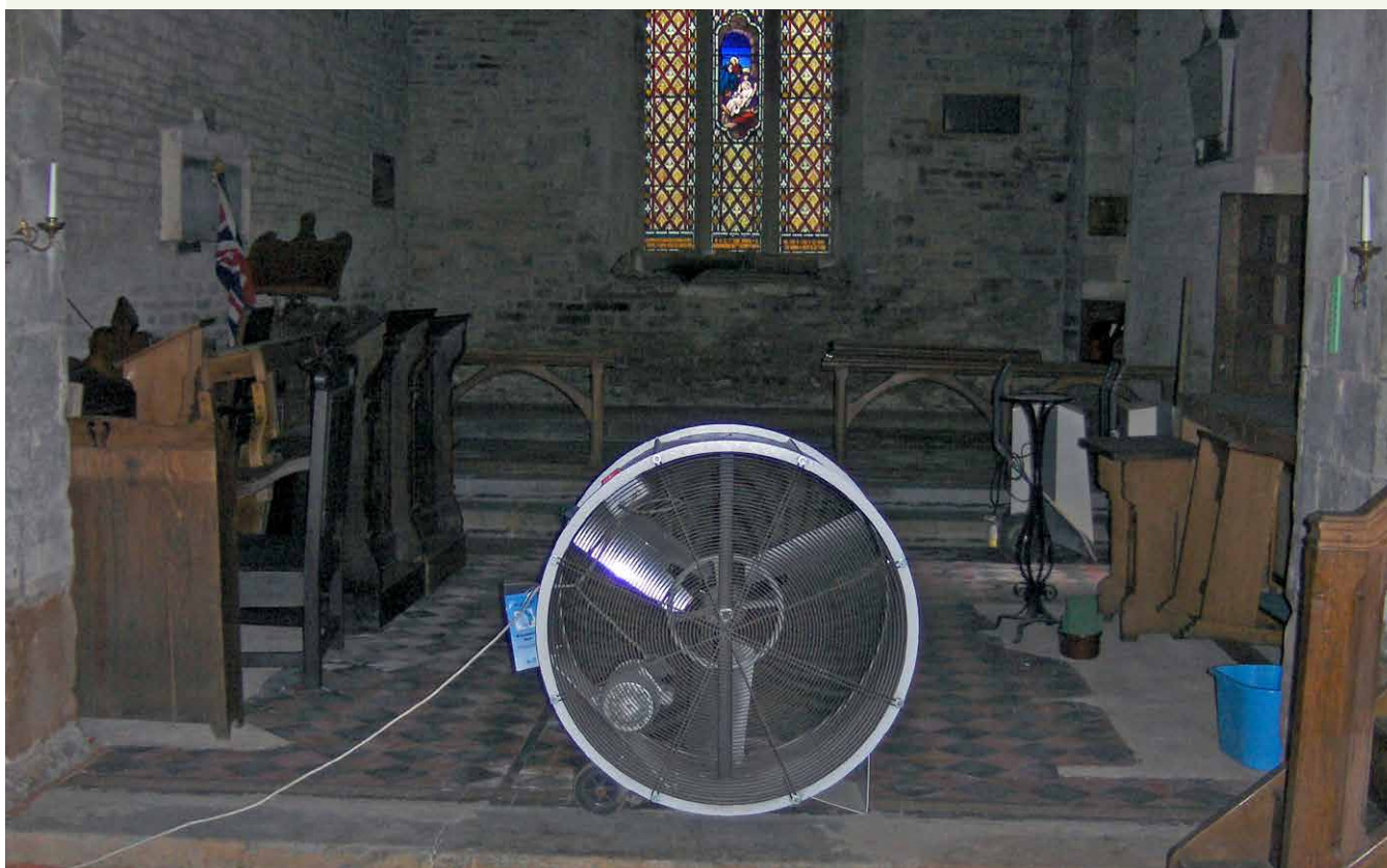
Large fans strategically placed to aid drying at Burford Church, Oxfordshire. [photo © Phil Hadley/Continuity]
