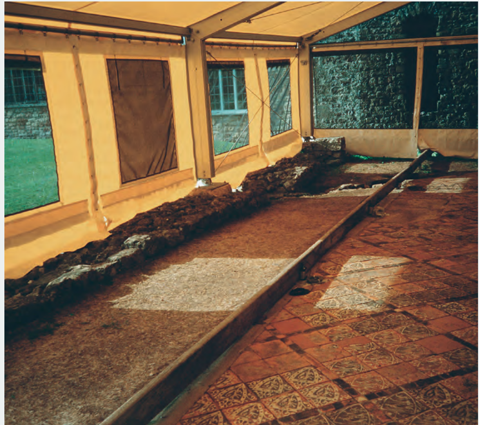
Solar radiation on the pavement contributes to environmental instability. These areas were specifically monitored to compare conditions with those constantly in shaded conditions.
