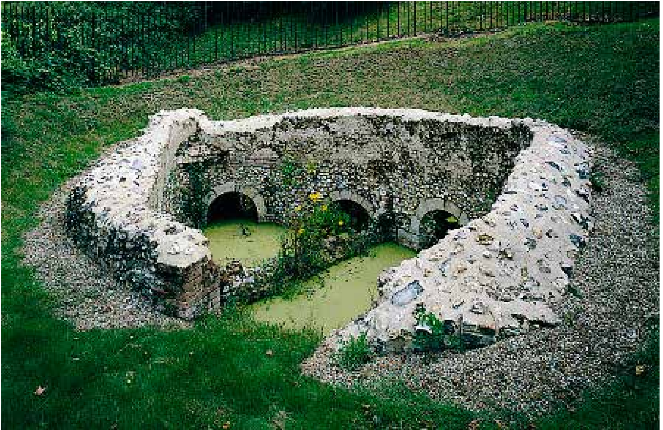
Figure 3 Conduit house, Canterbury, Kent. Part of the water supply for the Abbey of St Augustine, it comprises a mid-twelfth-century collecting and settling tank, now divided by an eighteenth-century wall. Four tunnelled
