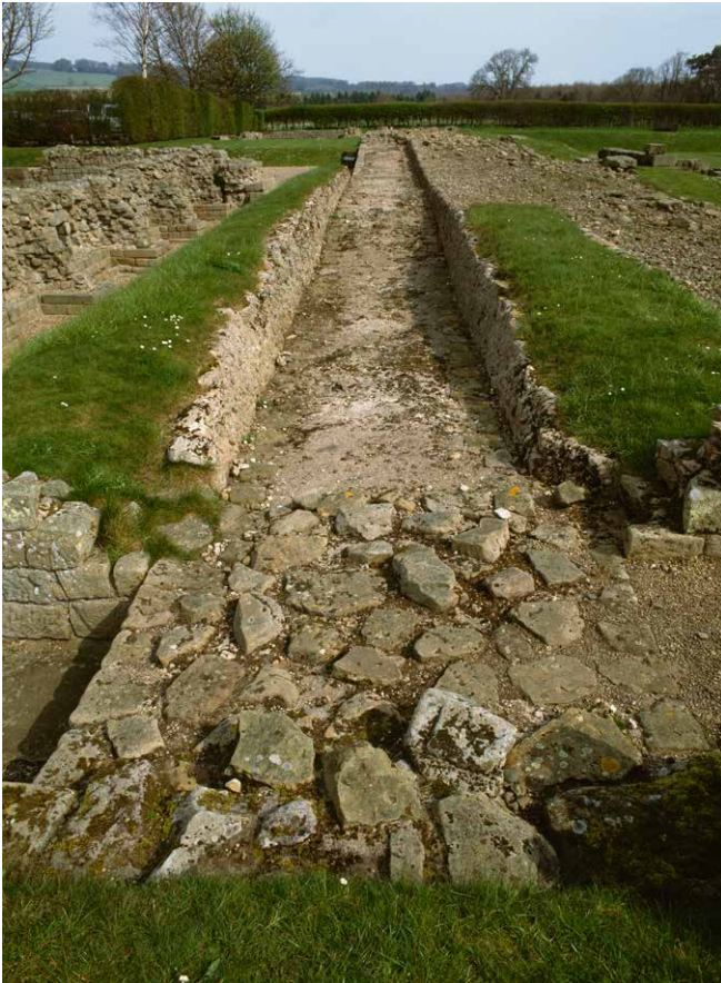
Figure 1 Roman aqueduct, Corbridge Roman town, Northumberland. An unusually well-preserved Roman aqueduct terminus, built by the XX Legion. It supplied water to a fountain house and water tank at the town centre.
