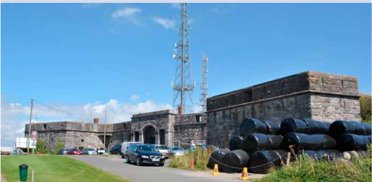
View of the entrance to Staddon Heights
