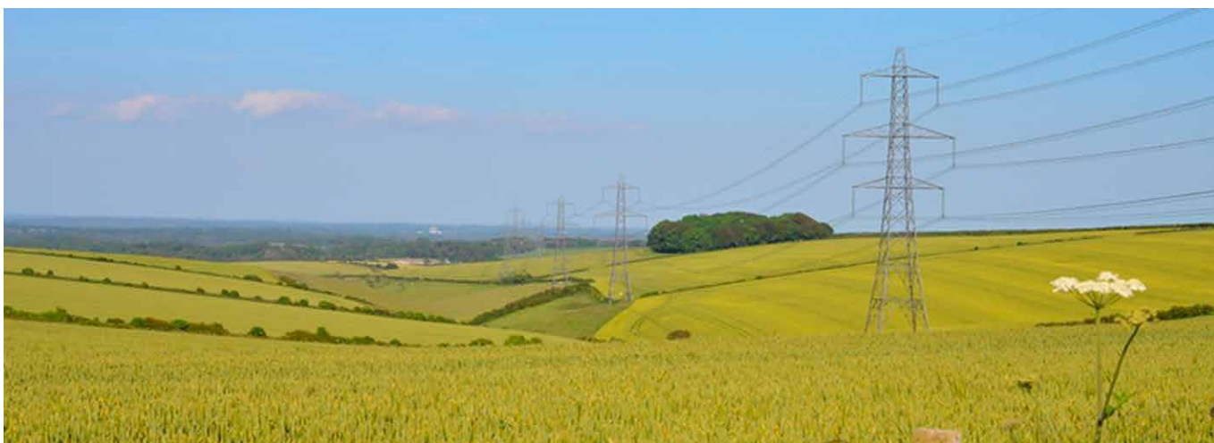
400kV line running through Dorset AONB. © National Grid plc
