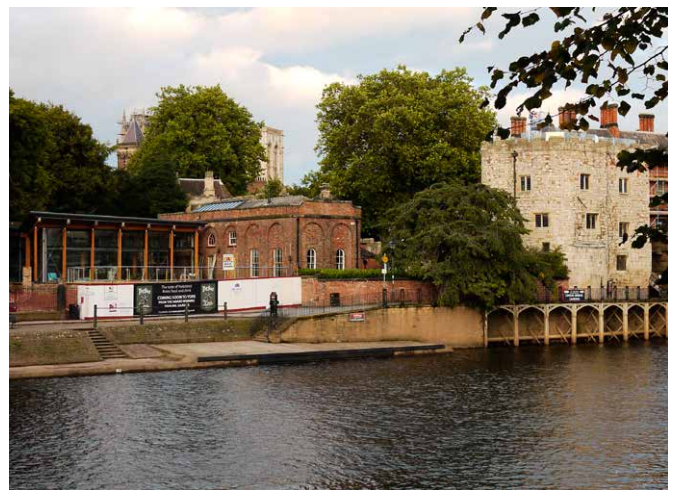
The Star Inn the City pub and restaurant. The new extension seen in its townscape context. © Historic England
