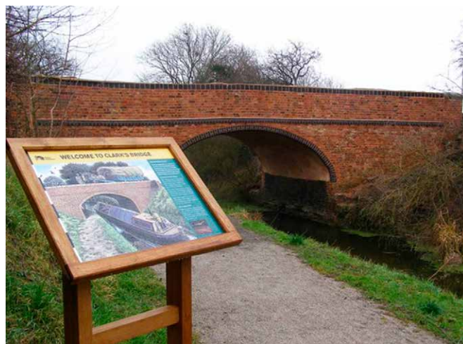
Works covered by the national LBCO will need to be of the highest quality. © Canal & River Trust
