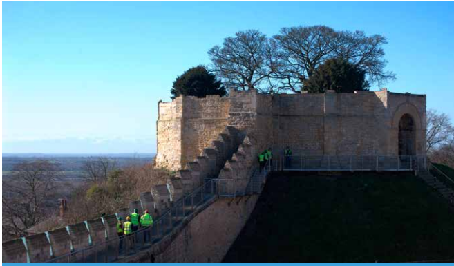
The shell keep on top of the Lucy Motte was comprehensively repaired as part of the Castle Revealed project and a full circuit to the wall walks was provided for the very first time vi a bridge on the exterior of the keep. © Andrew Tryner, Lincolnshire County Council
