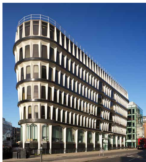
Front cover image: Former Credit Lyonnais building, 30 Cannon Street, London. © Historic England
