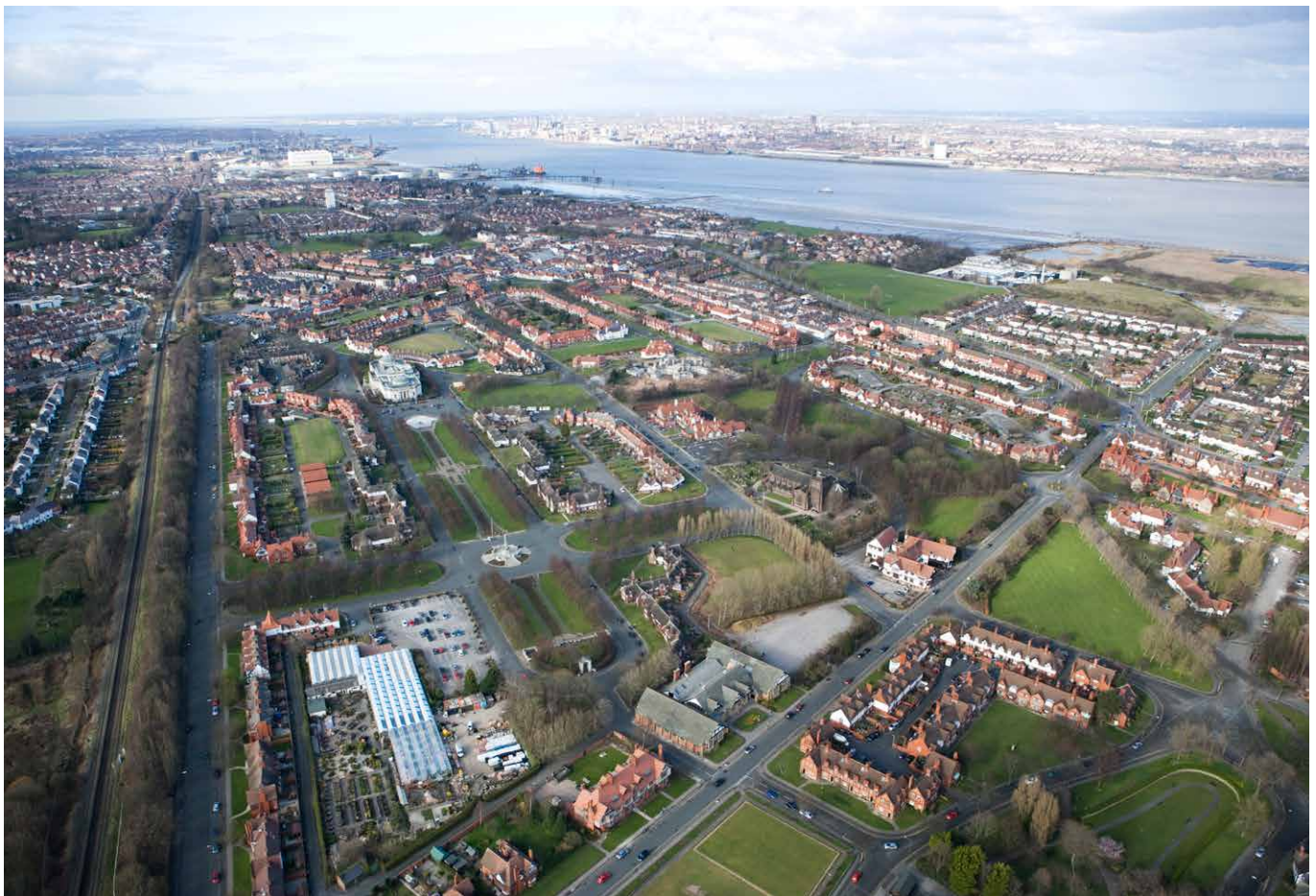
The principal part of the Model Village at Port Sunlight. © Historic England
