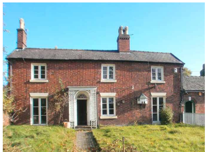
Repairs to a listed canal cottage could be covered by a Certificate of Lawfulness of Proposed Works. © Canal & River Trust
