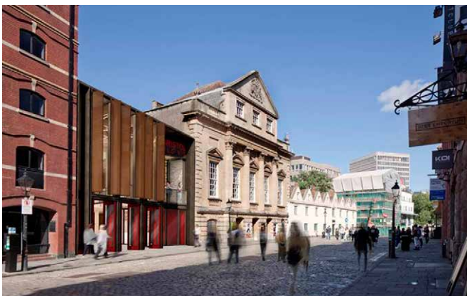
The Old Vic showing Moro’s blank studio elevation; The replacement structure, designed to create an active street frontage and obvious access point. © Haworth Tompkins and AVR London
