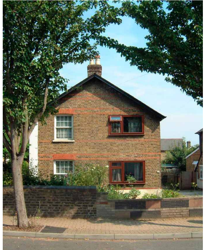
The Heritage at Risk campaign on conservation areas highlighted replacement windows as being the number one threat. © Historic England
