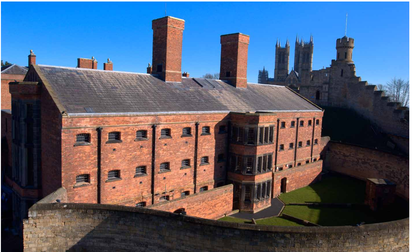
The Victorian prison building at Lincoln Castle, designed to enact the separating system which kept prisoners in near isolation removed from the corrupting influence of other inmates. The building has been comprehensively repaired and re-interpreted as part of the project. © Andrew Tryner, Lincolnshire County Council
