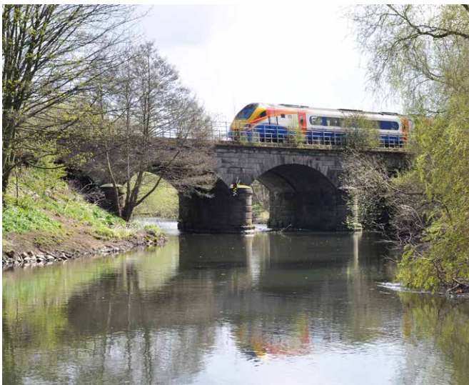
Derwent Bridge, Derby, on the Midland Main Line, now listed grade II. It was originally built as part of the North Midland Railway in 1836-40. © Alan Baxter and Associates
