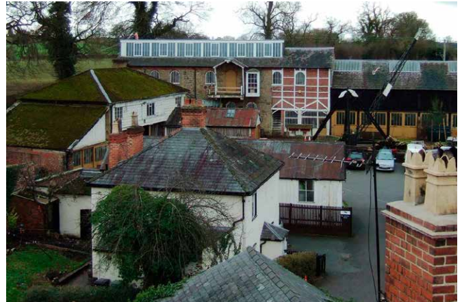
Ellesmere Yard could be subject to a Listed Building Heritage Partnership Agreement. © Canal & River Trust
