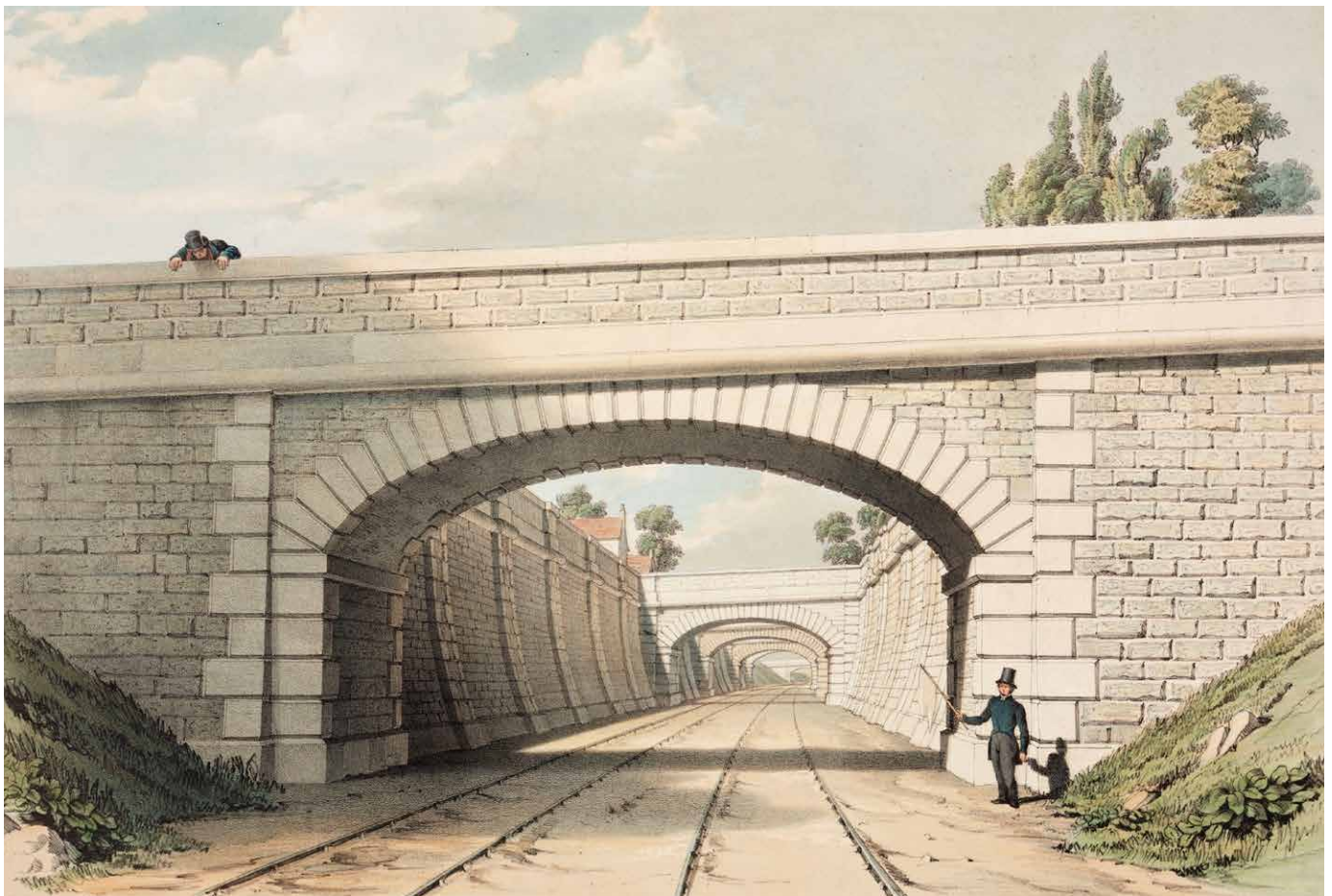
Lithograph by Samuel Russell c.1840 showing a sequence of bridges through Belper, Derbyshire, now part of the Midland Main Line. © Science Museum / Science & Society Picture Library
