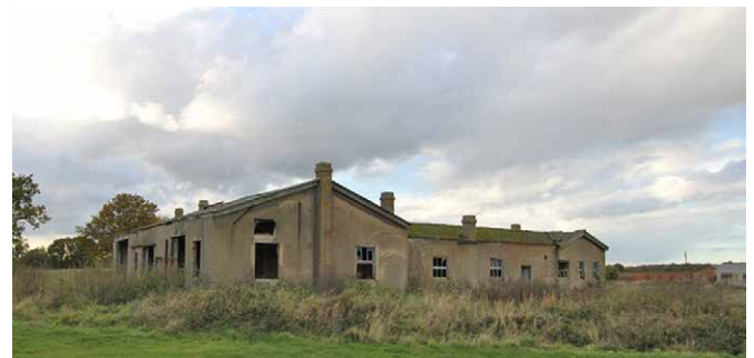
SMGWA: Building Hierarchy architectural features. © Maldon District Council
