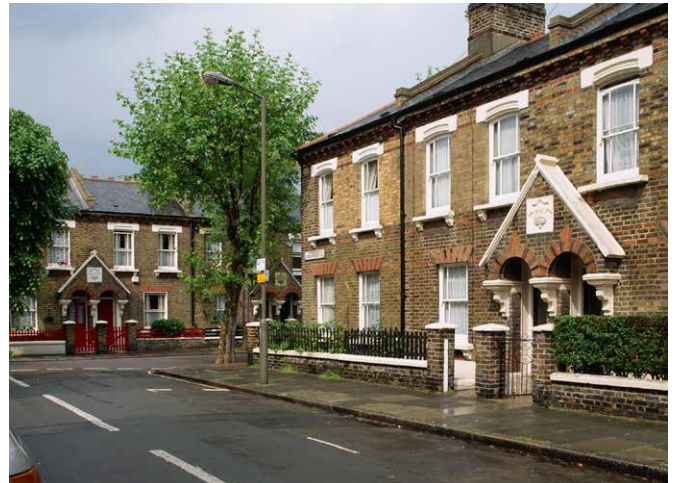
Research has shown that houses in conservation areas have added value and the retention of key elements such as traditional windows contributes to this. © Historic England
