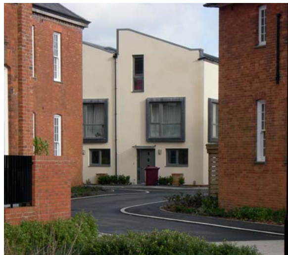
Graylingwell hospital, West Sussex, where newly built houses are sited in gaps between the converted ward blocks.
