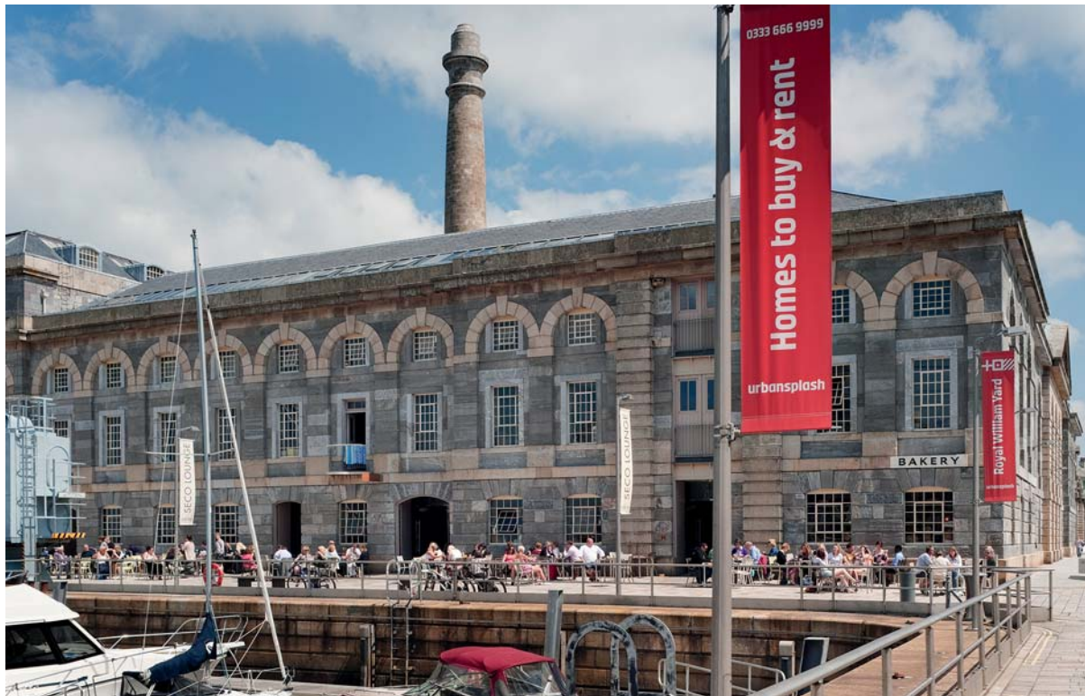
Urban Splash's conversion of the redundant Grade I Royal William Yard naval victualling depot has created a new residential and social hub for Plymouth. © Urban Splash
