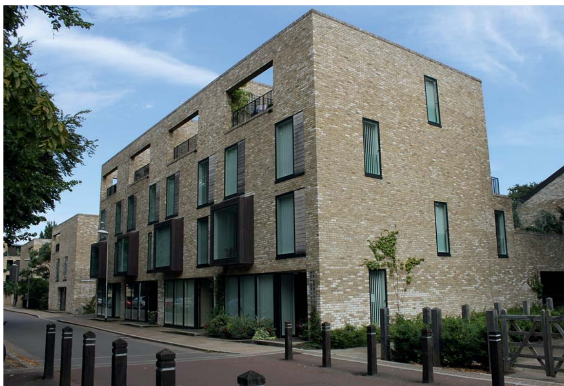
Accordia in Cambridge – a contemporary reinterpretation of the Georgian townhouse. © Peter Studdert
