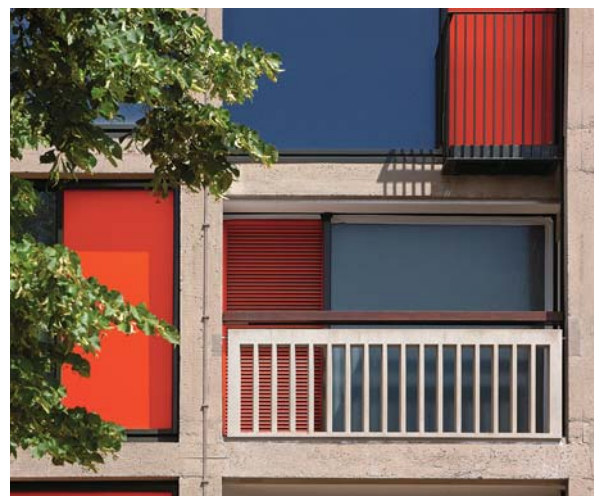
With advice from English Heritage Urban Splash revitalised Sheffield City Council’s Grade II* Park Hill housing scheme in a way that preserves the historic significance of its reinforced concrete frame while allowing substantial changes to the internal layout and decorative infill panels. © Urban Splash
