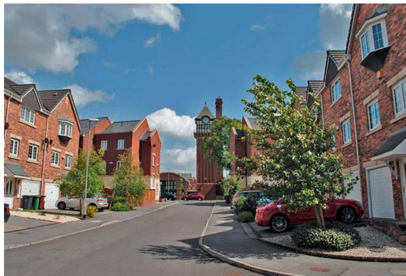
New housing development in Rothwell, Leeds, integrating the Grade II listed late-19th century clock tower. © Design for Homes
