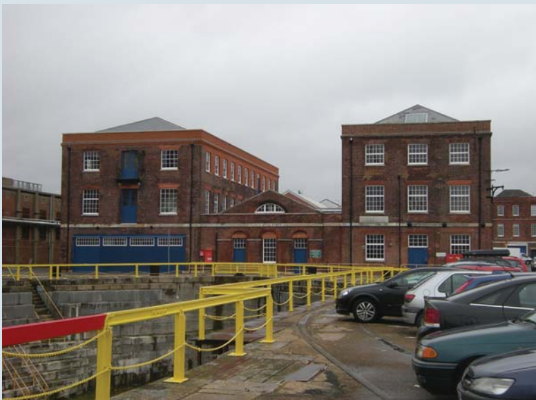
The Grade I Block Mills at Portsmouth, one of the most important buildings of the Industrial Revolution, has at last been removed from the Heritage at Risk Register; although its long-term future has still to be agreed.
