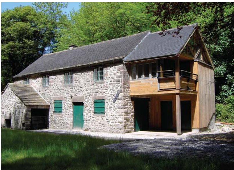
Slinger Woods, Cromford, Derbyshire. This former water-powered bobbin mill has been restored as a holiday cottage by the Arkwright Society, an educational charity devoted to the rescue of industrial heritage buildings in and around Cromford.
