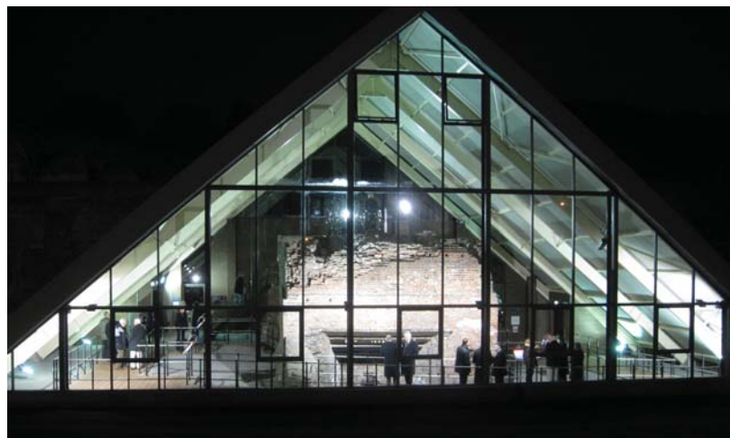
A UK Anchor Point: the blast furnace, Museum of Iron, Coalbrookdale, part of the Ironbridge Gorge Museum complex.
