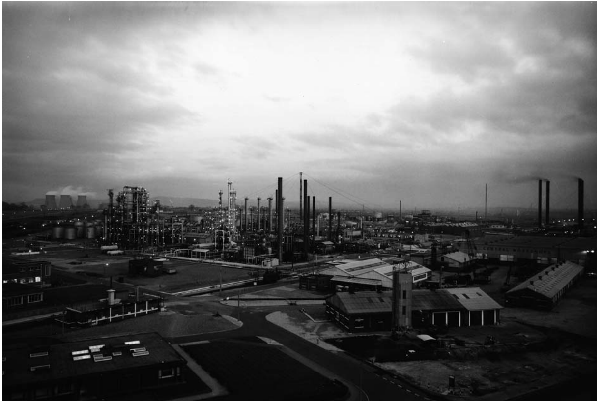
The Stanlow oil refinery in Ellesmere Port, Cheshire. Reproduced by permission of English Heritage.NMR
