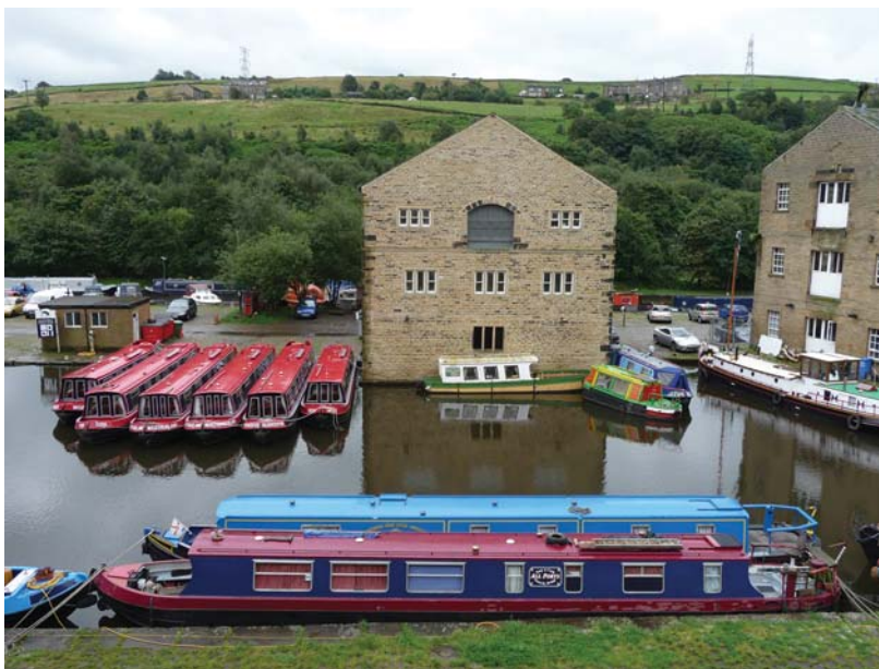
The conversion of these canal warehouses at Sowerby Bridge Wharf in West Yorkshire into space for small businesses shows how industrial heritage can be adapted to meet the needs of modern working life. The project was led by The Prince's Regeneration Trust with partnership support from Heritage Lottery Fund, Calderdale Council, British Waterways, Yorkshire Forward and stakeholders in the local community.
