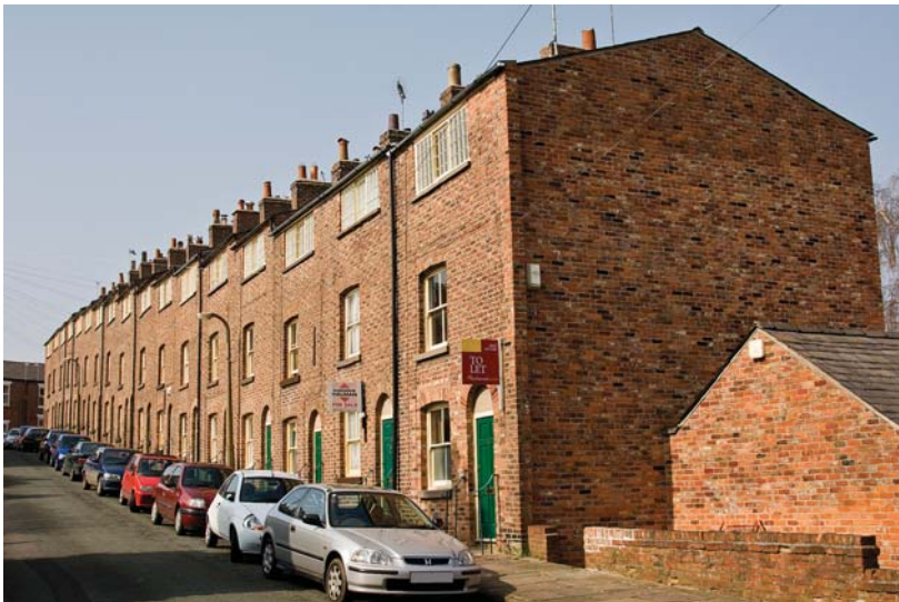
Paradise Street, Macclesfield. Built for home-working silk weavers, the houses had a basic two-up-and-two-down layout but the very top floor was completely open. ‘I can remember hearing a loom working in one of these in the mid-sixties. My grandfather was born in one of them in the late 1880s. I like the way they have been built to accommodate the slope.’
