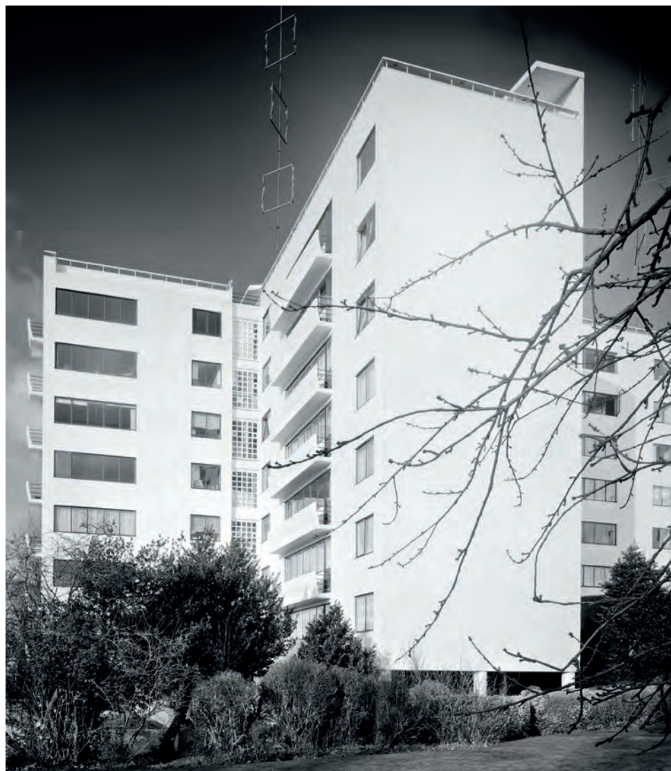
Highpoint I, Highgate, London, 1933–35. The flats were originally commissioned to house staff from the Gestetner company. Corbusier described them as “an achievement of the first rank” .
