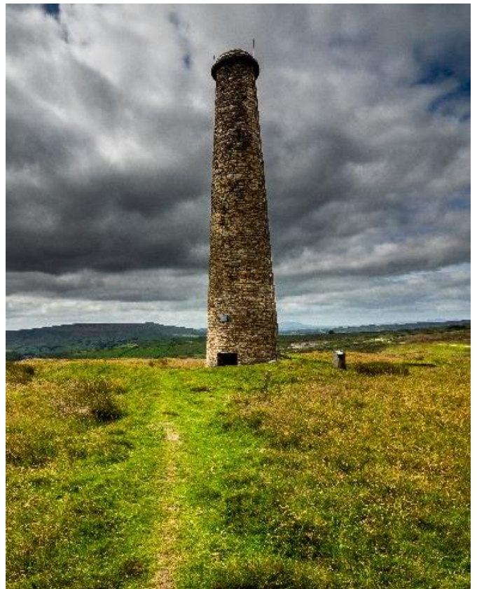
Figure 2.8: Grassington Moor smelt mill chimney
