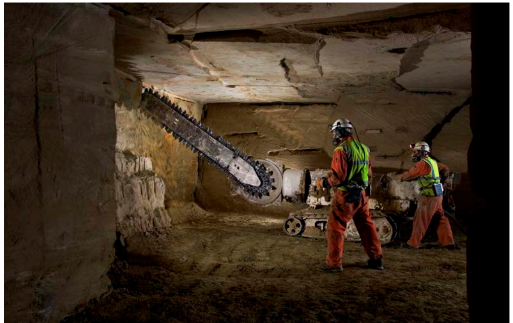
Figure 11: Underground quarry, Chilmark. Chilmark Stone.
