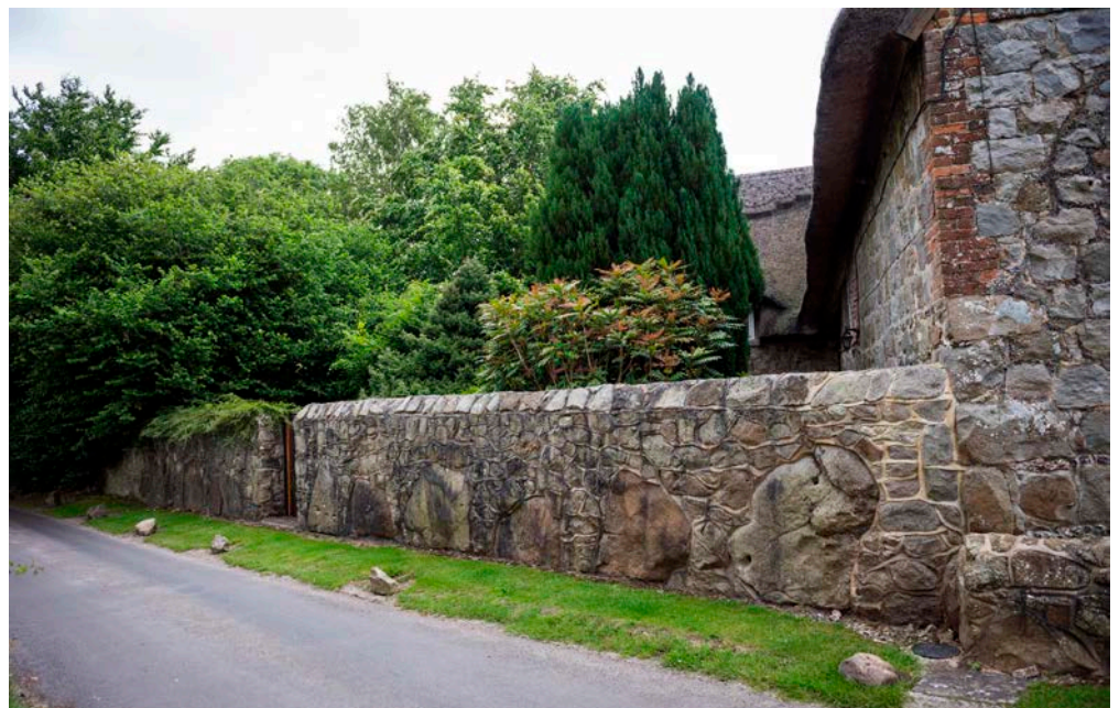
Figure 18: Building and garden walls, East Kennet. Sarsen stone.
