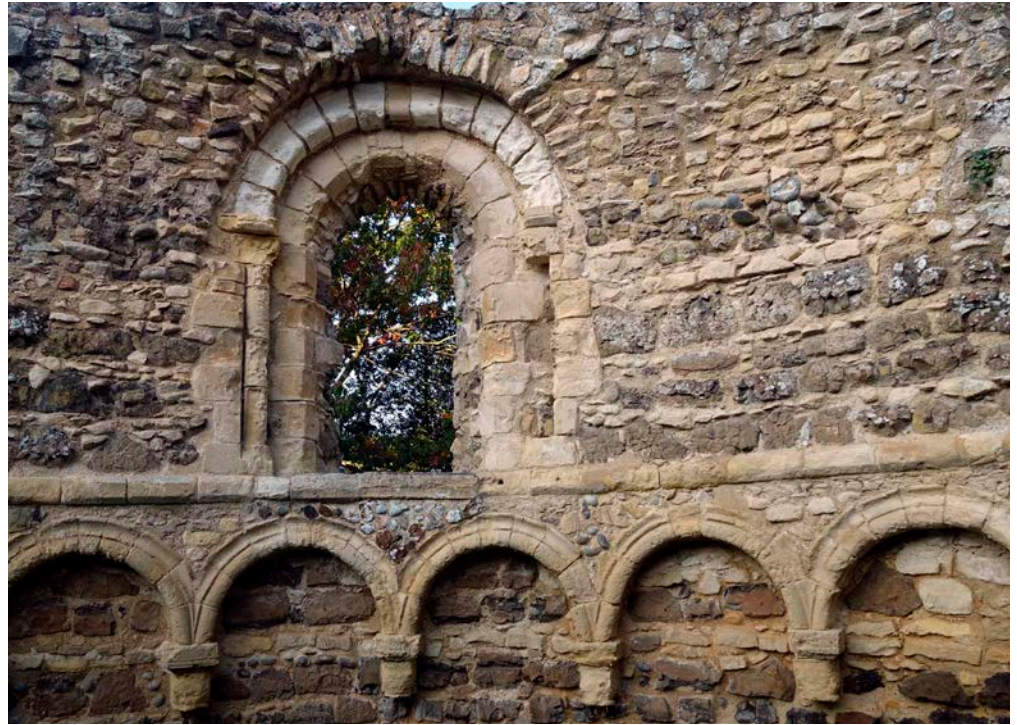
Figure 50: Leper Chapel, Dunwich. Caen Stone, London Clay septaria, flints and other materials.
