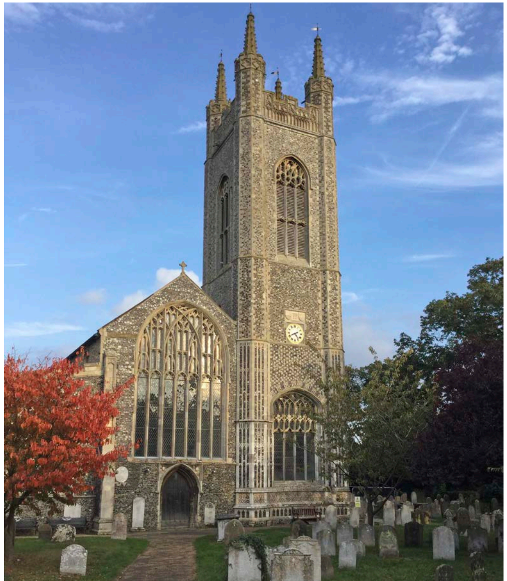
Figure 8: St Mary's Church, Bungay. Flint, septaria, limestone, brick and pebbles, with Lincolnshire Limestone dressings.
