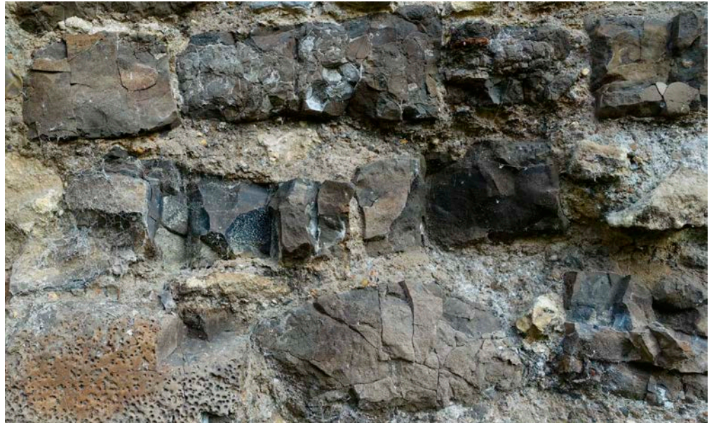
Figure 30: Leper Chapel, Dunwich. Septaria.
