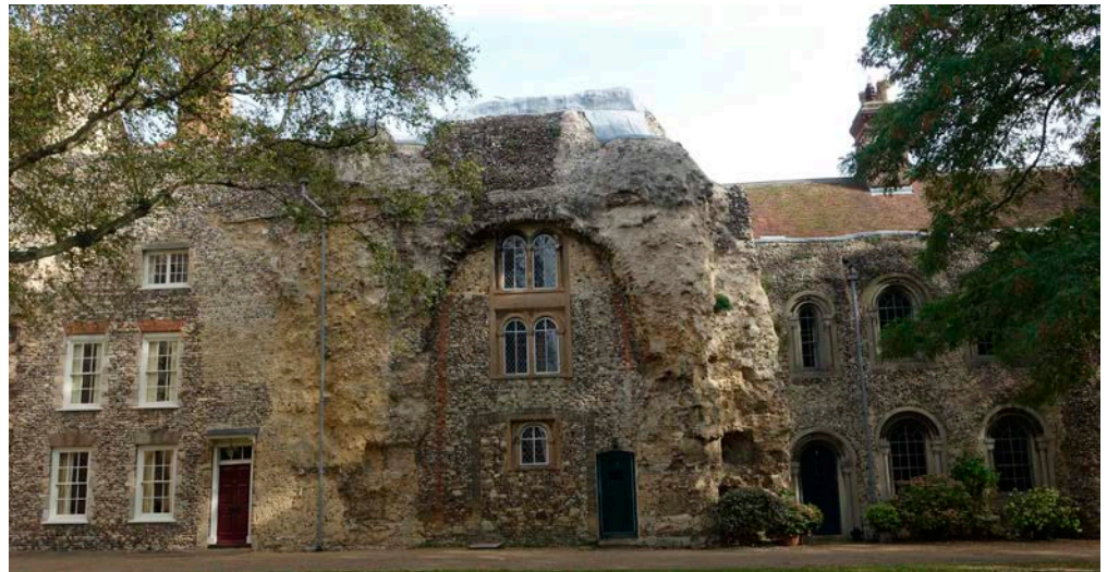
Figure 2: Abbey west front, Bury St Edmunds. Quaternary Flint pebbles and blocks of Caen Stone and Barnack Stone.
