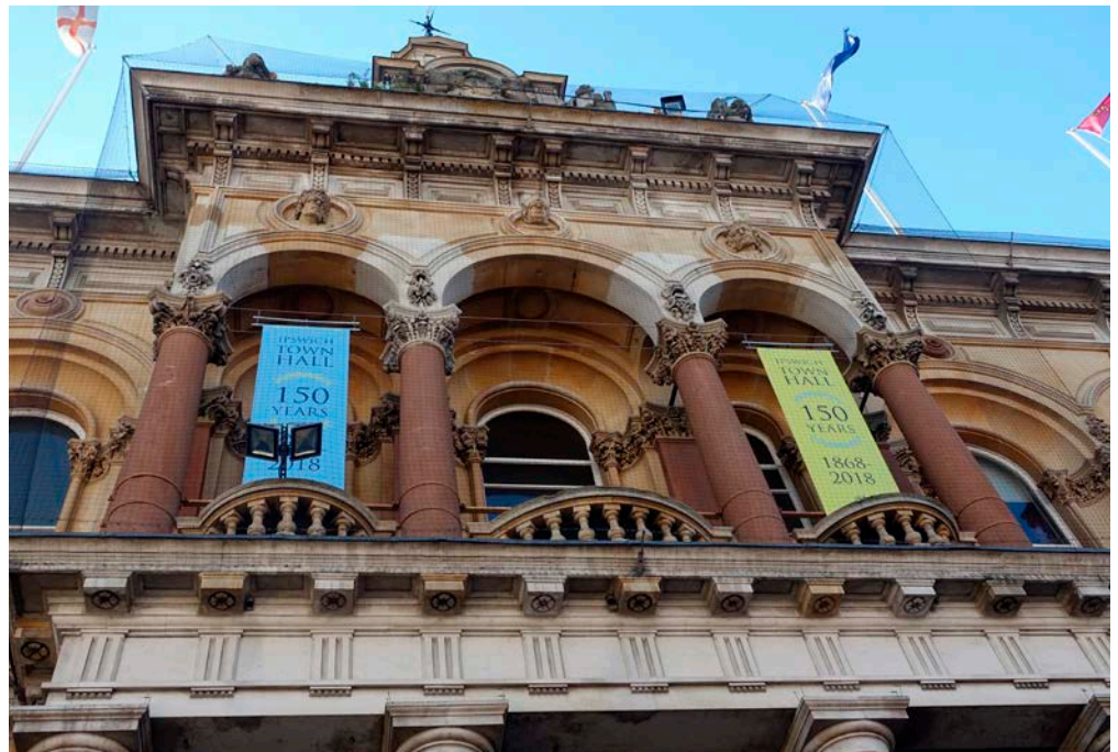
Figure 49: Ipswich Town Hall, Ipswich. Bath Stone ashlar with Red Mansfield Stone pillars.
