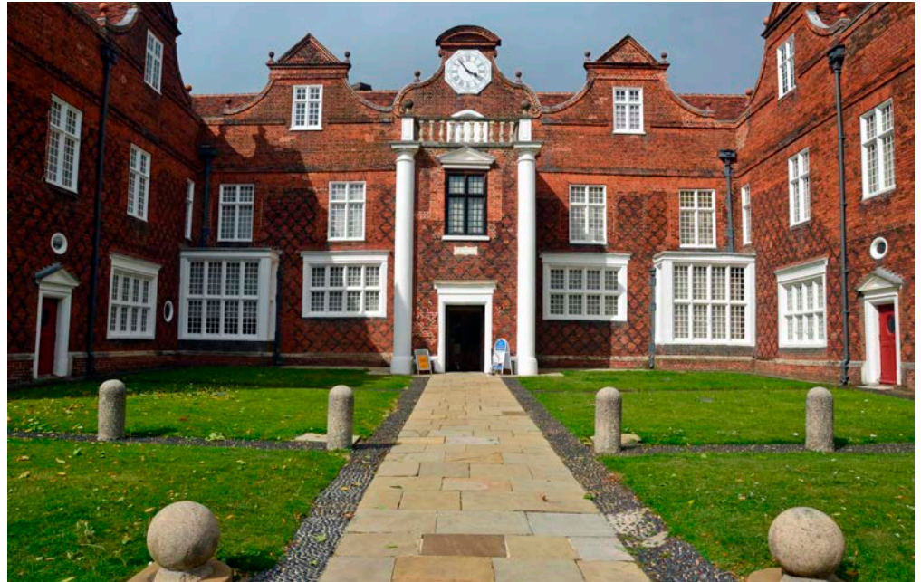
Figure 44: Christchurch Mansion, Christchurch Park, Ipswich. Yorkshire Flagstone paving.
