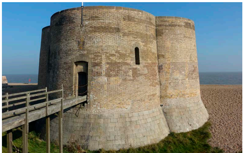
Figure 54: Martello Tower, Aldeburgh. Brick on granite ashlar plinth.
