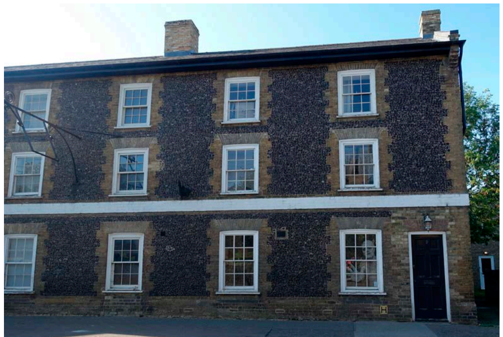
Figure 26: 19th-century House, Lakenheath. Knapped and roughly coursed nodules of Quarry Flint with buff brick dressings.
