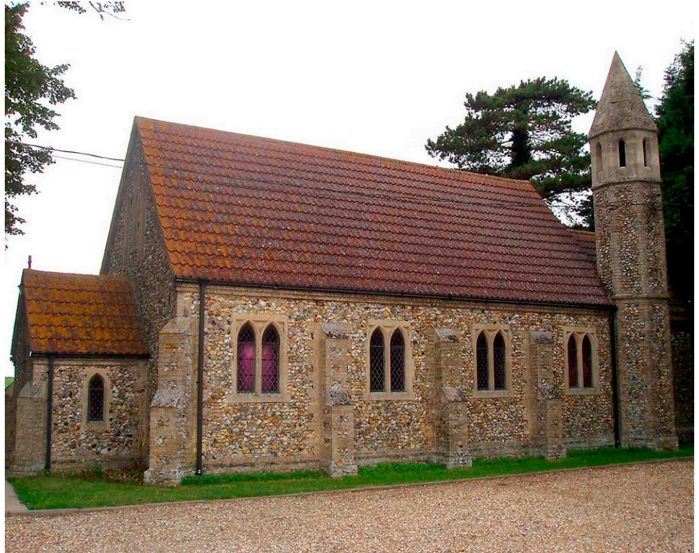
Figure 6: St James' Church, Kenny Hill. Quaternary Flint with Lincolnshire Limestone dressings.
