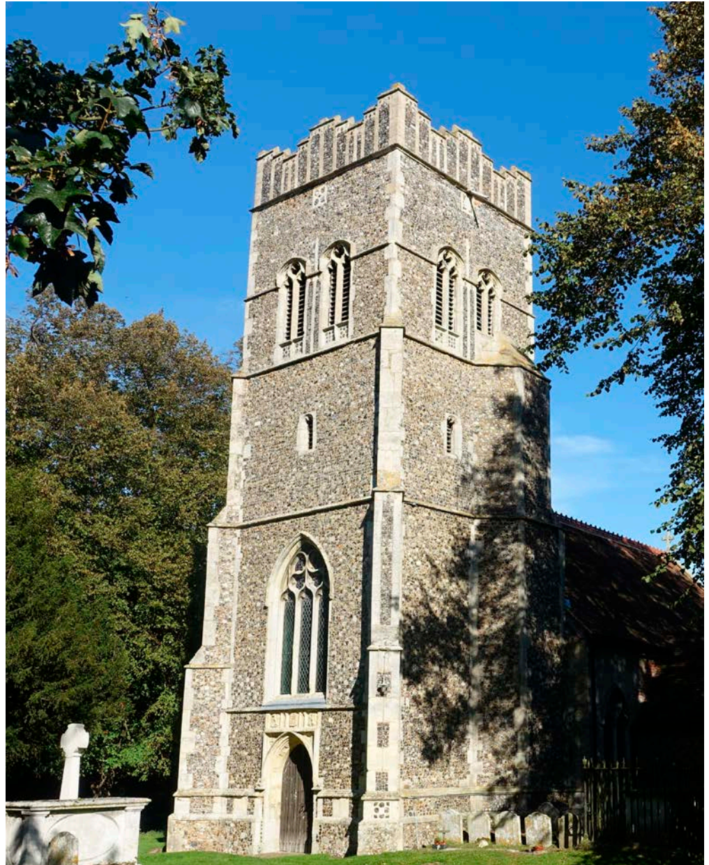
Figure 40: St Ethelbert's Church, Falkenham. Quaternary Flint, chert, quartzite, exotic stones and septaria.
