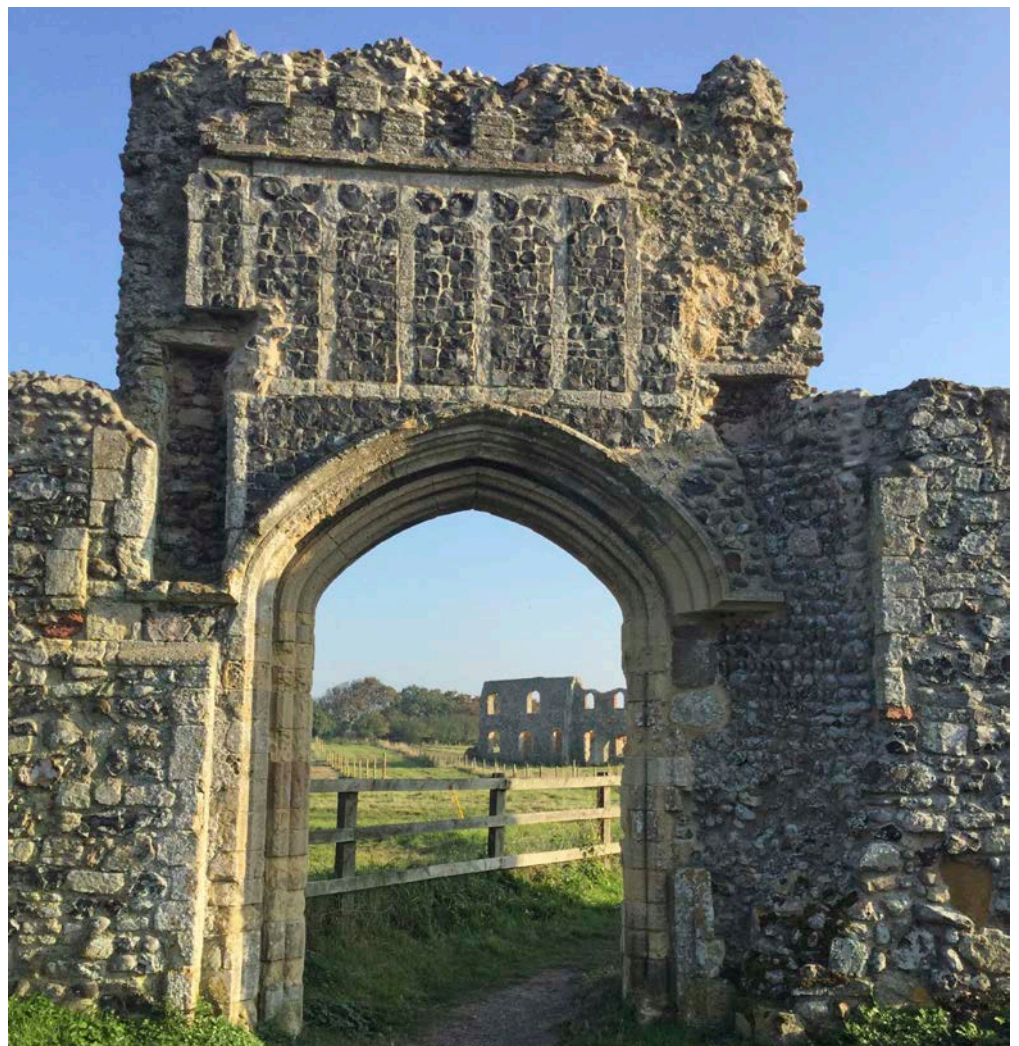
Figure 10: Greyfriars Priory, Dunwich. Flint flushwork and Caen Stone dressings.
