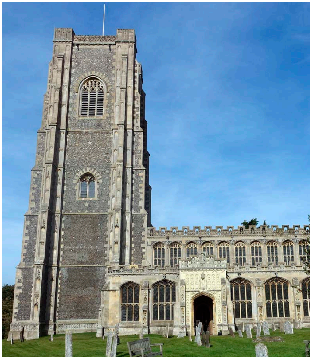
Figure 46: Church of St Peter and St Paul, Lavenham. Knapped flint and Casterton-type stone.
