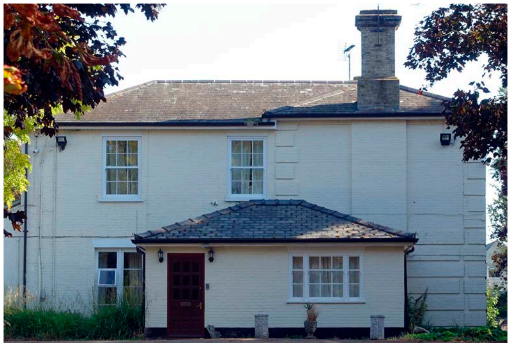
Figure 58: Shakespeare Lodge, Back Street, Lakenheath. Welsh Slate roof.
