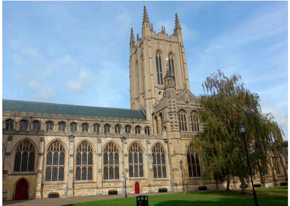
Figure 47: St Edmundsbury Cathedral, Bury St Edmunds. Lincolnshire Limestone and Clipsham Stone.
