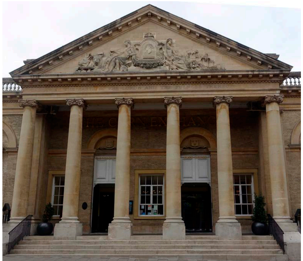
Figure 48: Corn Exchange, Bury St Edmunds. Ancaster Stone and Portland Stone.
