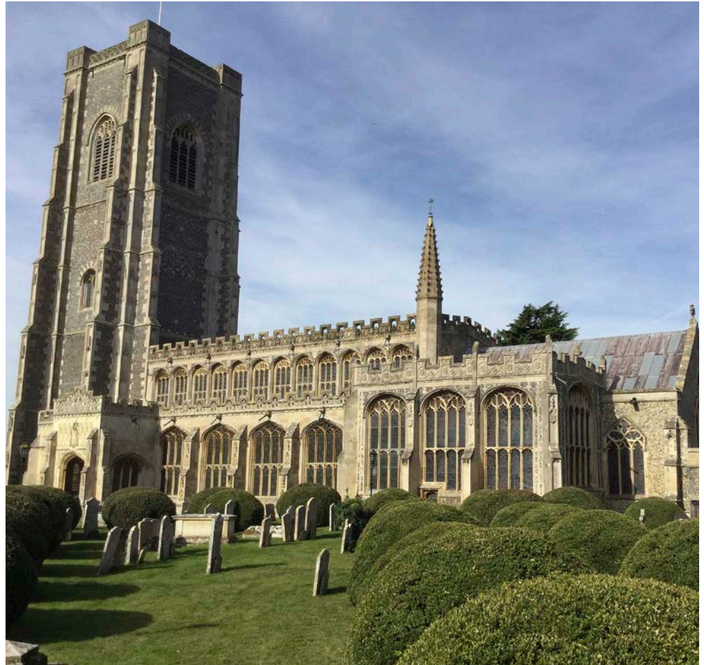
Figure 18: SS Peter and Paul's Church, Lavenham. Knapped Quaternary Flint, with ornamental flushwork, limestone ashlar and Casterton Stone dressings.
