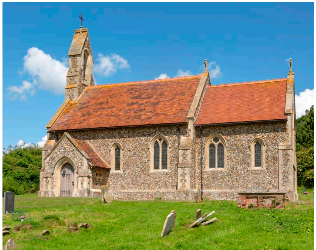
Figure 19: Church of St Mary, Willisham. Flint and septaria rubble with freestone dressings.
