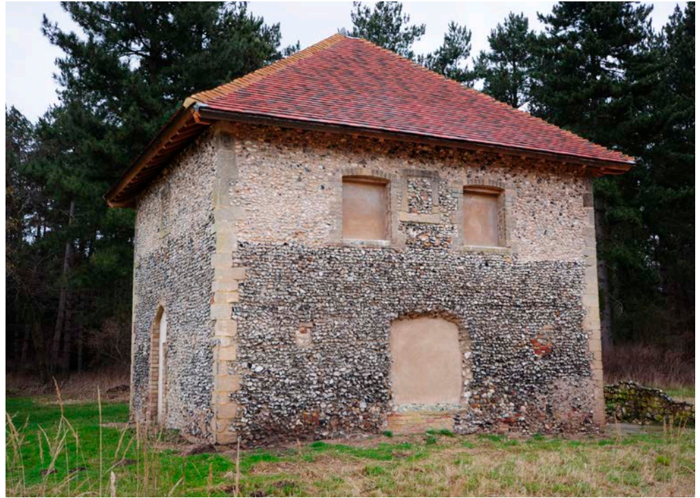
Figure 16: Mildenhall Warren Lodge, Mildenhall. Quaternary Flint pebbles and nodules with limestone quoins.
