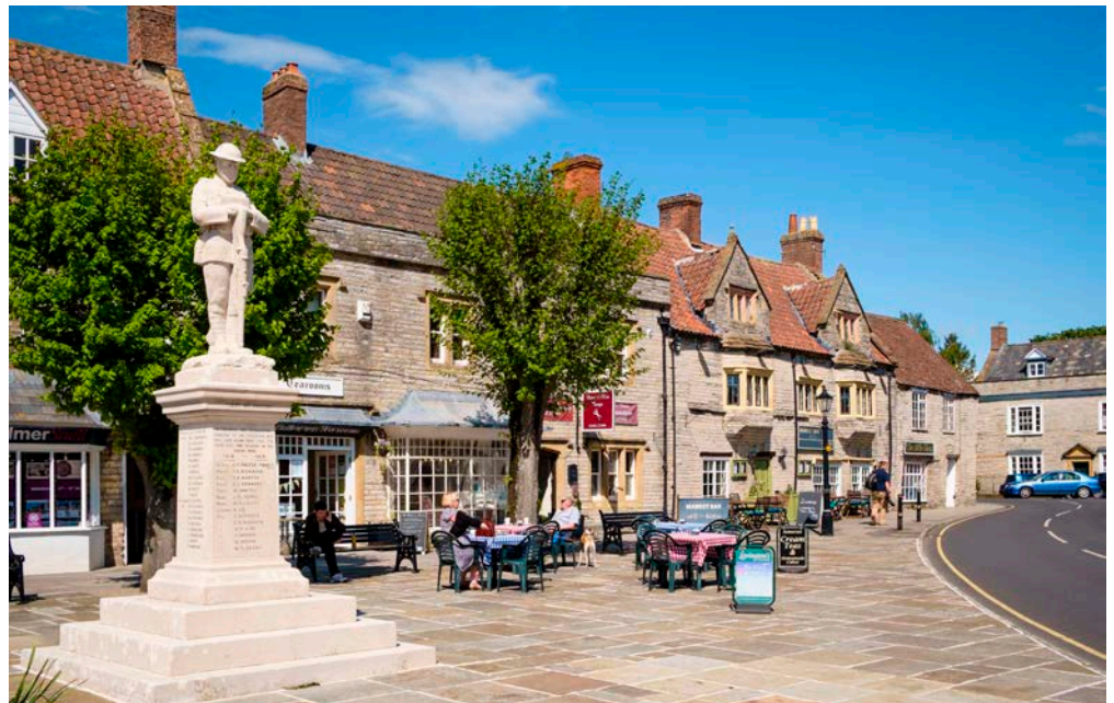
Figure 12: Village buildings, Somerton. Blue Lias, some Douling Stone or Ham Stone dressings.
