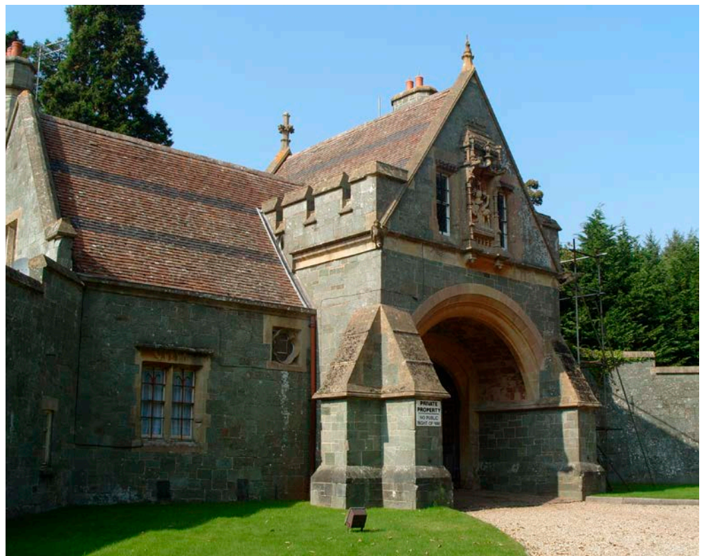
Figure 4: Gatehouse, Quantock Lodge, Over Stowey. Cockercombe Tuff with Bath Stone and Otter Sandstone dressings.
