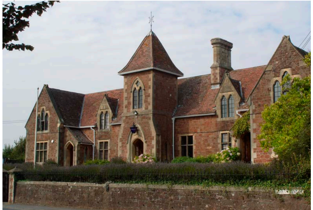
Figure 8: Former Police Station, Priest Street, Williton. Otter Sandstone, Wiveliscombe Sandstone and Hangman Sandstone.
