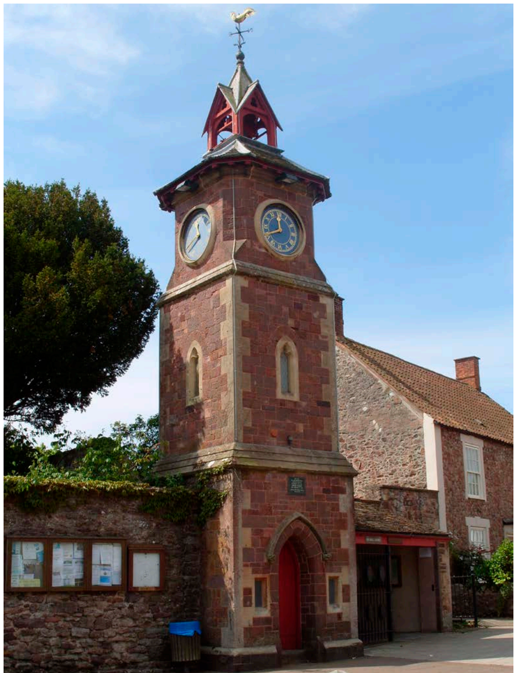
Figure 2: Clock tower, Nether Stowey. Ilfracombe Slate, Hangman Sandstone and Otter Sandstone. Doulling Stone quoins and tracery.
