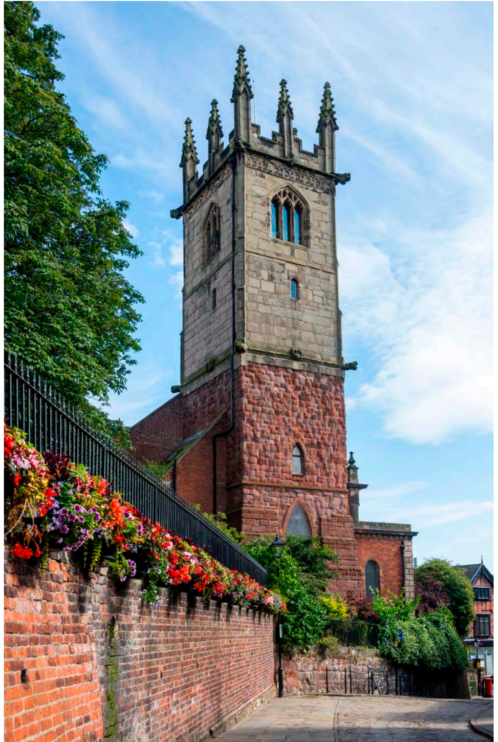
Figure 41: St Julian's Church, Shrewsbury. Keele Beds sandstone and Grinshill Stone.
