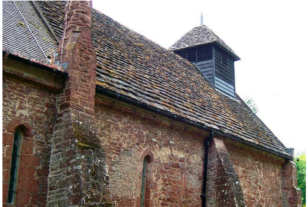
Figure 16: Church of St Michael and All Angels, Pitchford. Harnage Stone slate roof.
