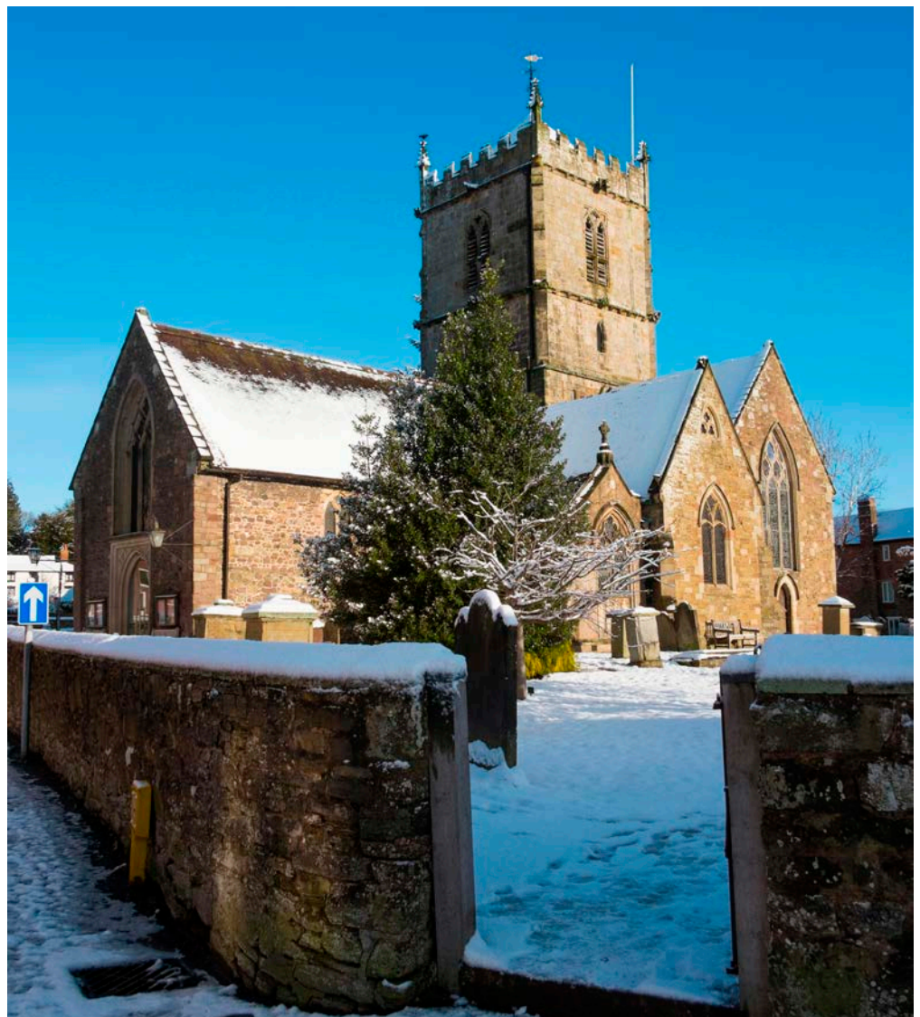
Figure 13: Tower, St Laurence Church, Church Stretton. Hoar Edge Grit.
