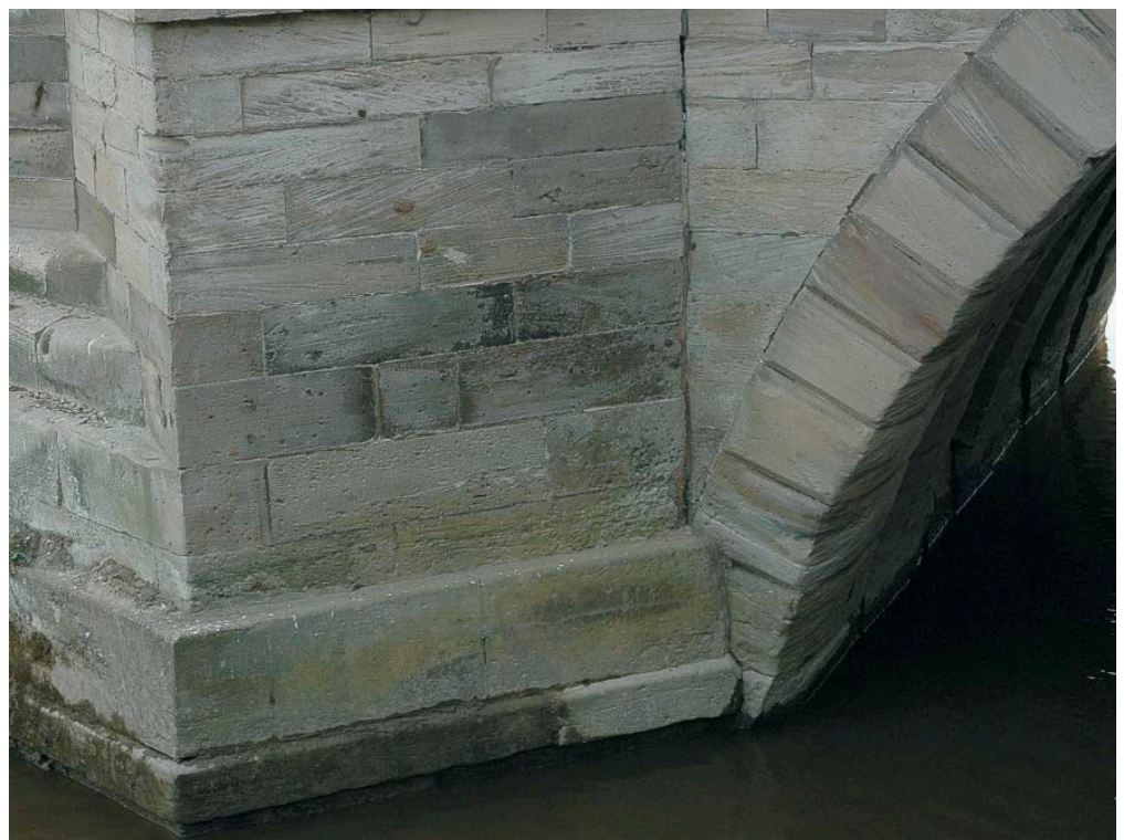
Figure 38: Bridgnorth Bridge. Highley Sandstone.
