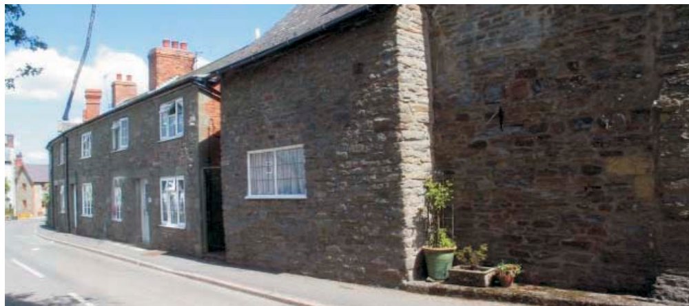
Figure 30: Cottages, Clun. Siltstone frontages.
