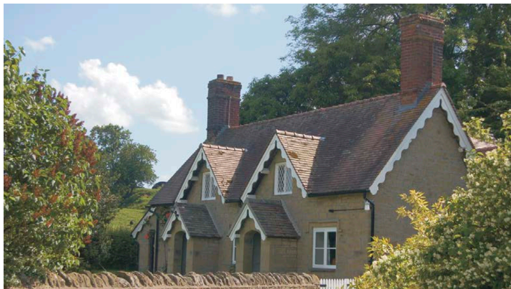
Figure 31: Cottages, Corfton. Downton Castle Sandstone.
