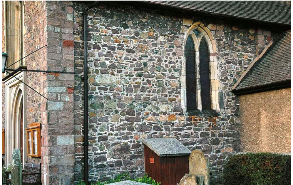
Figure 2: St Laurence's Church, Church Stretton. Longmyndian stones, with quoins of Carboniferous and Permo-Triassic sandstone. North transept is Soudley Sandstone.
