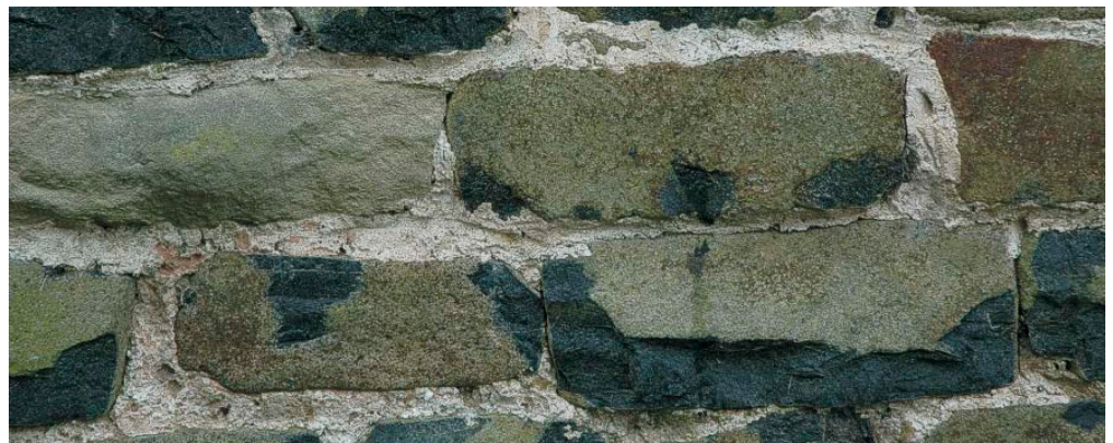
Figure 44: House wall, Cleobury North. Dhustone.
