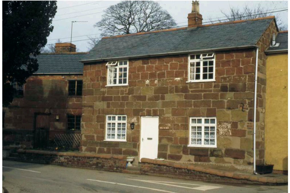
Figure 49: Cottage, Myddle. Wilmslow Sandstone.
