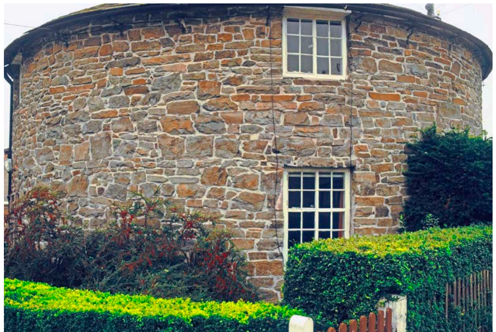
Figure 22: Former estate cottage, Clun Road, Aston on Clun. Siltstone.
