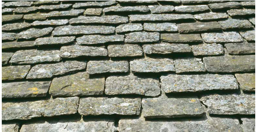
Figure 14: Langley Chapel, near Acton Burnell. Hoar Edge Grit roof slates.
