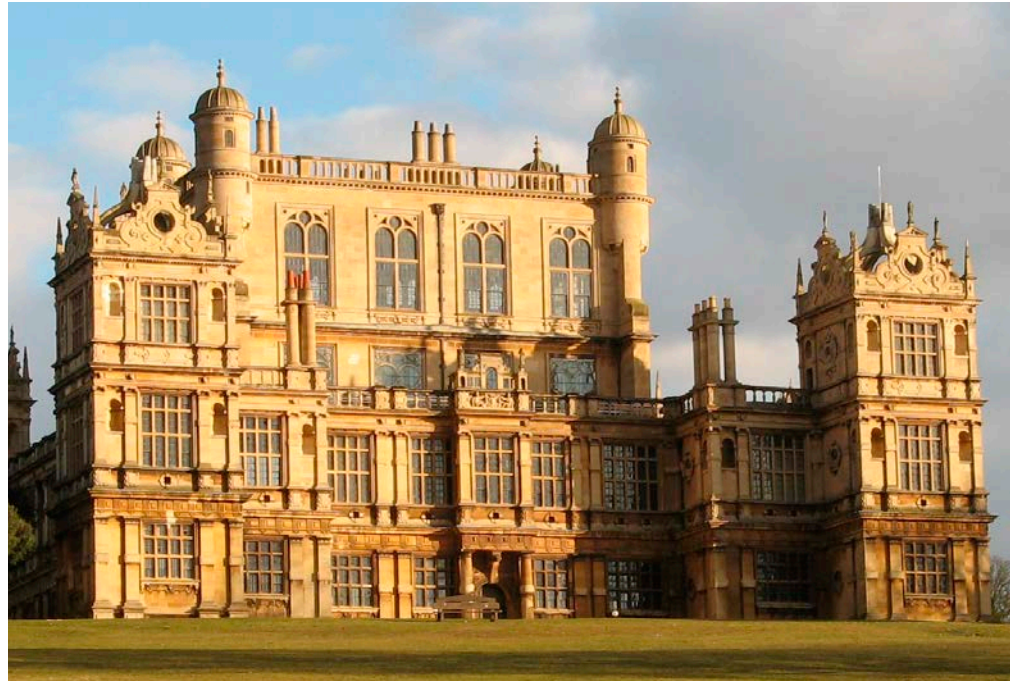
Figure 20: Wollaton Hall. Lincolnshire Limestone.
