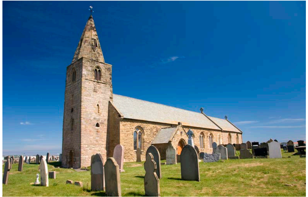
Figure 19: St Bartholomew's Church, Newbiggin-by-the-Sea. Middle Coal Measures Sandstone.
