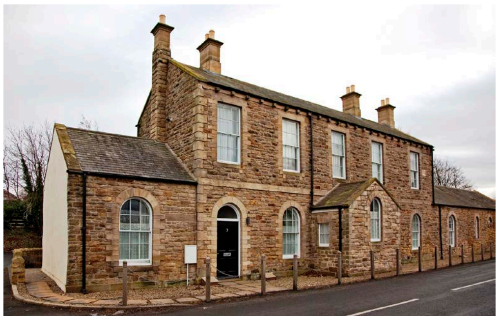
Figure 15: Old station buildings, Morpeth. Lower Coal Measures Sandstone.
