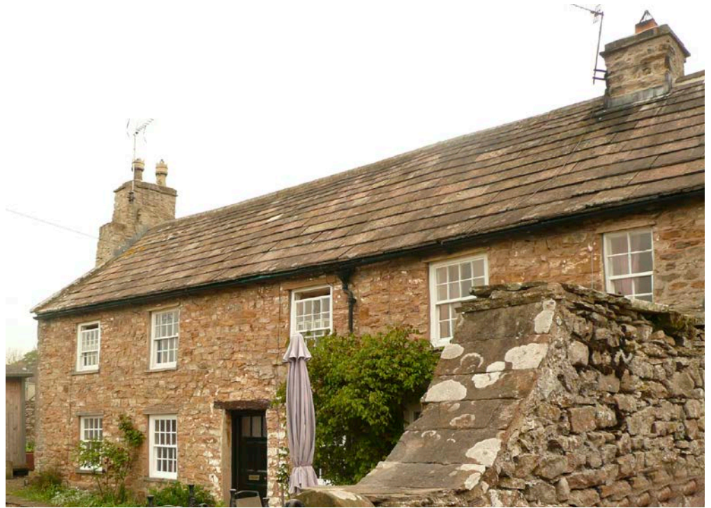
Figure 8: Manor House, Redmire, Wensleydale. Yoredale Group sandstone roof slates and lintels.
