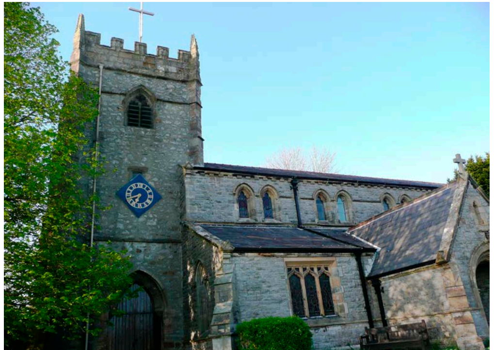
Figure 19: Church of St Mary, Ingleton. Malham Formation limestone with pebbles of Ingletonian slate (nave); limestone rubblestone and sandstone blocks (tower); Eldroth Grit sandstone windows, quoins and buttresses.
