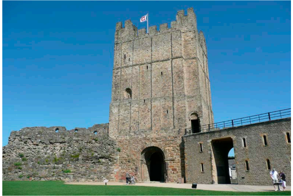
Figure 26: Richmond Castle, Richmond. Ten Fathom Grit, Stainmore Formation limestones and Underset Sandstone.
