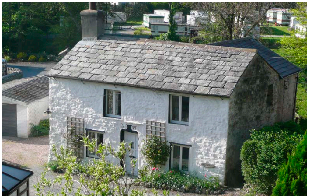
Figure 11: Cottage, Ingleton. Ingleton Slate roof.
