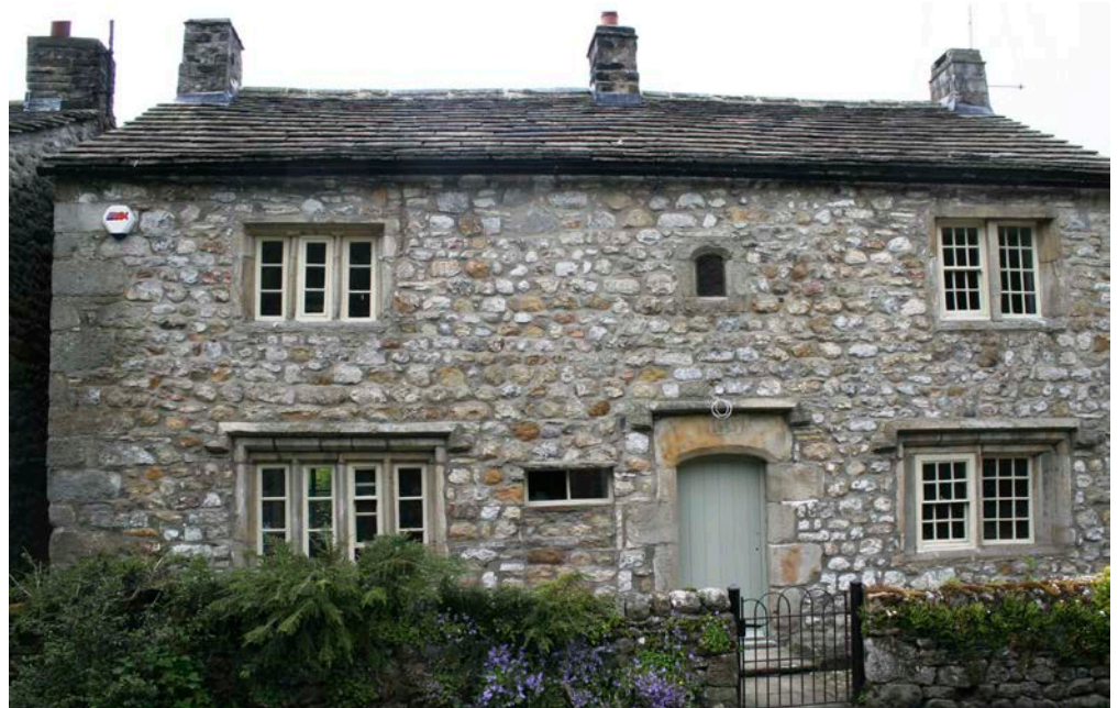
Figure 14: Yeomans Cottage, Kirkby Malham. Craven Group limestone and sandstone rubblestone. Millstone Grit sandstone dressings.
