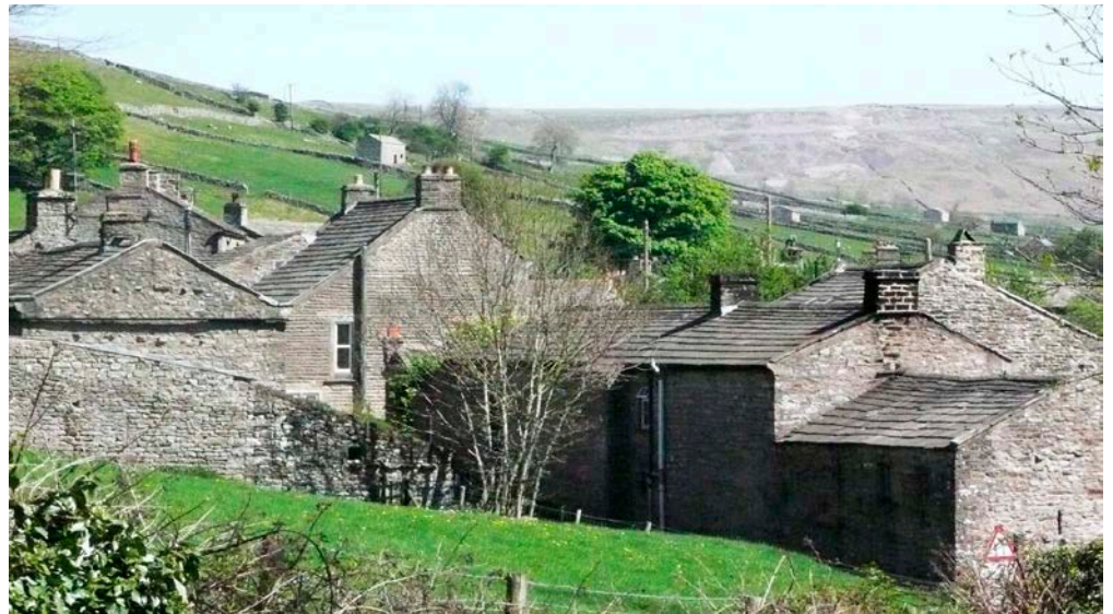
Figure 9: Healaugh village, Swaledale. Yoredale sandstone slates.
