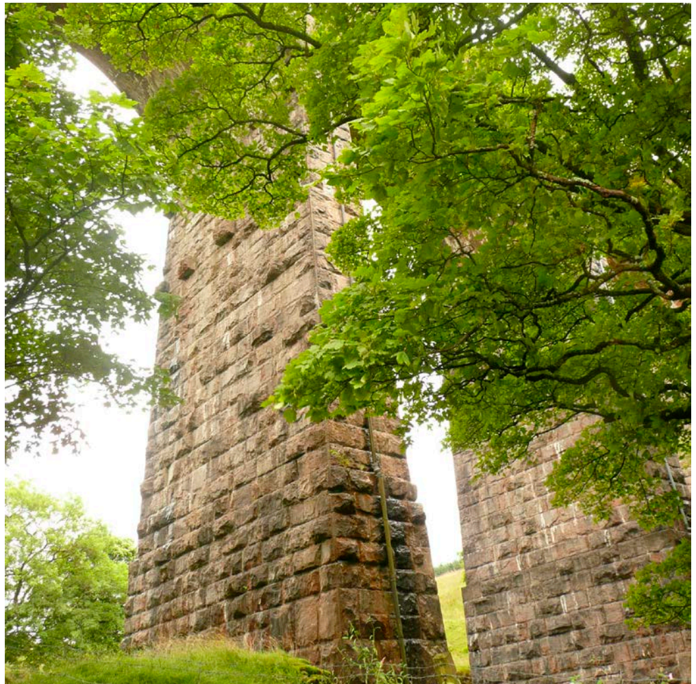
Figure 23: Dent Head viaduct. Hardraw Scar Limestone and Simonstone Limestone.
