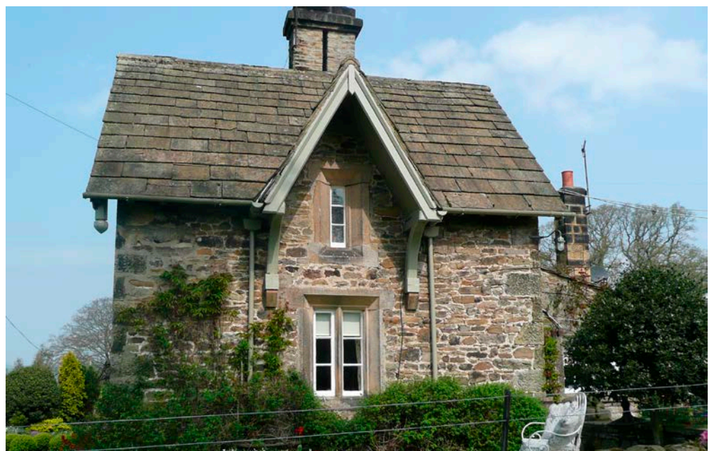
Figure 10: Hardy Grange Farmhouse, Beamsley. Millstone Grit Group sandstone roof slates.
