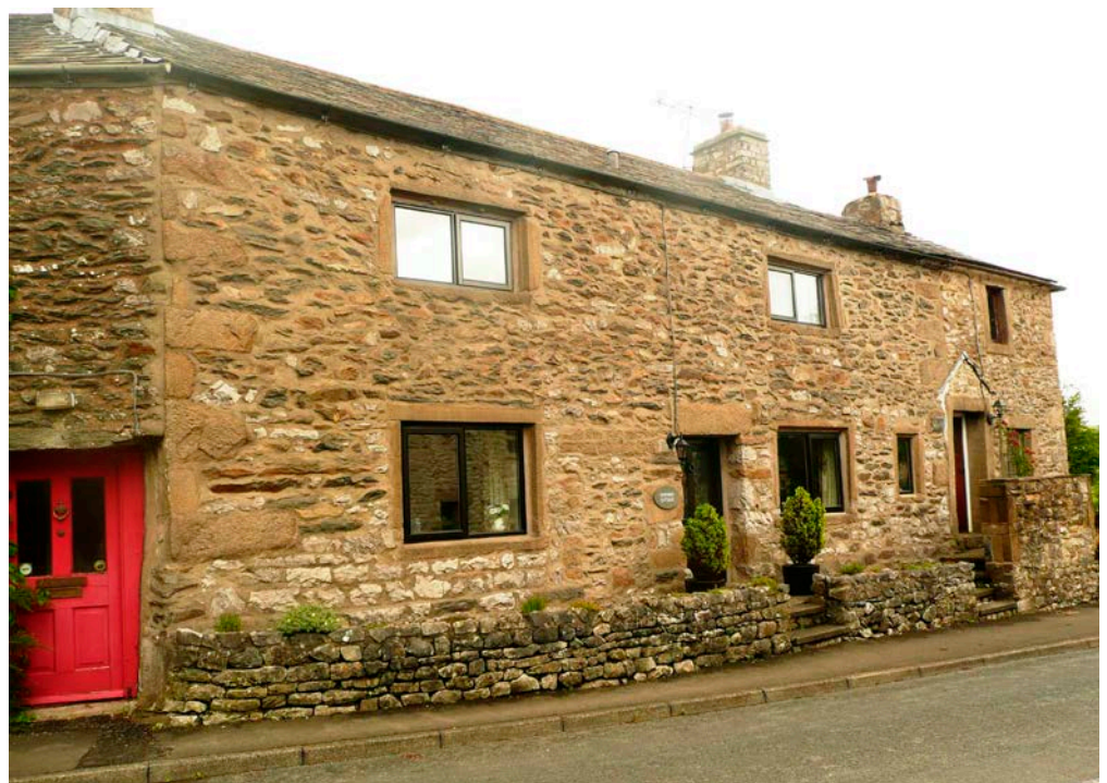
Figure 18: Oxenber Cottage, Hollin Hill, Austwick. Carboniferous limestone and Palaeozoic rubblestone.
