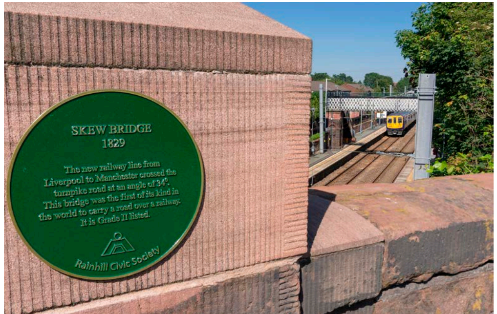
Figure 9: Skew Bridge, Rainhill Station. Rainhill Stone.
