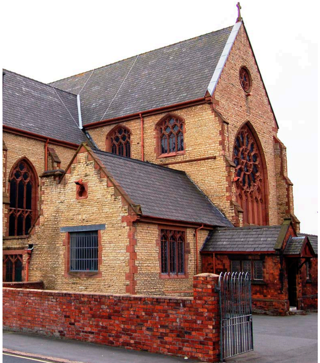
Figure 2: Holy Cross and St Helen Church, St Helens. Yellow Carboniferous sandstone coursed masonry (probably Milnrow Sandstone) and red sandstone dressings.
