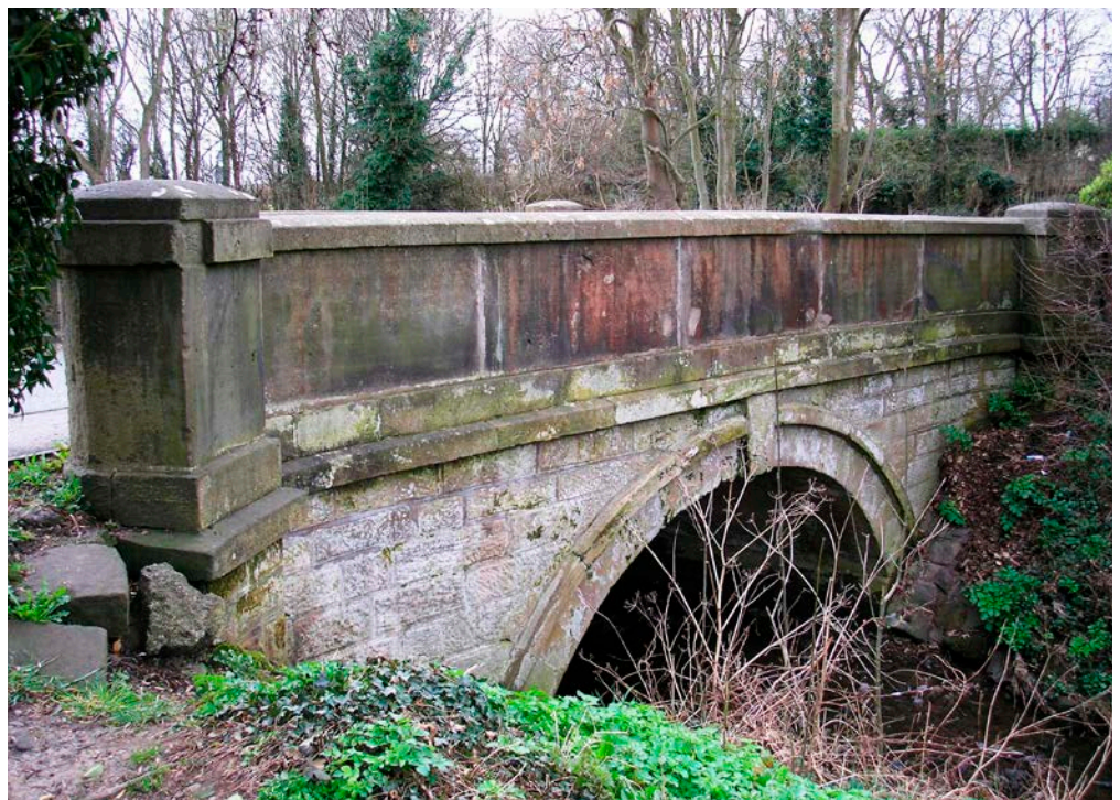
Figure 21: Road bridge at Saughall Massie, Wirral. Storeton Stone.
