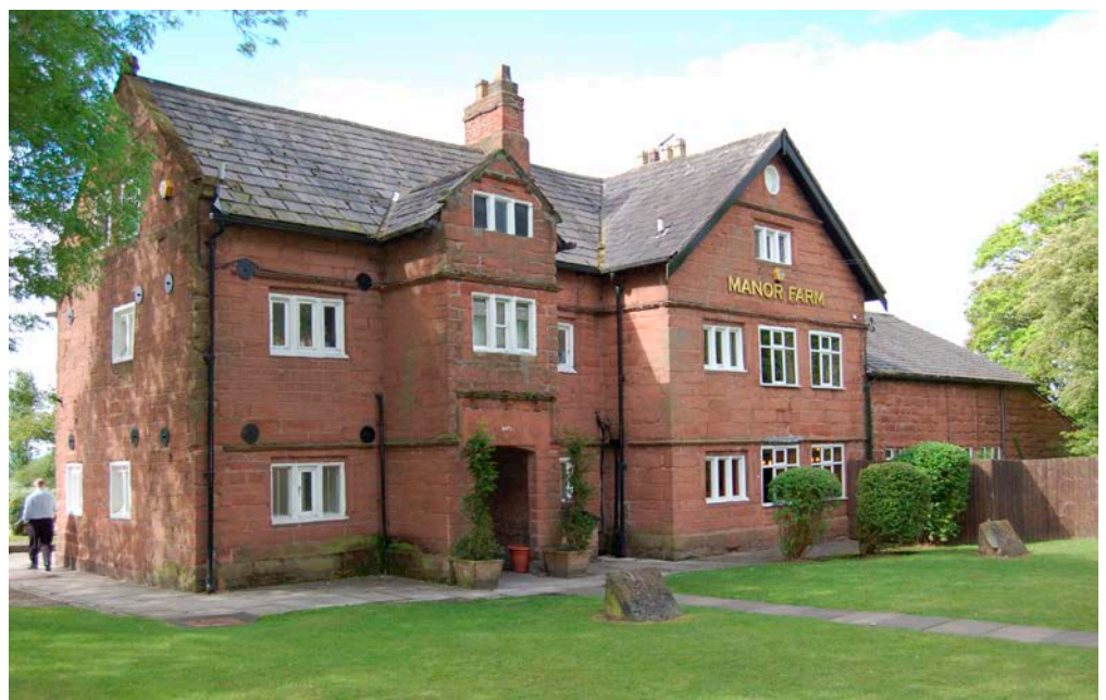
Figure 7: Manor Farm pub, Rainhill. Rainhill Stone.
