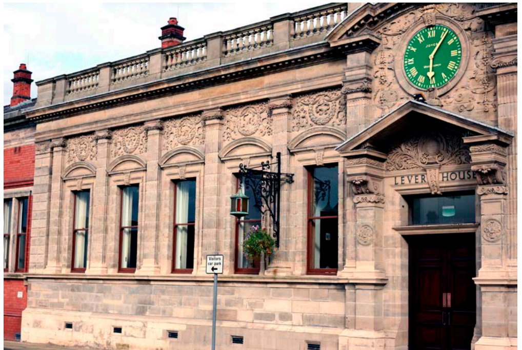
Figure 17: Lever House, Port Sunlight. Storeton Stone.
