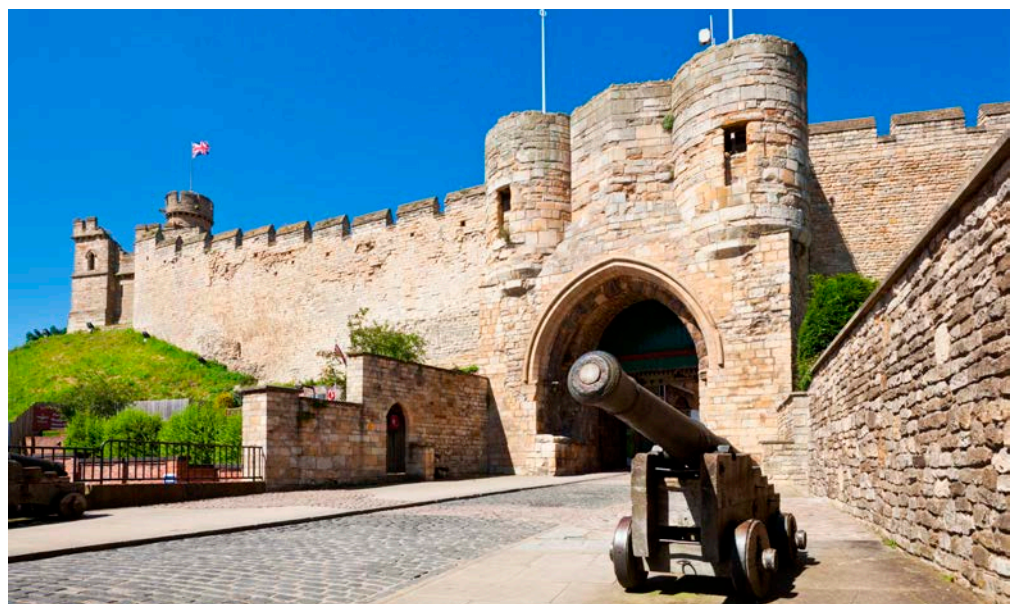
Figure 9: Curtain wall and east gateway, Lincoln Castle. Lincolnshire Limestone.
