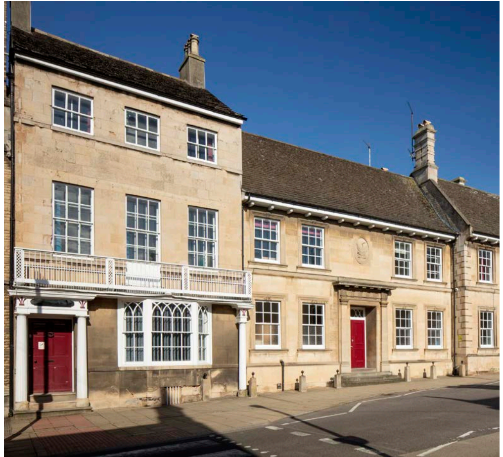
Figure 11: St Martin's Place, Stamford. Lincolnshire Limestone.
