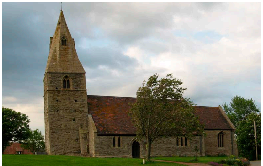
Figure 4: Church of St James, Dry Doddington. Blue Lias and Lincolnshire Limestone.
