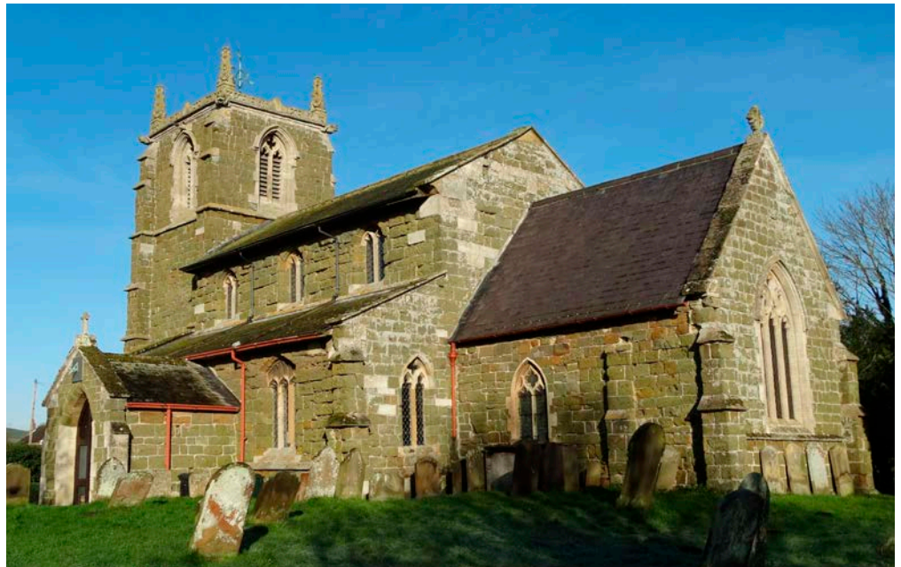
Figure 13: St Mary's Church, Tetford. Spilsby Sandstone.
