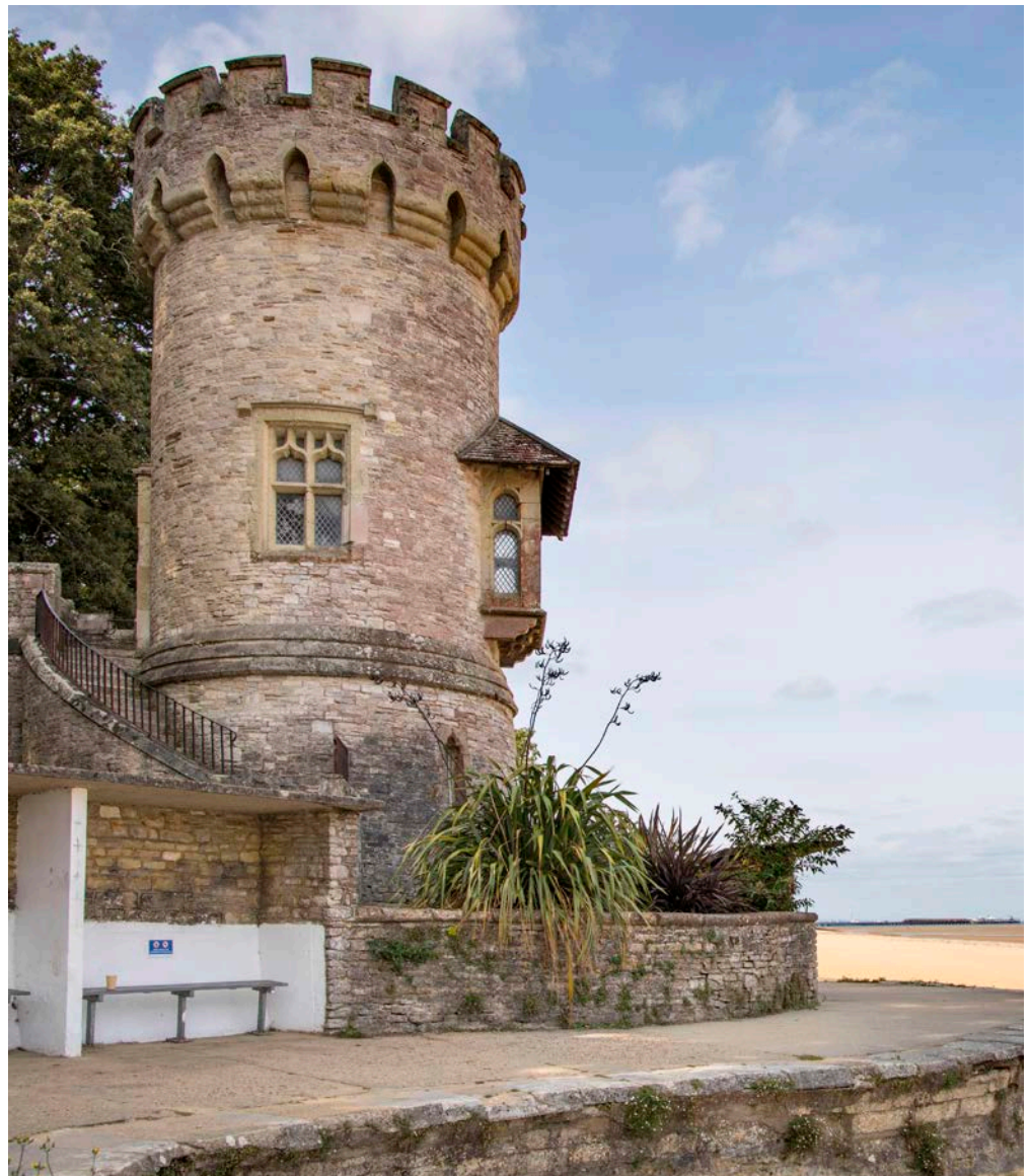
Figure 17: Appley Tower, Ryde. Nettlestone Sandstone, Featherstone, Bembridge Limestone, Upper Greensand Sandstone and Monk's Bay Sandstone.
