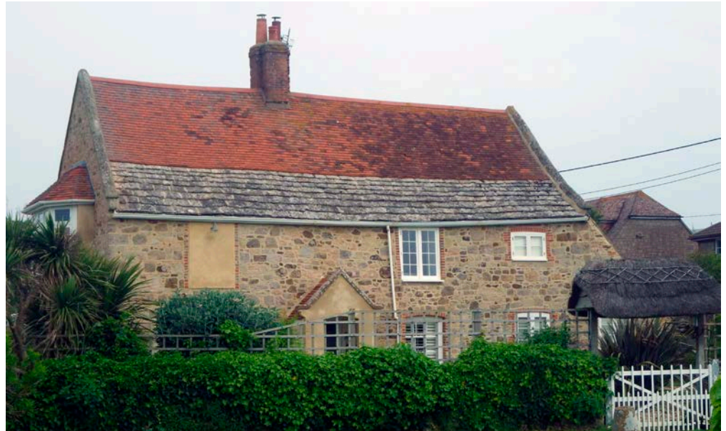
Figure 25: Hanover House, Coastguard Lane, Brook. Purbeck Stone slate roof.
