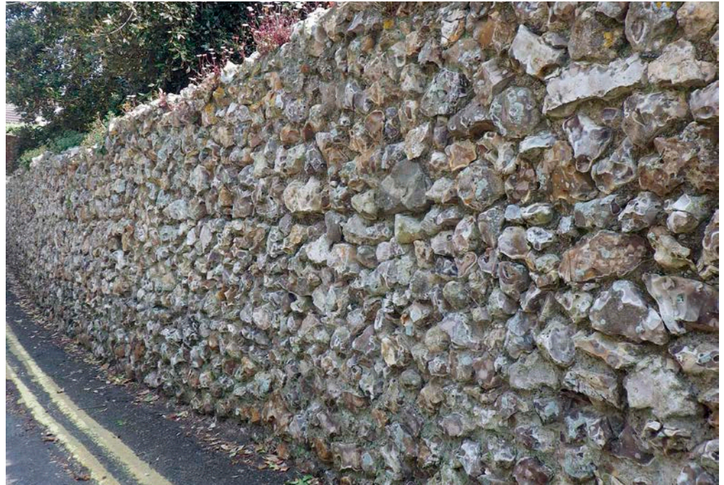
Figure 13: Wall, Kings Bay Road, Bonchurch. Flint and chert.
