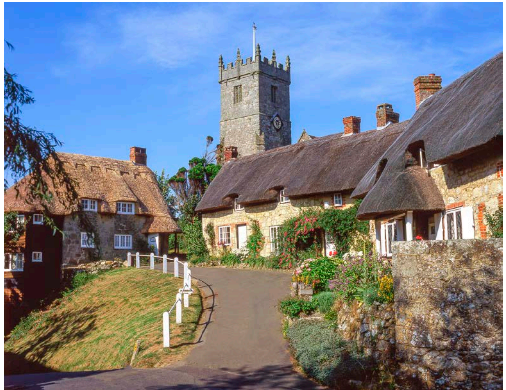
Figure 1: Cottages, Godshill. Chert and Upper Greensand Sandstone.
