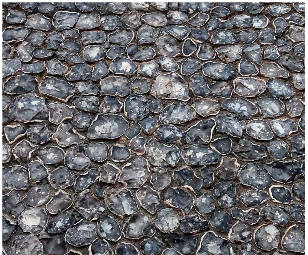
Figure 18: Old School House, Wheathampstead. Knapped flint nodules.
