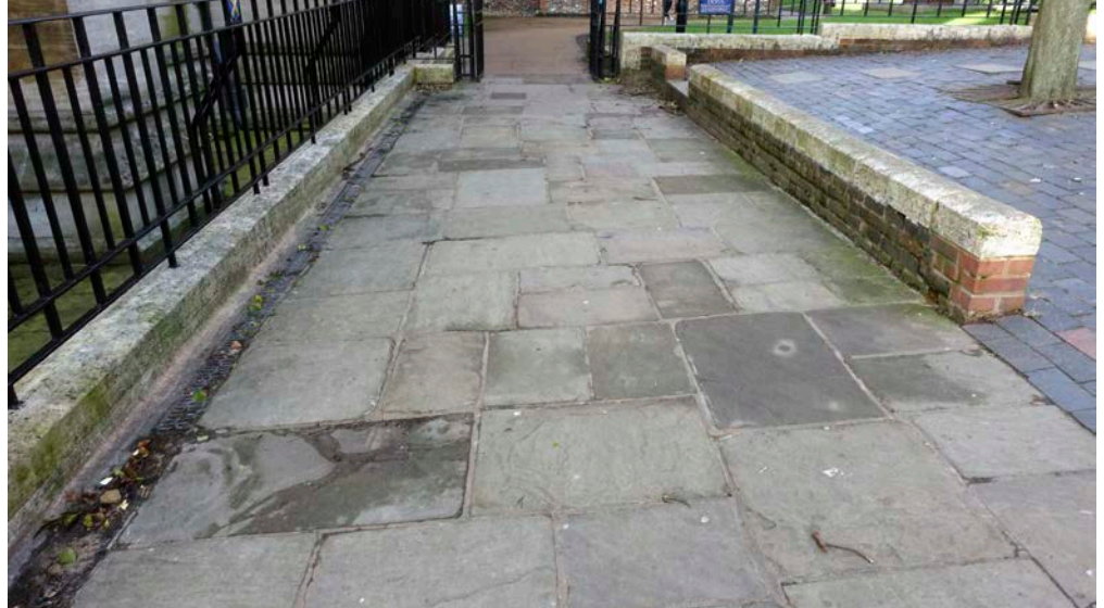
Figure 42: Cathedral path, St Albans. York Stone paving slabs.
