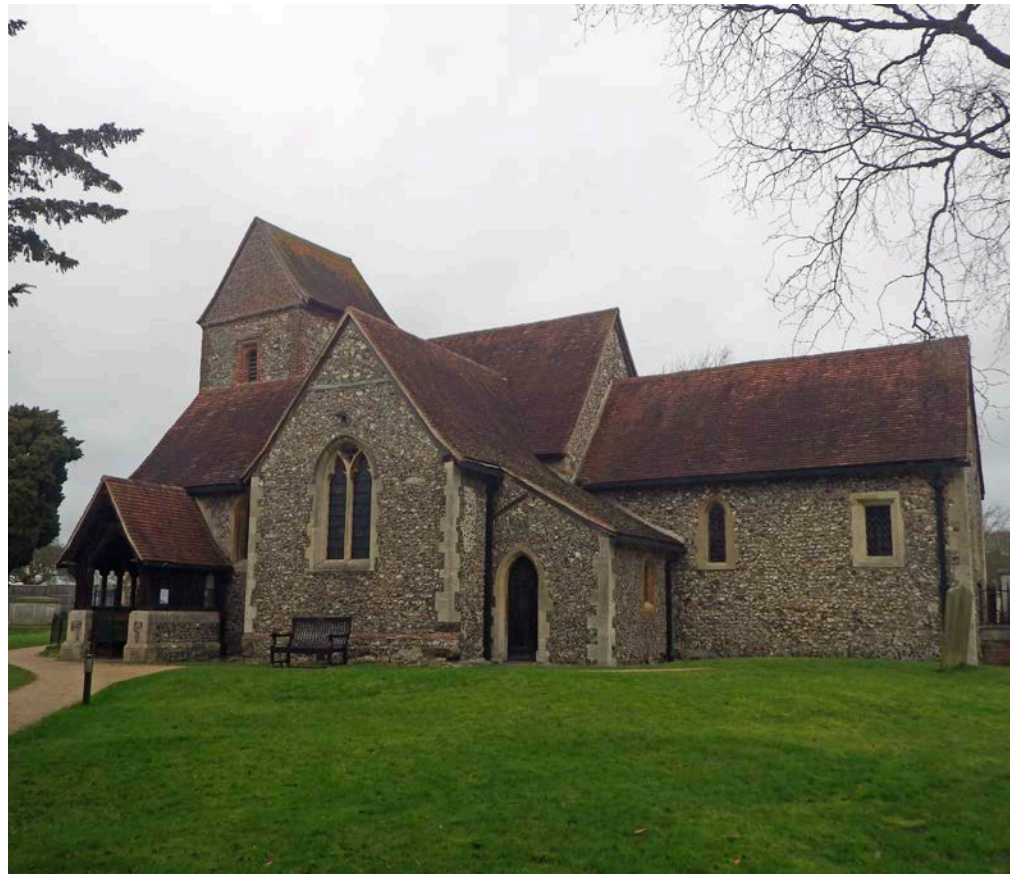
Figure 26: Church of the Holy Cross, Sarratt. Hertfordshire Puddingstone with Quarry Flint and Totternhoe Stone dressings.
