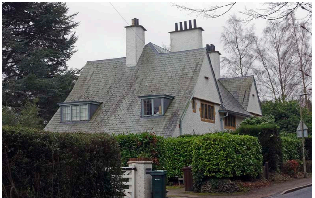
Figure 60: The Orchard, Shire Lane, Chorleywood. Roughcast brick with limestone (probably Bath Stone) dressings and a Cumberland Slate roof.
