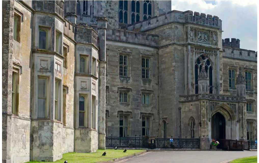
Figure 15: Ashridge House, near Berkhamsted. Totternhoe Stone ashlar, with Portland Stone and Ancaster Stone repairs.
