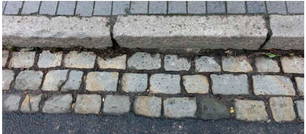
Figure 31: St Michael's Street, St Albans. Sarsen stone and granodiorite kerbing.
