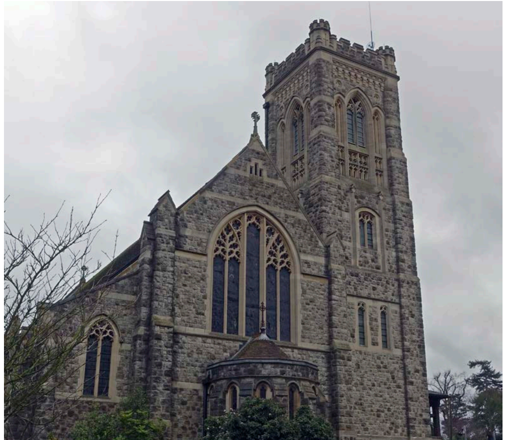
Figure 54: Church of St Peter, Bushey. Kentish Ragstone with Middle Jurassic limestone quoins and dressings.
