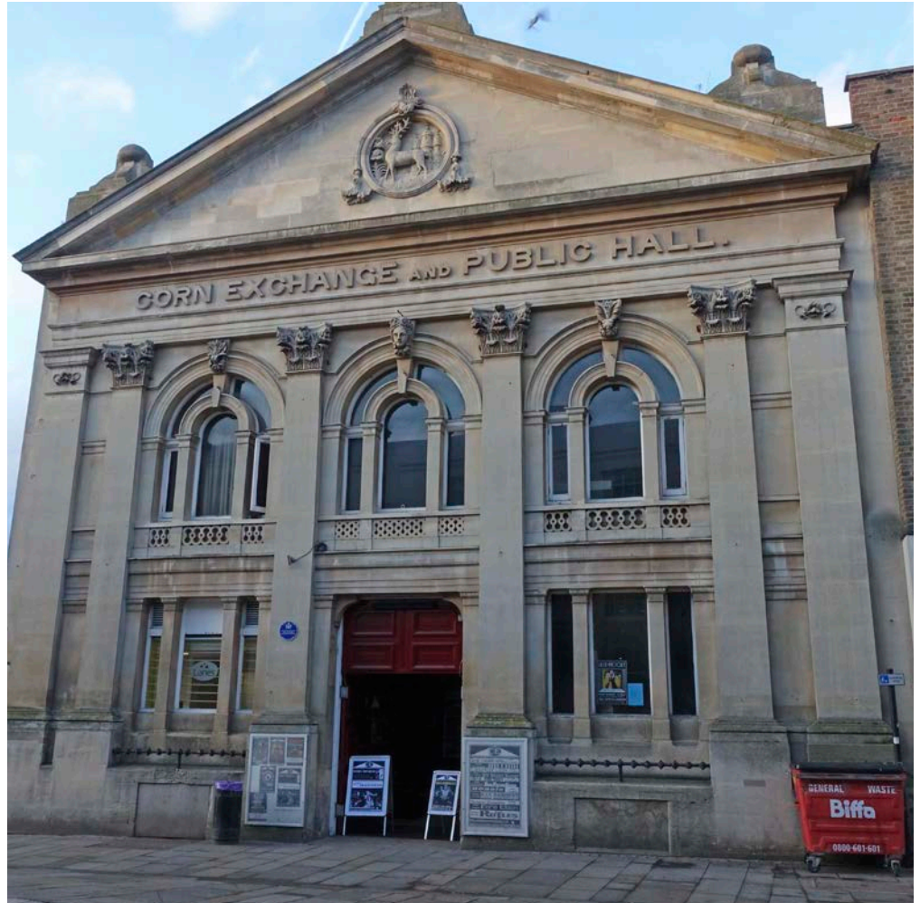
Figure 51: Corn Exchange and Public Hall, Fore Street, Hertford. Bath Stone ashlar.
