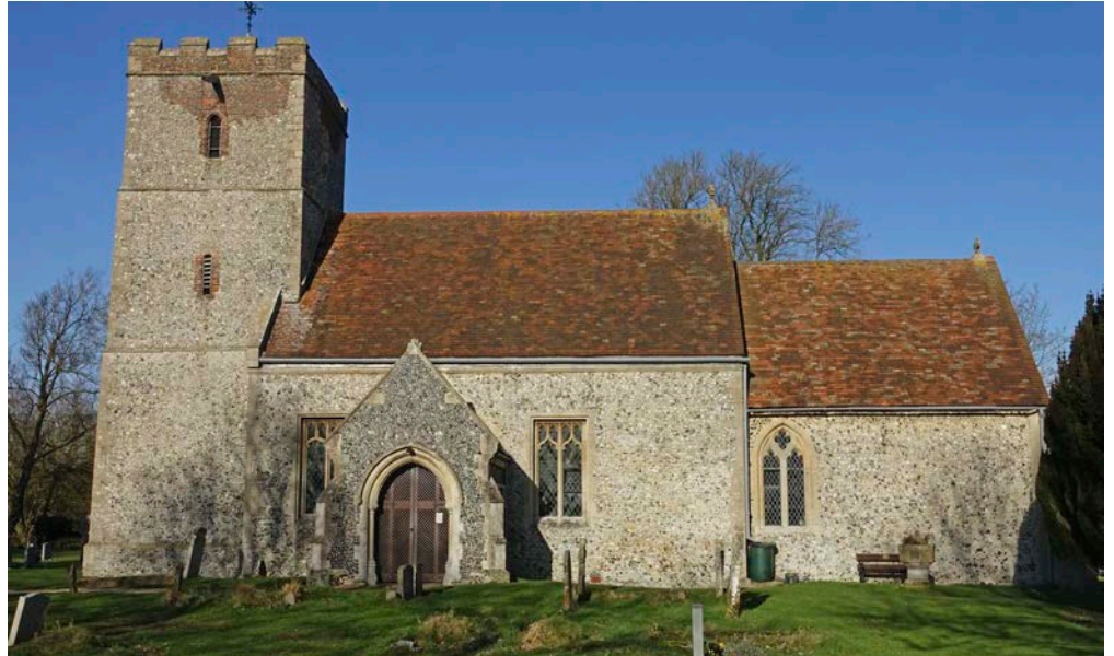
Figure 49: Church of St Mary, Reed. Quarry Flint with Quaternary Flint nodules, chalk clunch and Barnack Stone dressings.
