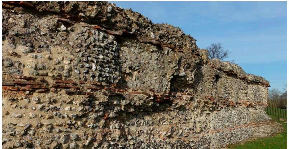
Figure 9: City wall, St Albans. Quaternary flint nodules and Roman tiles, with occasional glacial pebbles and cobbles.
