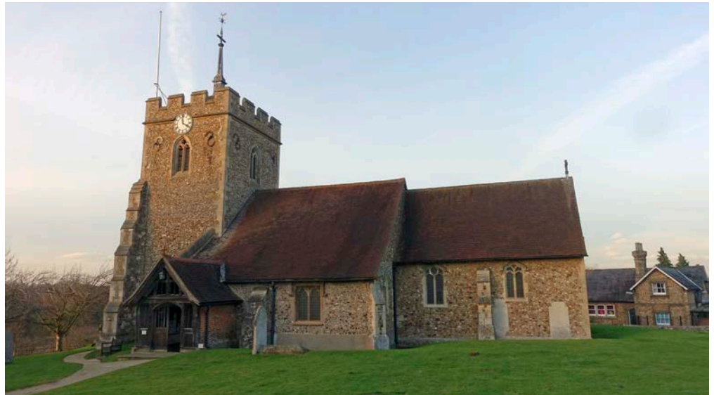
Figure 36: Church of St Ippolyts, St Ippolyts. Tufa, Quaternary Flint and Hitchin Carstone, with occasional glacial pebbles and cobbles and isolated blocks of Hertfordshire Puddingstone and False Puddingstone.
