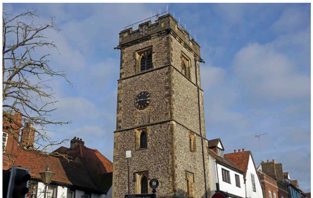
Figure 41: The Clock Tower, St Albans. Carboniferous sandstone and local flint.
