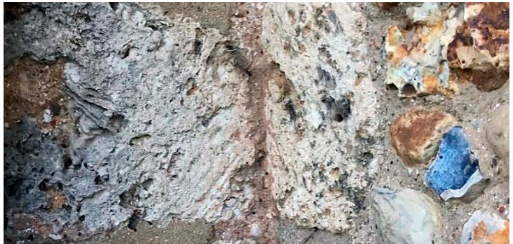
Figure 37: Church of St Ippolyts, St Ippolyts. Tufa with Quaternary Flint pebbles.
