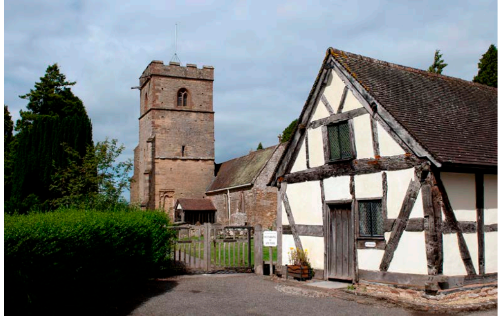
Figure 1: Timber framed building, Colwall. Stone sole plate.
