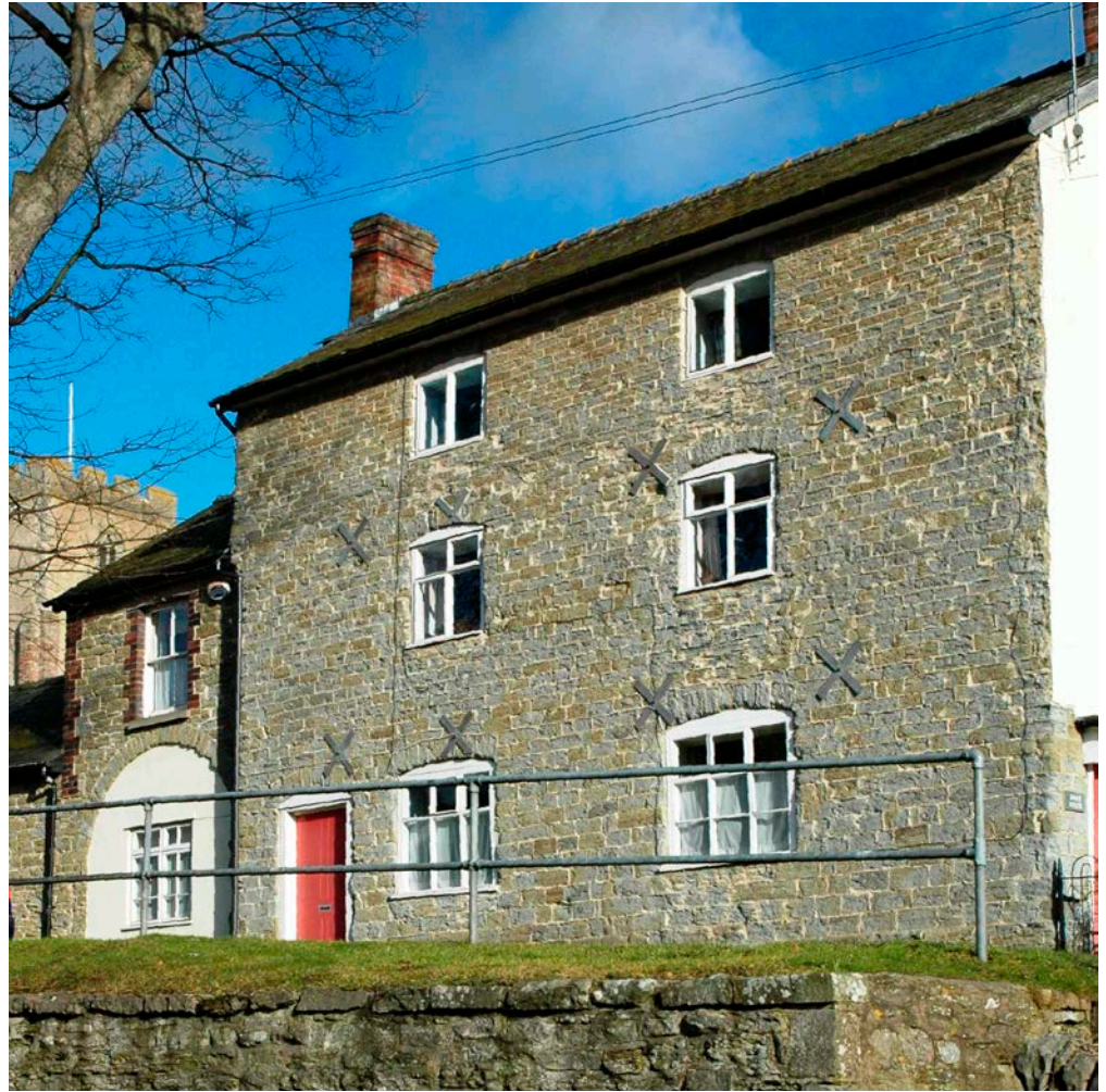
Figure 16: Bank House, High Street, Leintwardine. Upper Ludlow Shale stone.
