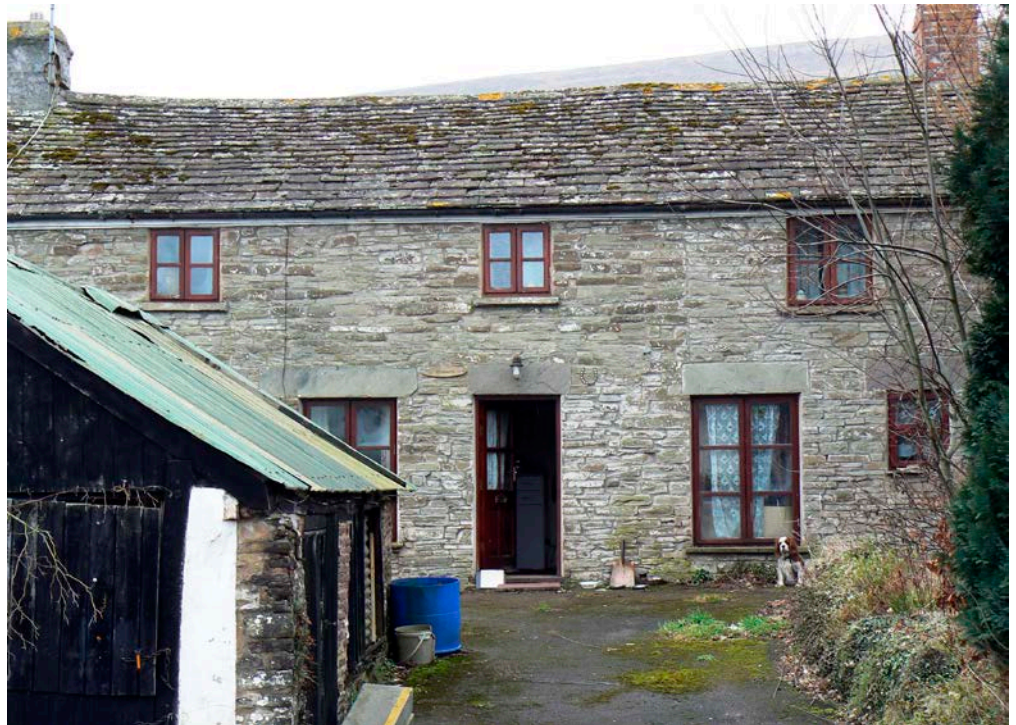
Figure 30: Flagstone roofs, Longtown. St Maughans Sandstone.
