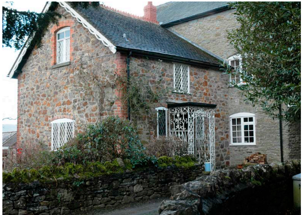
Figure 3: Buckton Mill, near Brampton Bryan. Upper Ludlow Shale and Broomie Hill Stone.
