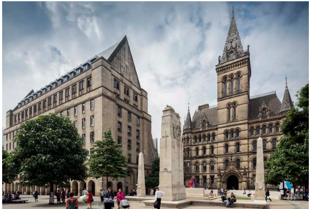
Figure 18: Manchester town hall (Gaisby Rock, right), the town hall extension (Darley Dale Stone, left) and the Cenotaph (White Portland Stone).
