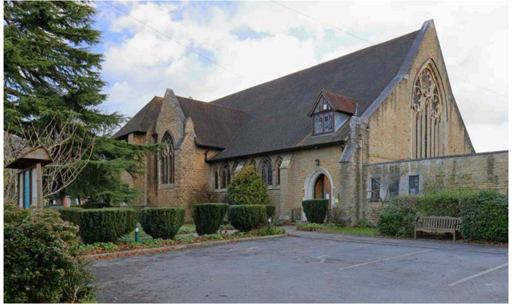
Figure 43: Church of St John, Belmont. Bargate Stone, with Ketton Stone (and possibly Bath Stone) dressings.
