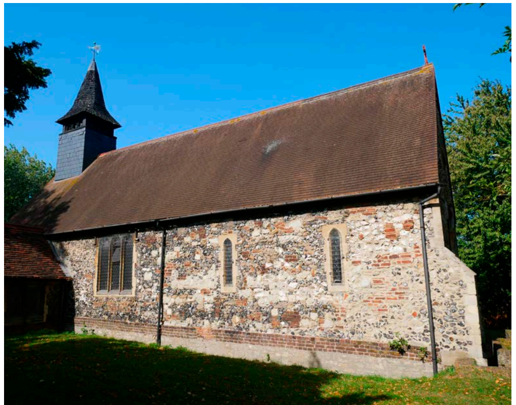
Figure 18: Greek Orthodox Church of Christ the Saviour, East Wickham. Knapped Quarry and Quaternary Flint, chalk, Cretaceous sandstone and brick.
