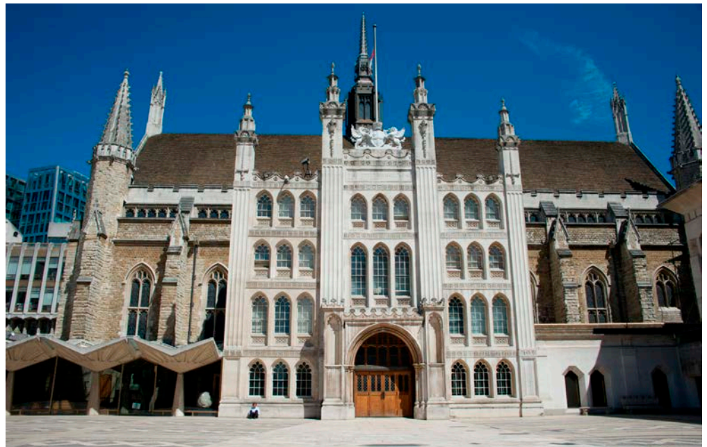
Figure 4: Guildhall, City of London. Kentish Ragstone and Portland Stone, with Collyweston Stone slate roof.
