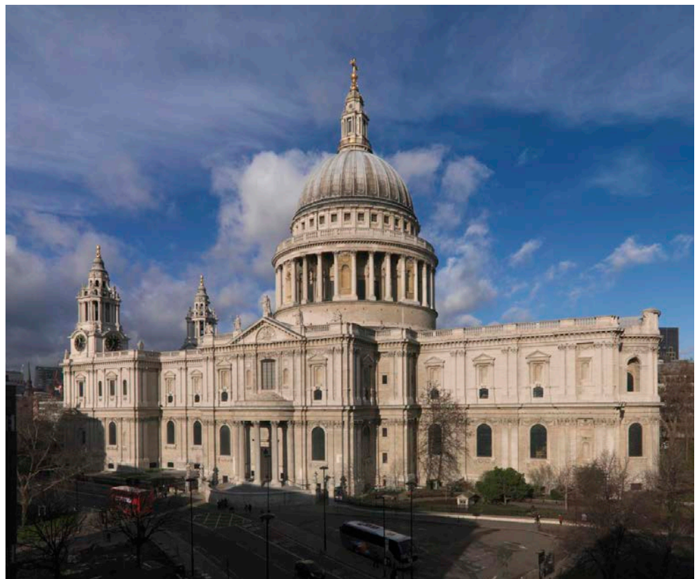
Figure 39: St Paul's Cathedral, City of London. Portland Stone including Jordans Basebed variety and some Weldon Stone.
