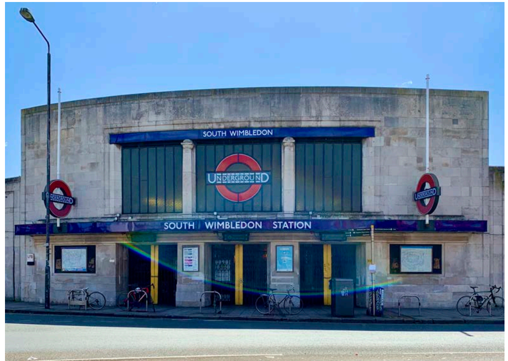
Figure 15: London Underground Station, South Wimbledon. Portland Stone cladding.
