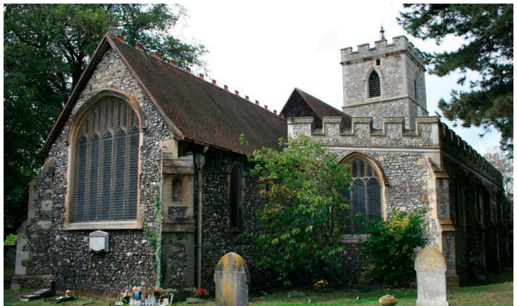
Figure 44: Church of St Mary the Virgin, Hayes. Quaternary Flint with Reigate Stone dressings.
