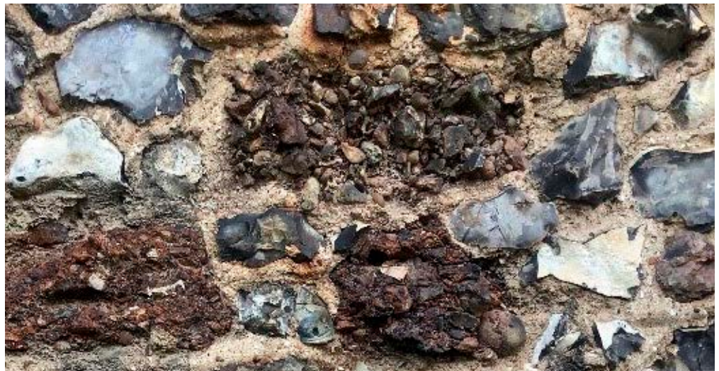
Figure 22: Church of SS Peter and Paul, Harlington. Hertfordshire Puddingstone, Conglomeratic Ironstone and Quaternary Flint.
