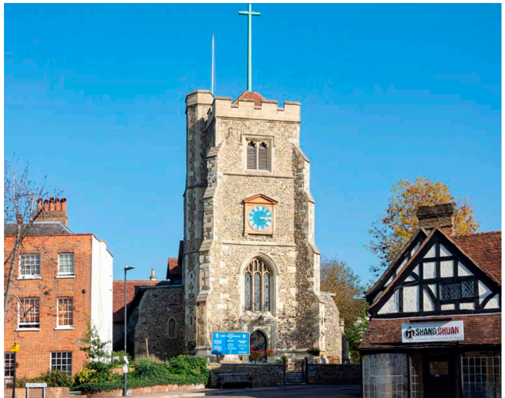
Figure 10: St John the Baptist Church, Pinner. Hertfordshire Puddingstone with flint and ironstone quoins.
