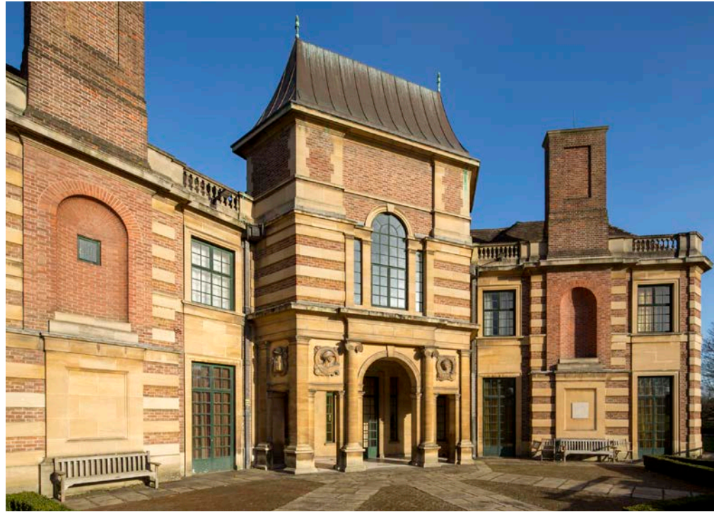
Figure 13: Eltham Palace, Eltham. Red brick and Clipsham Stone dressings.
