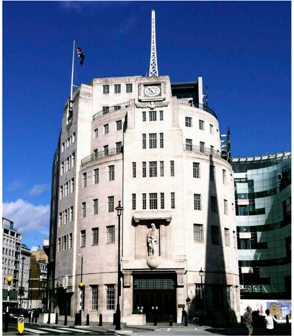
Figure 40: BBC Broadcasting House, Portland Place. Portland Stone and Bowers Roach variety.
