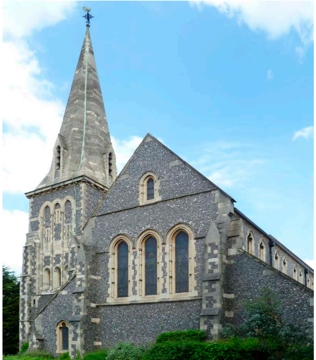
Figure 29: Church of All Saints, Oakleigh Park. Quaternary Flint, Ancaster Stone and Bath Stone.
