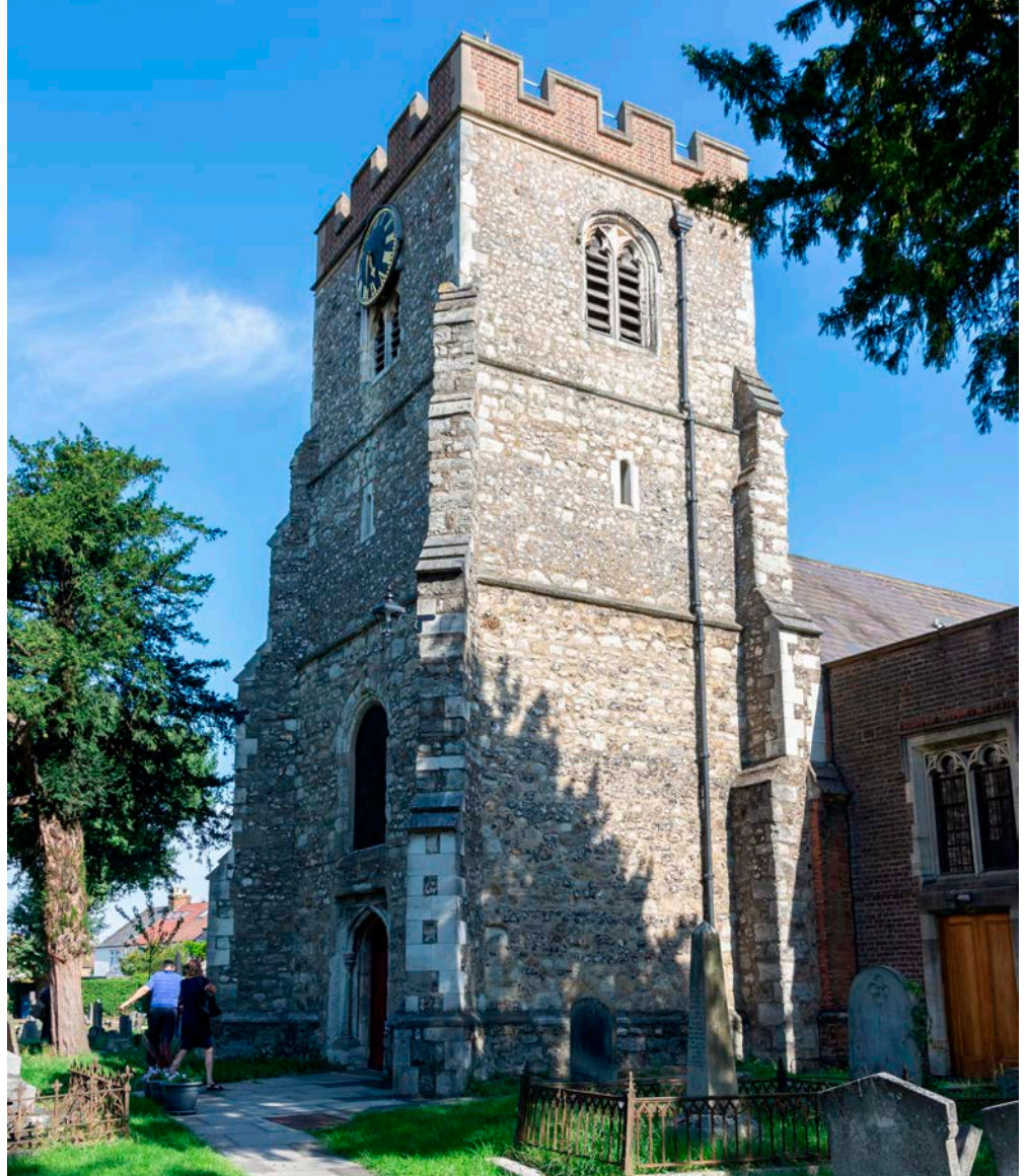
Figure 21: Church of St Margaret of Antioch, Edgware. Hertfordshire Puddingstone and other stones.
