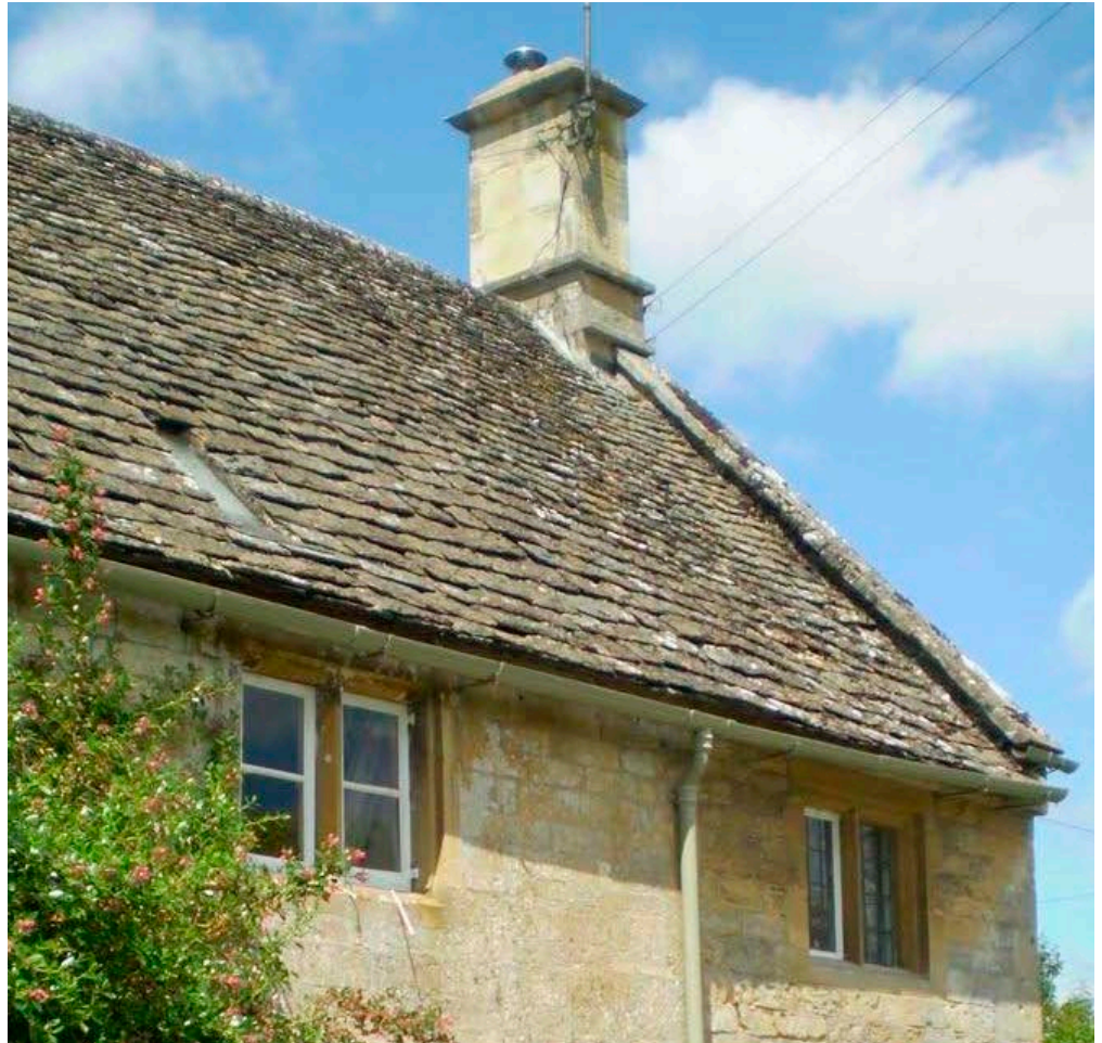
Figure 16: Cottage roof, Taynton. Cotswold Stone slate.
