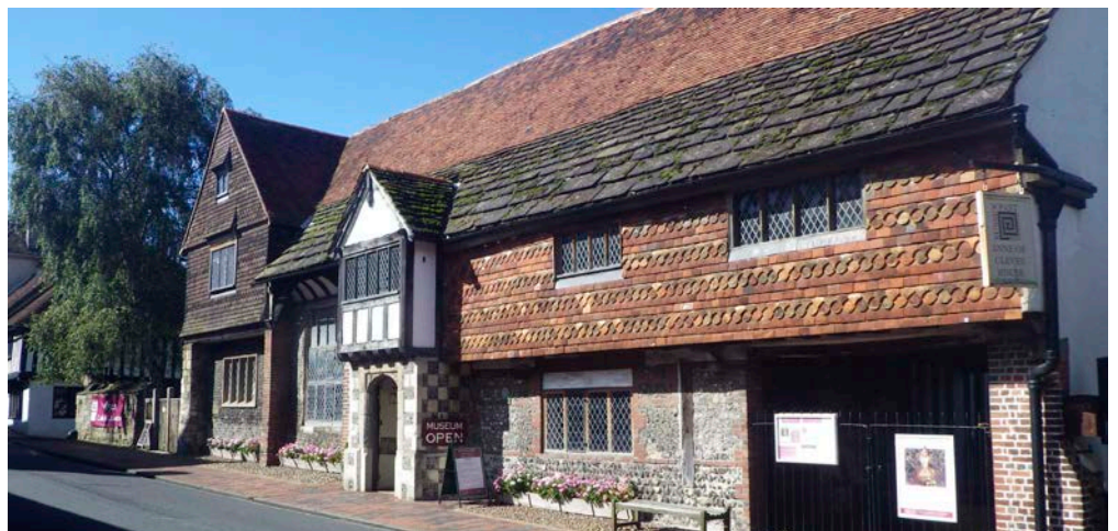
Figure 12: Anne of Cleves House, Lewes. Horsham Stone slate roof eaves.
