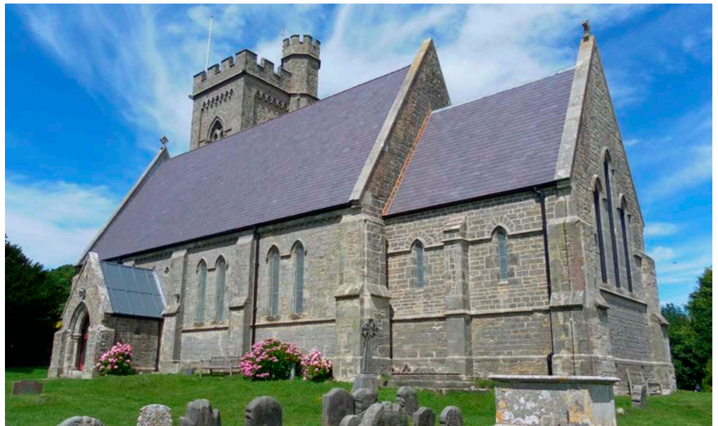
Figure 6: St Andrew's Church, Fairlight. Cliff End Sandstone.
