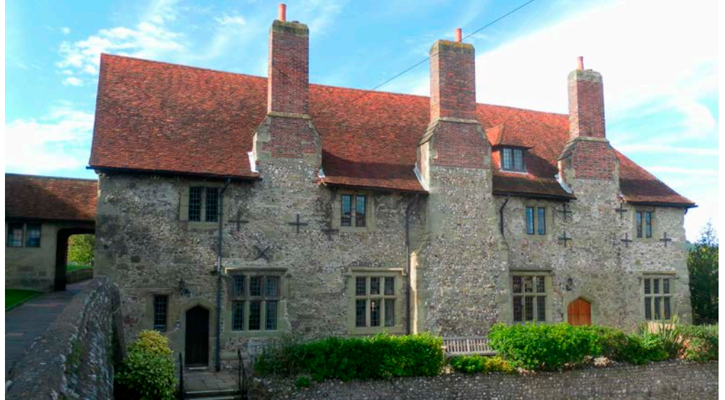
Figure 15: Parsonage, Eastbourne. Flint nodules and pebbles, with occasional blocks of ironstone and quoins of Eastbourne Sandstone.
