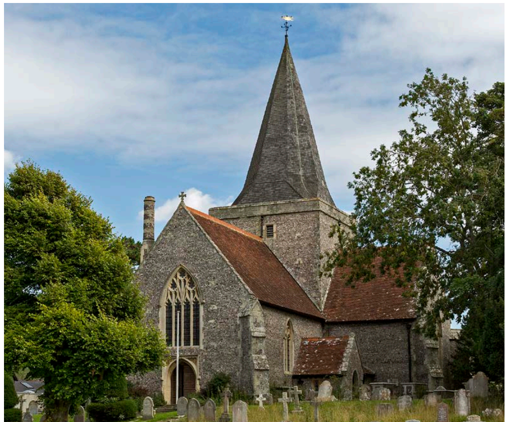
Figure 17: St Andrew's Church, Alfriston. Knapped Quarry Flint and Downland Field Flint.
