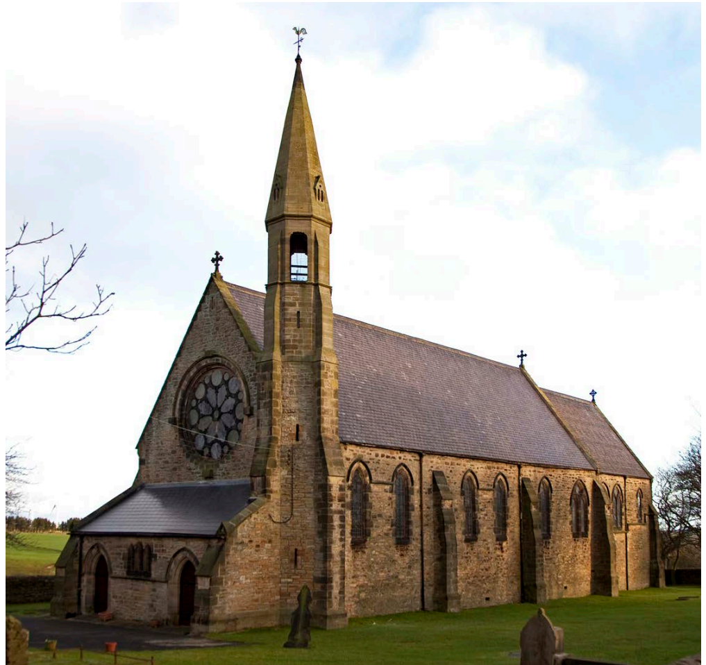
Figure 9: Church of St Philip and St James, Tow Law. Lower Coal Measures Sandstone.
