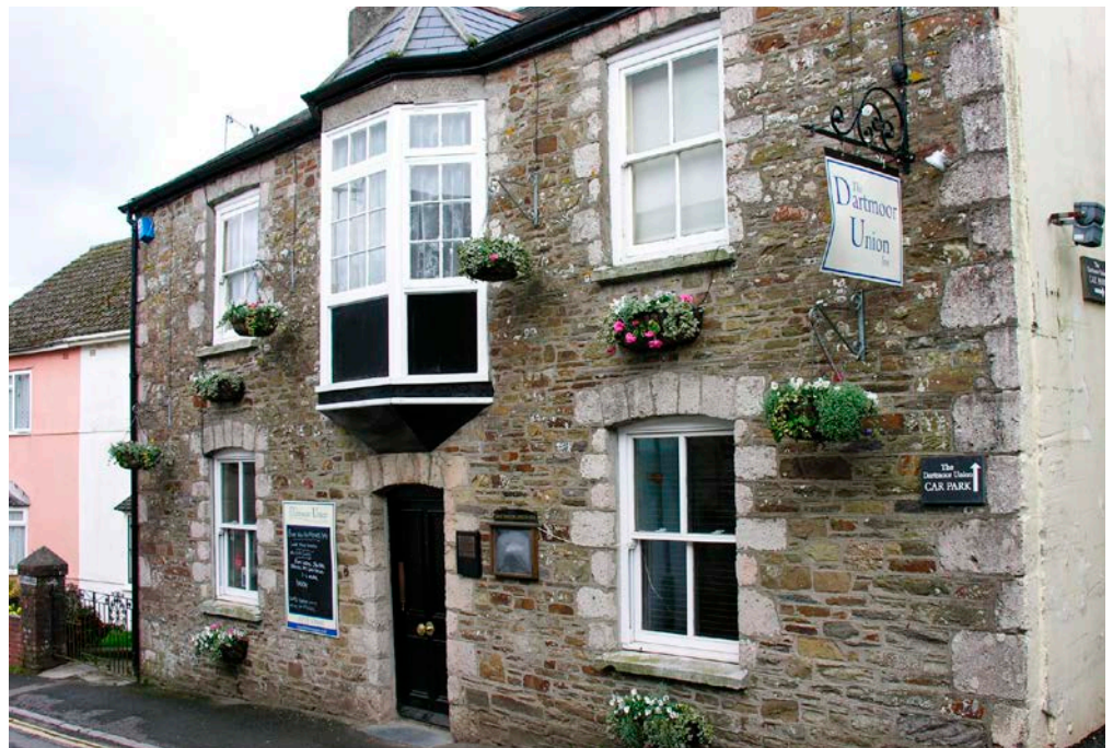
Figure 3: Public house, Holbeton. Meadfoot Group stone.
