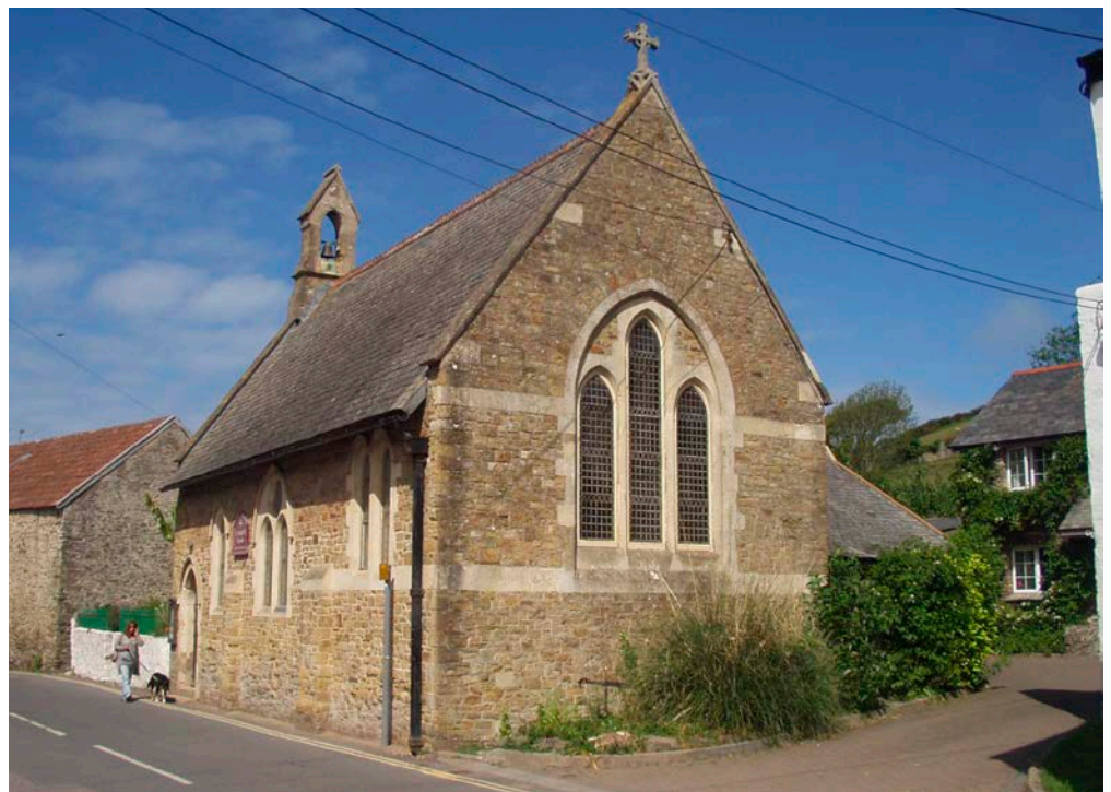
Figure 9: St Mary's Church, Croyde. Baggy Sandstone with Bath Limestone dressings.
