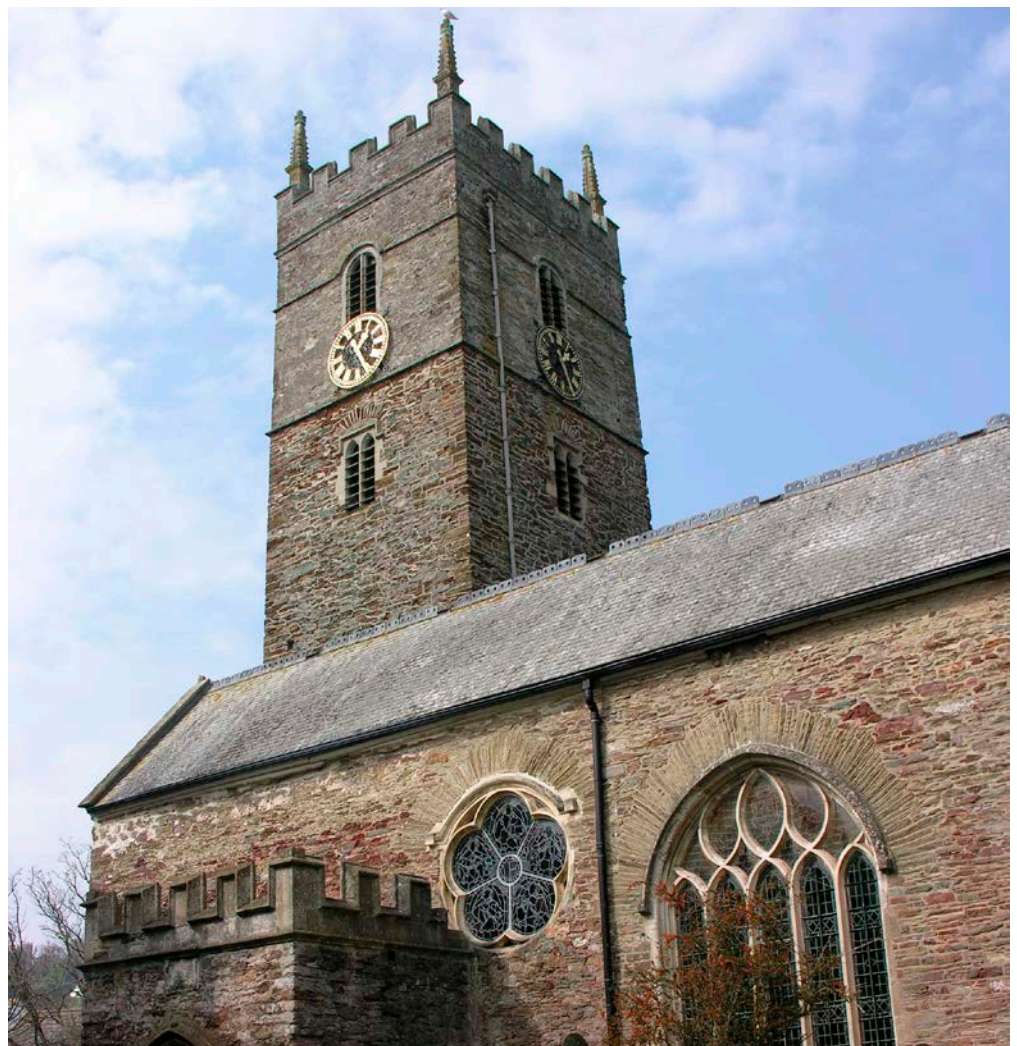
Figure 2: St Saviour's Church, Dartmouth. Local rubblestone from the Whitsand Bay Formation, with Bath Stone and Salcombe Stone dressings.
