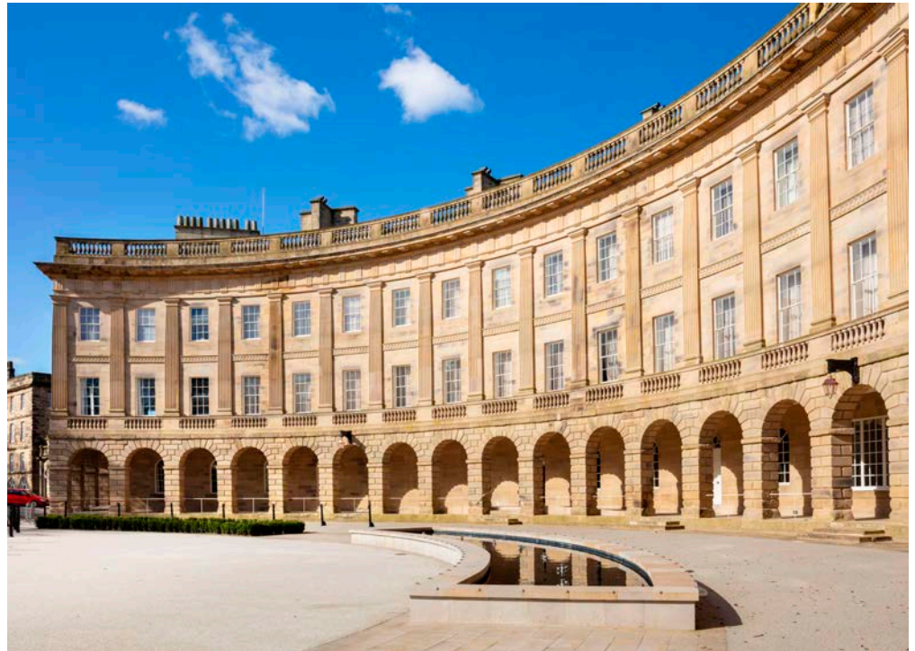
Figure 10: The Crescent, Buxton. Corbar Grit.
