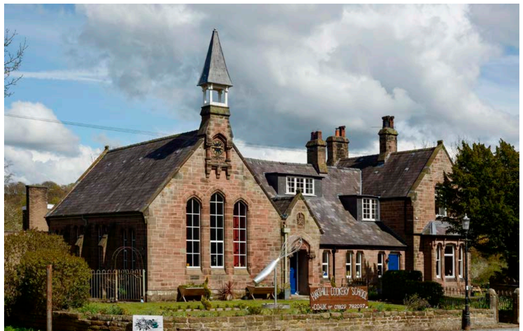
Figure 12: Former school, Harthill. Delamere Sandstone.
