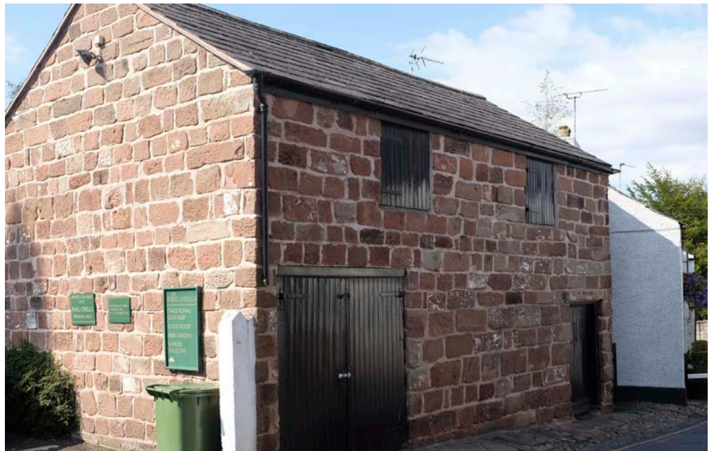
Figure 14: Outbuildings on Bellemonte Road, Frodsham. Frodsham Sandstone.
