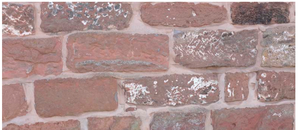
Figure 15: Outbuildings on Bellemonte Road, Frodsham. Frodsham Sandstone.
