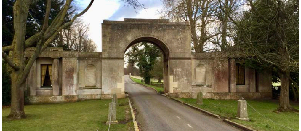
Figure 68: Entrance gateway, Tyringham Hall, near Newport Pagnell. Roman cement render and Weldon Stone dressings.
