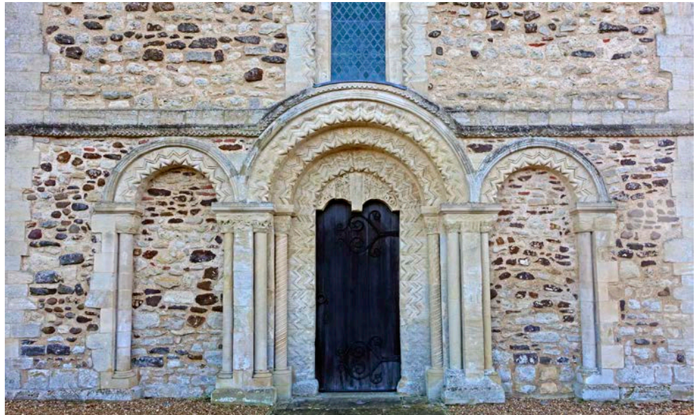
Figure 57: St Michael and All Angels Church, Stewkley. Portland Limestone (Buckinghamshire type) and glacial pebbles and cobbles.
