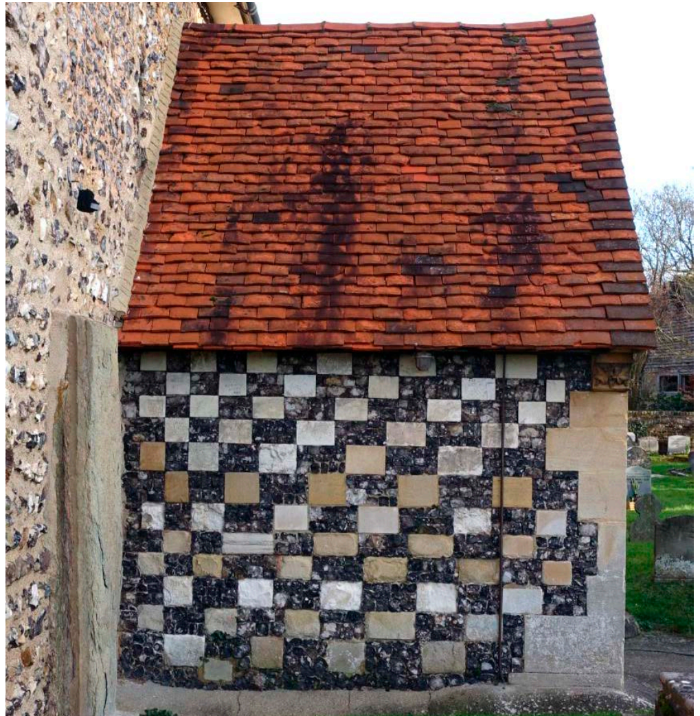
Figure 35: St Mary's Church, Burnham. Quarry Flint and Jurassic limestone, including Portland Limestone (Buckinghamshire type), chequerwork.
