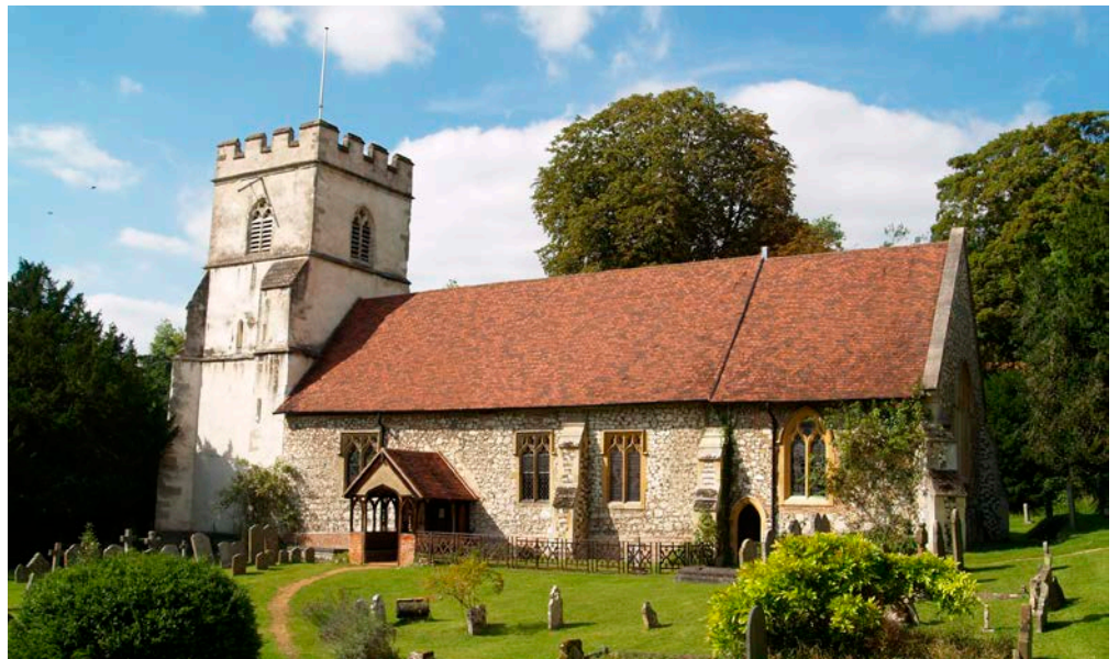
Figure 40: Church of St Peter and St Paul, Medmenham. Quarry Flint and chalk block with Bath Stone dressings.
