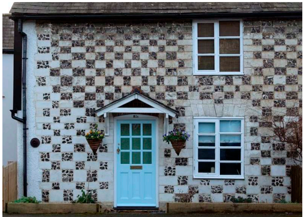
Figure 13: Cottage, Princes Risborough. Quarry Flint and chalk block chequerwork.
