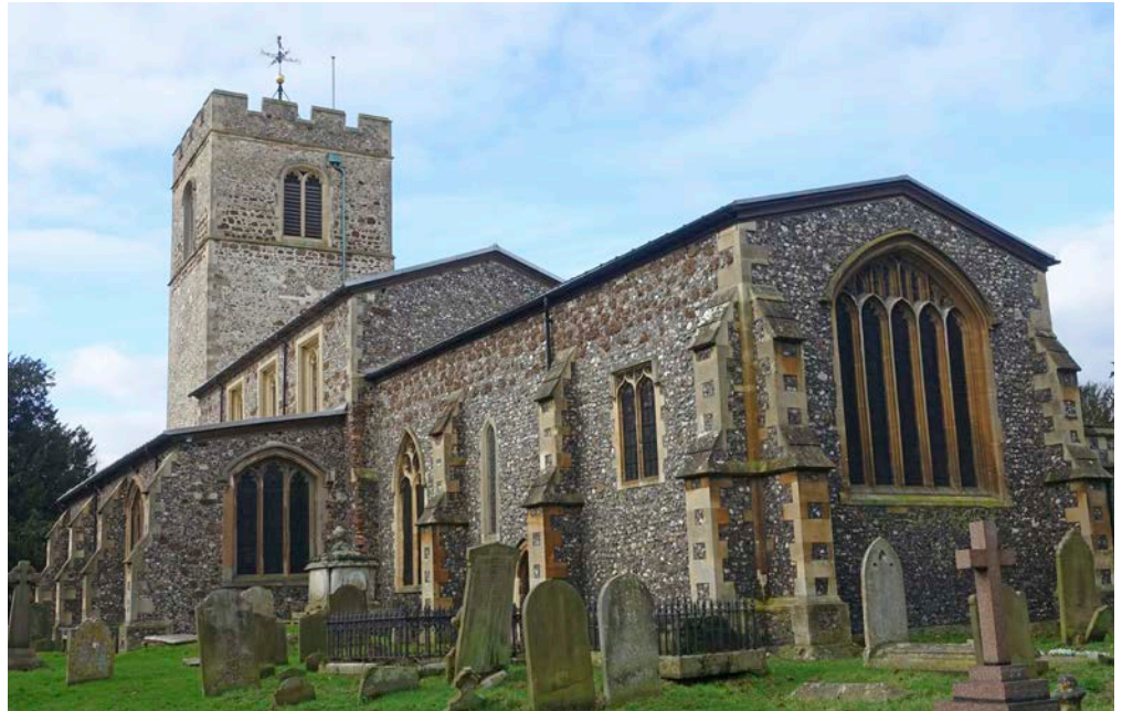
Figure 54: St Peter's Church, Iver. Quarry Flint with False Puddingstone, glacial pebbles and cobbles and Roman tiles.
