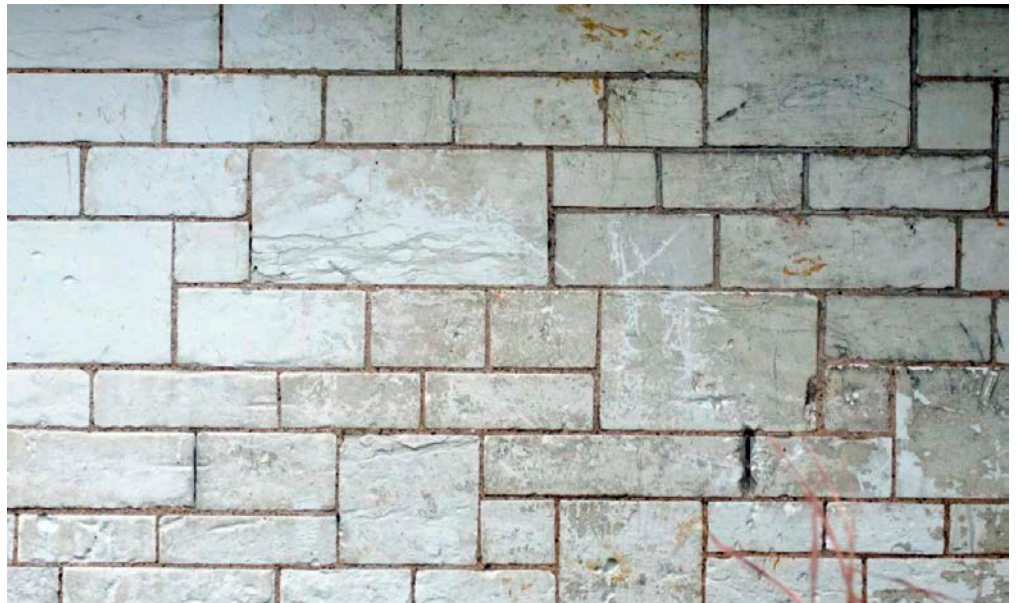
Figure 39: Cottages, Bockmer End, Medmenham. Chalk block ashlar.
