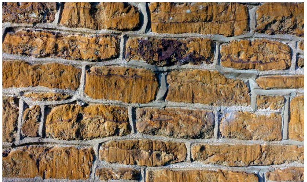
Figure 65: Church wall, Hoggeston. Northampton Ironstone.
