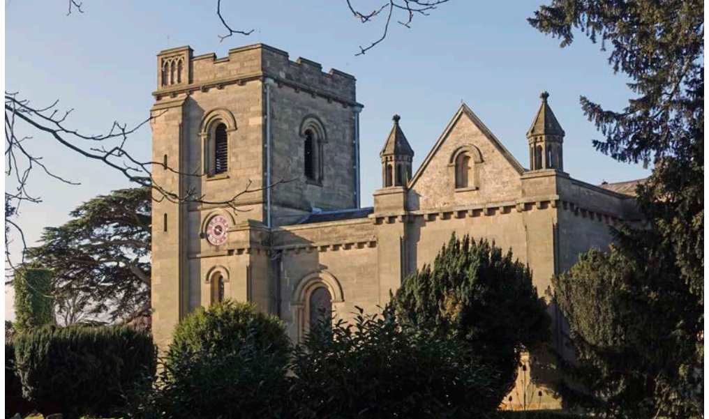
Figure 62: Church of the Holy Trinity, Wolverton. Attleborough Sandstone and Blisworth Limestone.
