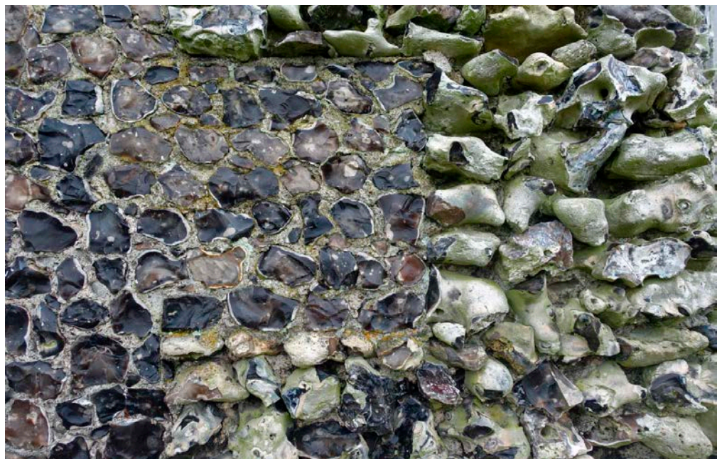
Figure 53: Dashwood Mausoleum, West Wycombe. Knapped Quarry Flint and Quaternary Flint contrasting with unworked Quaternary Flint nodules.
