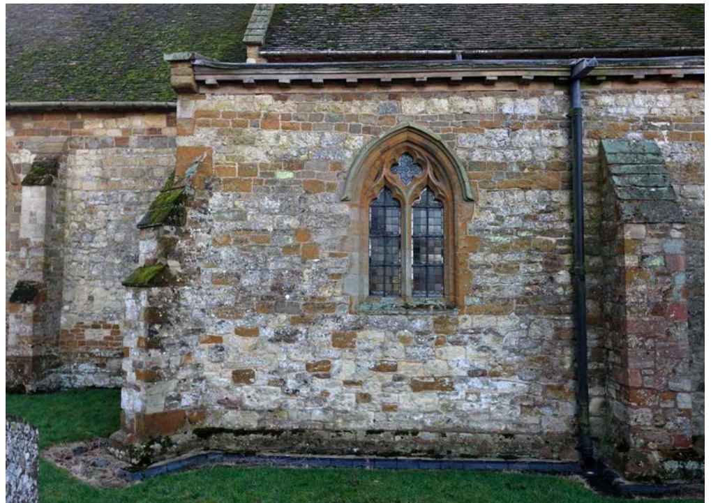
Figure 64: Church of the Holy Cross, Hoggeston. Northampton Ironstone and Portland Limestone.
