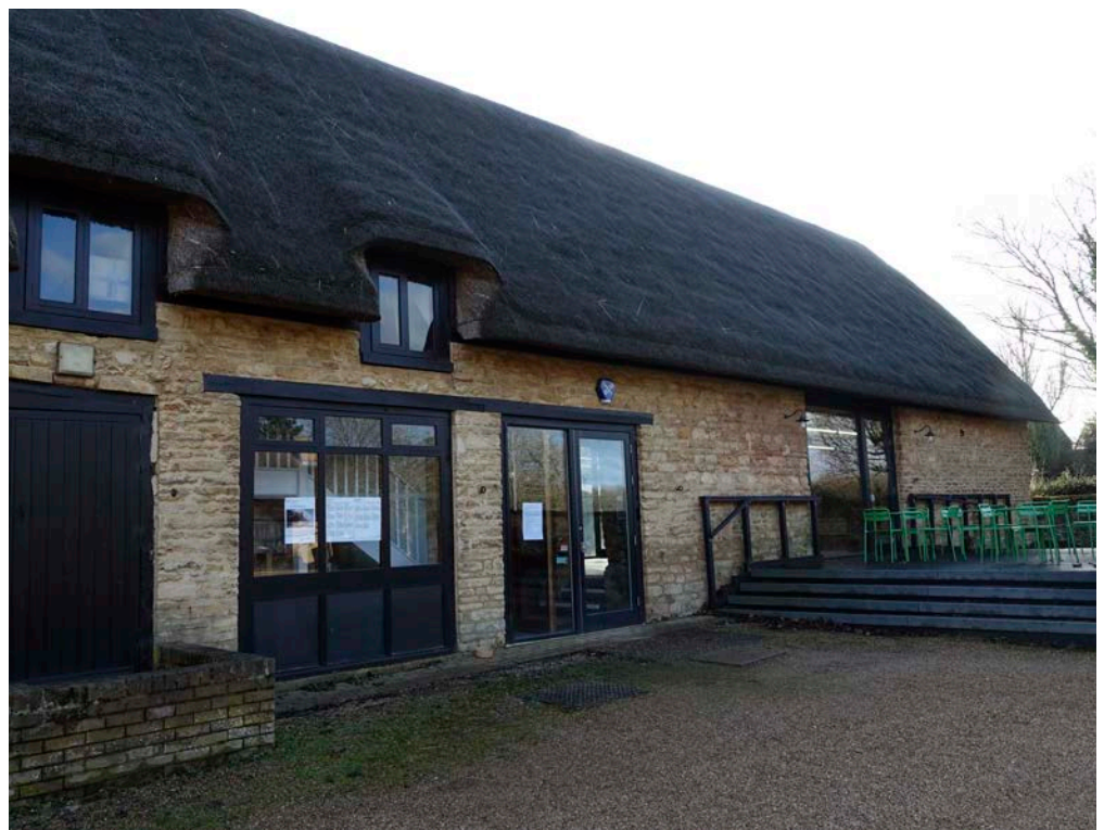
Figure 71: Milton Keynes Arts Centre, Great Linford. Blisworth Limestone and a pink Northamptonshire type limestone.
