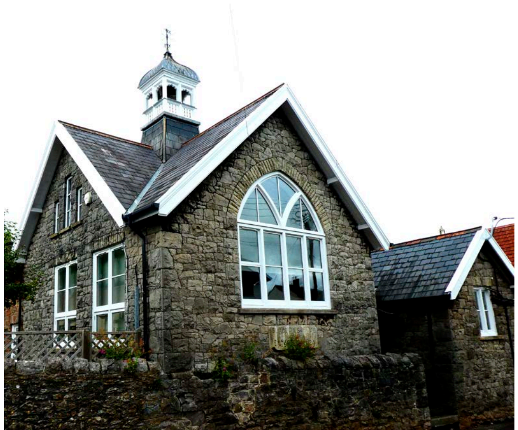
Figure 5: Blagdon Primary School, Blagdon. Lower Carboniferous Limestone.
