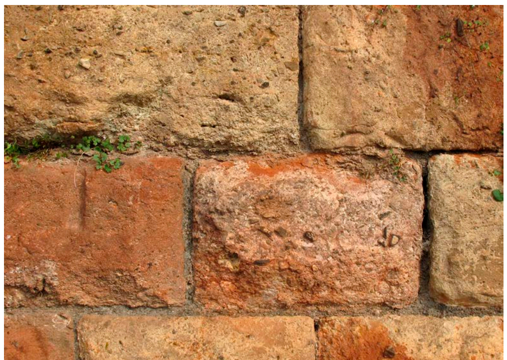
Figure 14: Walling, College Road, Clifton, Bristol. Deep red Dolomitic Conglomerate used with Carboniferous Limestone and Oolitic Limestone.
