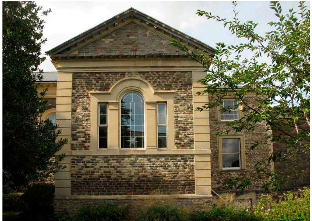
Figure 12: Lodge, St John's Road, Clifton, Bristol. Pennant Sandstone, some Lower Carboniferous Limestone, and Bath Stone quoins, ornament and window surrounds.
