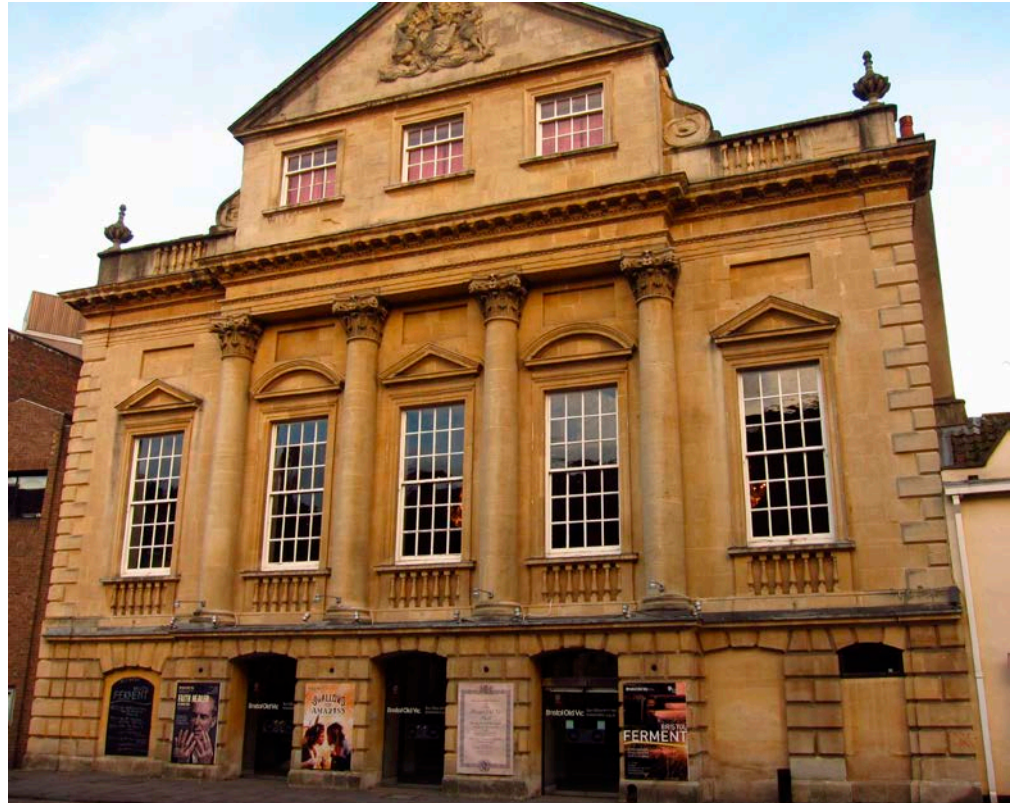
Figure 31: Bristol Old Vic Theatre, King Street, Bristol. Bath Stone.
