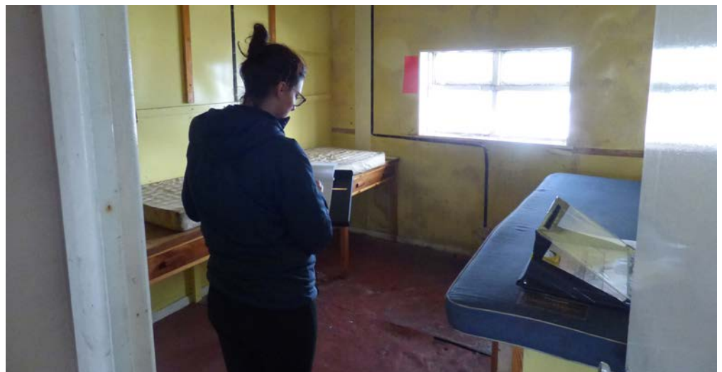
Figure 15: Undertaking a condition survey on site © Joanna Hull
