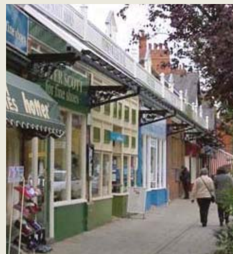
Image Shopfronts in Woodhall Spa restored as part of the East Lindsey HERS © East Lindsey District Council
