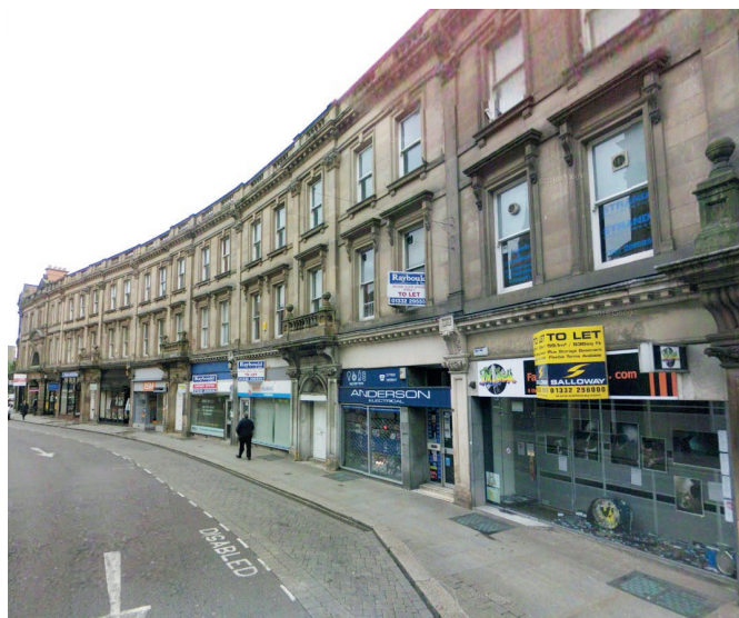
Images: 10 – 28 The Strand, Derby before and after multiple shop front repairs and reinstatement
