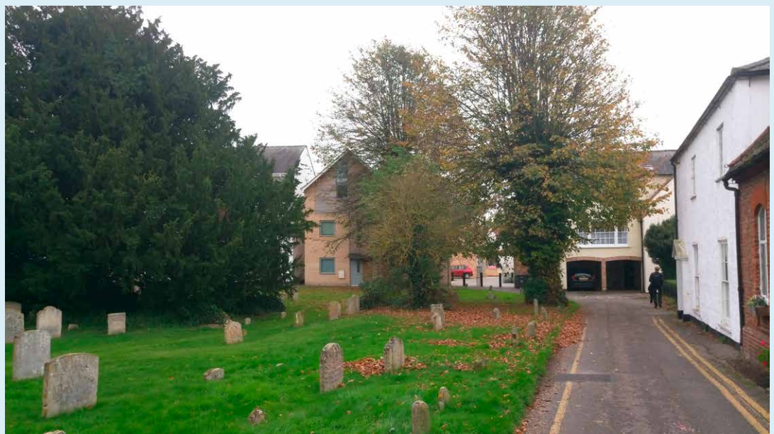
Image: The development responds sensitively to its location, melding with its surroundings facing into the churchyard. © Edward James
