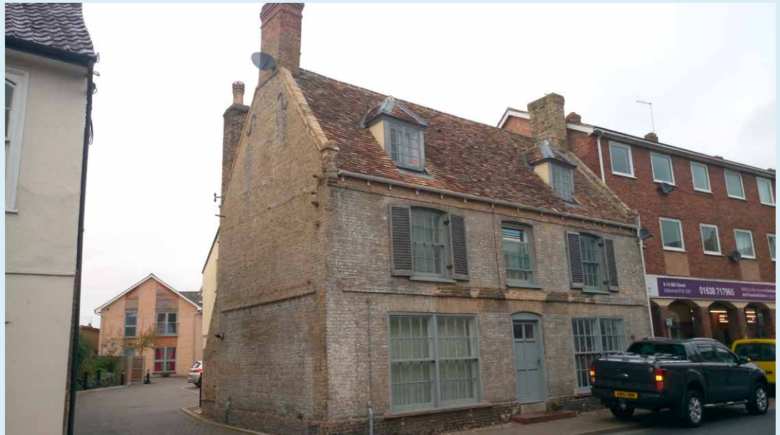
Image: The front, street facing elevation of 16 Mill Street. © Edward James
