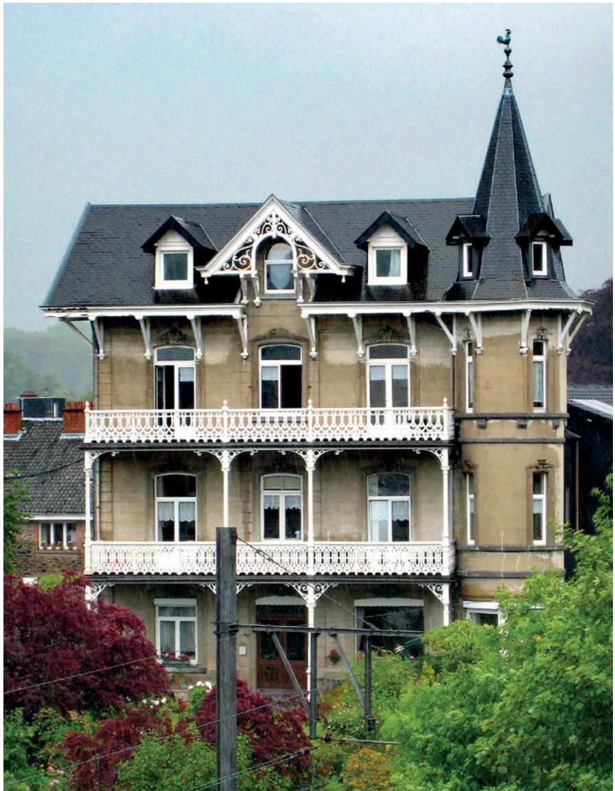
Traditional building features such as wide overhangs and hood mouldings were designed to keep water from entering the wall at weak points, keeping the walls dry and allowing them to resist driving rain.
