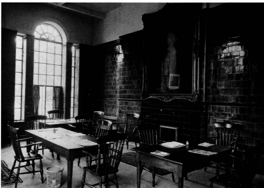
Fig. 11 Ada Lewis Women's Lodging House, Daily Mirror photograph of sitting room c.1913. The portrait of the patron, Ada Lewis, was hung on the glazed tiled walls. This room has integral fireplaces which help create a grand and comfortable space amongst the other, practical common rooms.
