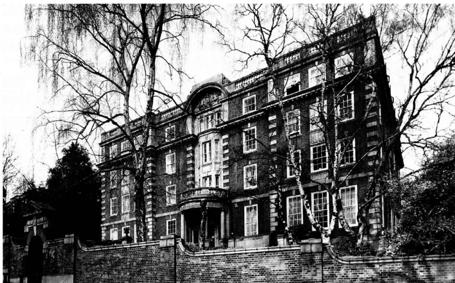
Fig. 13 Furnival House, Cholmeley Avenue, Highgate. Listed Grade II. [Geoff Brandwood].
