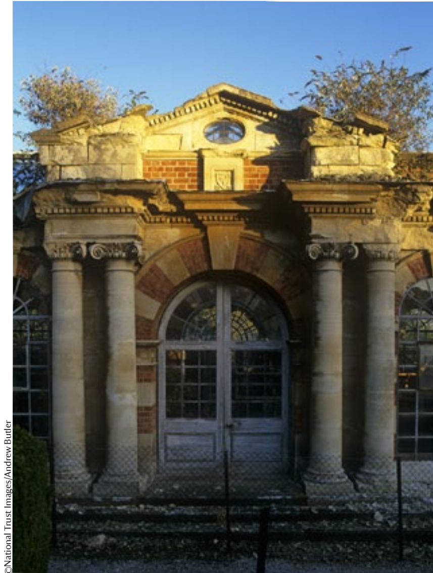
Above Detail of the Orangery door showing the decaying stonework
