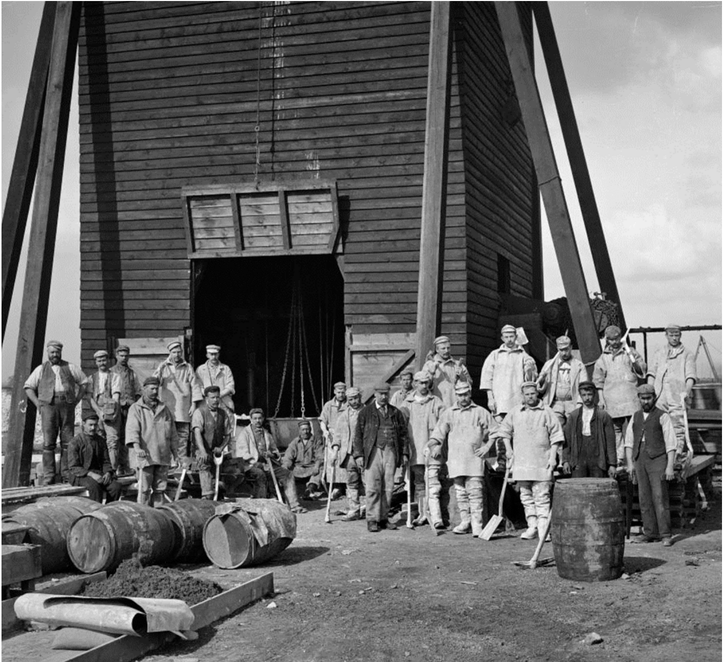
East London Water Works, New Road, Barking, Greater London
